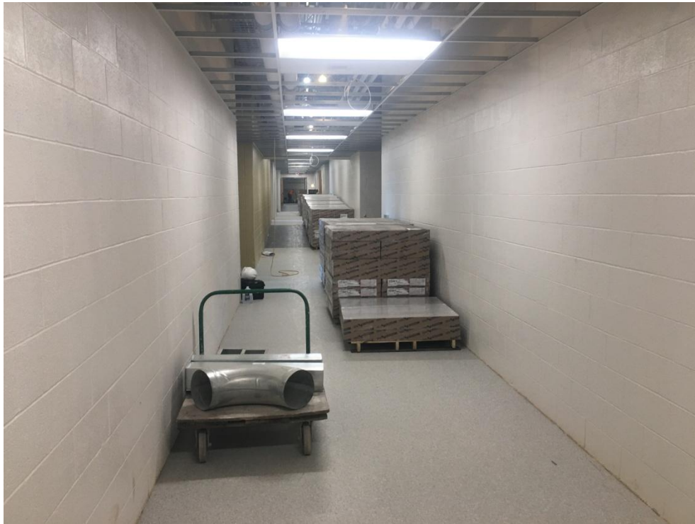
View of corridor in Classroom Addition with flooring and new lighting in place.
