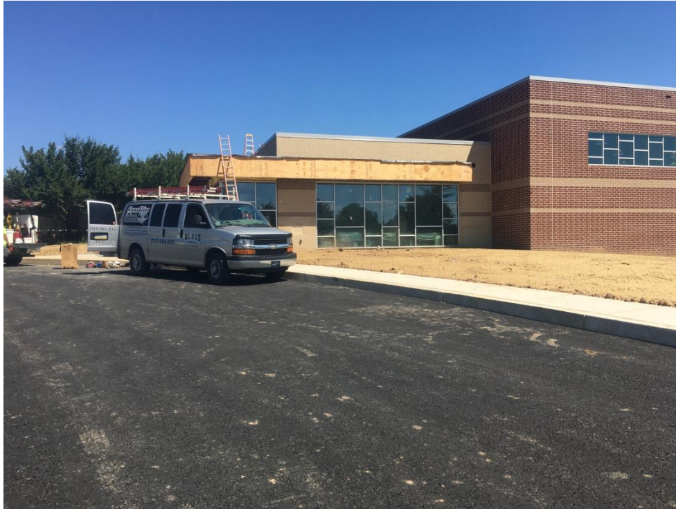
View of South side of exterior of Gym lobby entrance.
