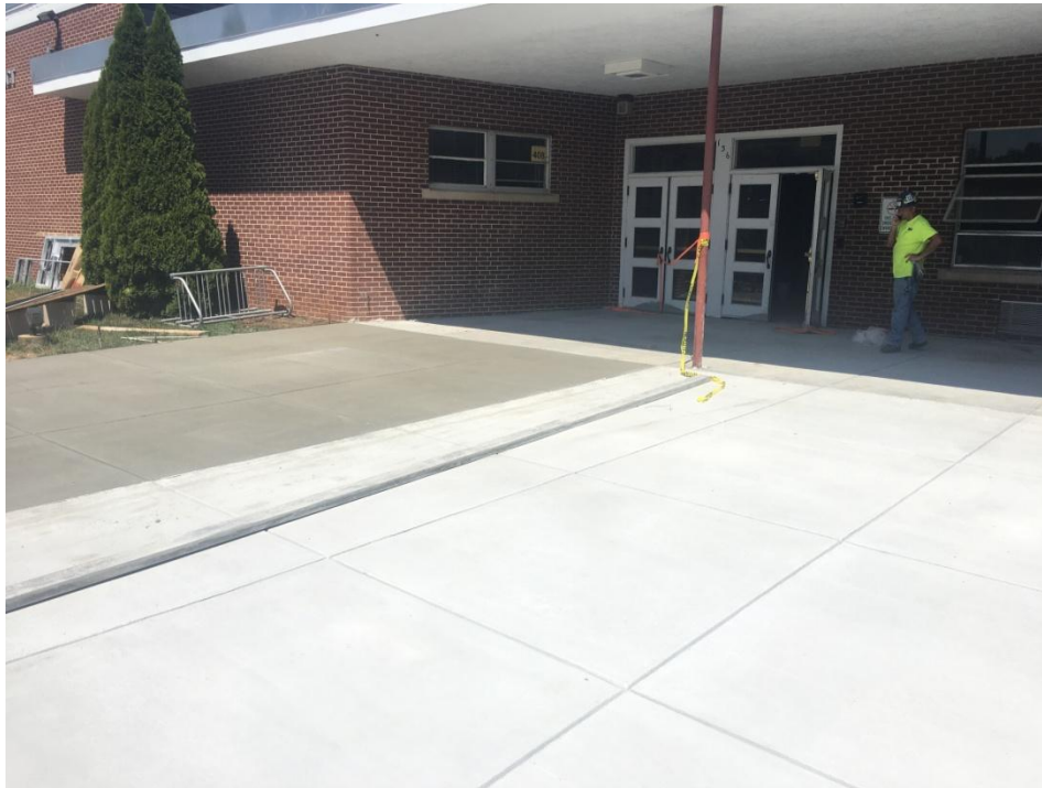
View of new concrete slab and walk at Front Entrance.
