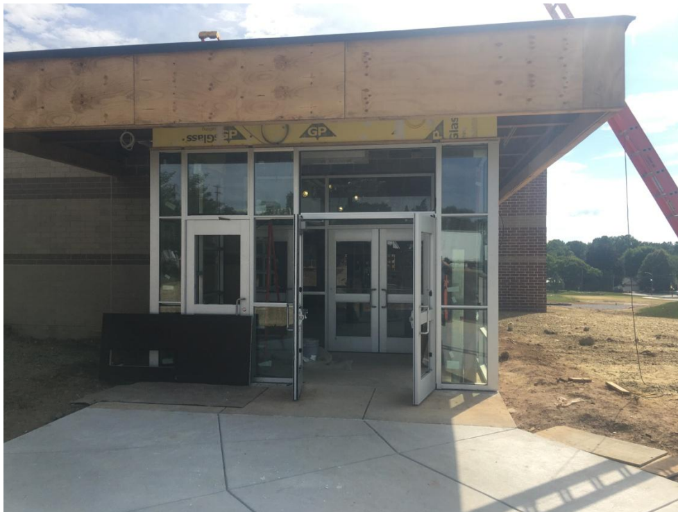
View of storefront entrance to new Gym.
