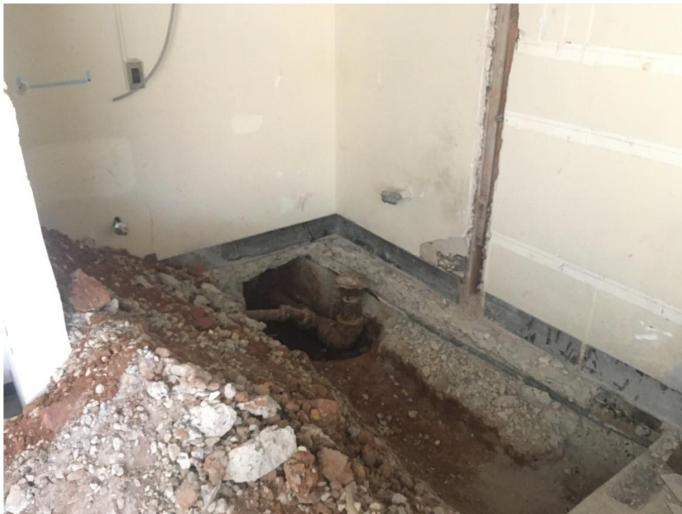
View of excavation for new bath in Life Skills room.
