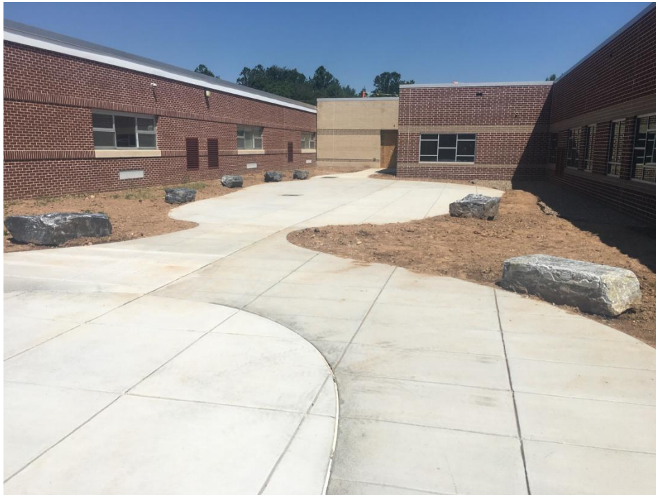
View of new Courtyard with stones in place.
