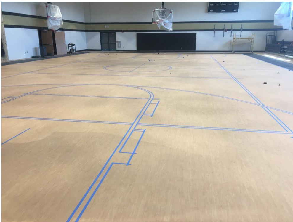
View of masking for line painting in new Gym.
