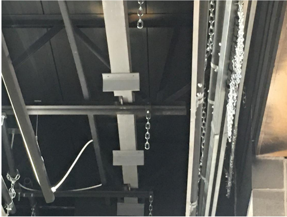
View of bottom of steel reinforcing for moveable partition on Gym Platform.
