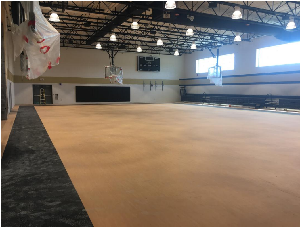
View of New Gym with flooring.
