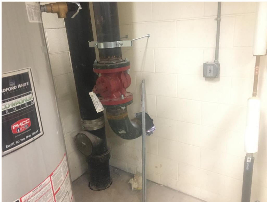
View of new gas connection.
