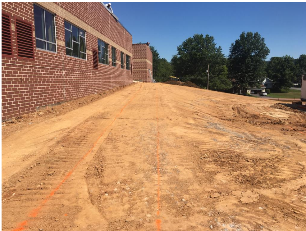
View of grading for ramp at rear of new Classroom Addition.
