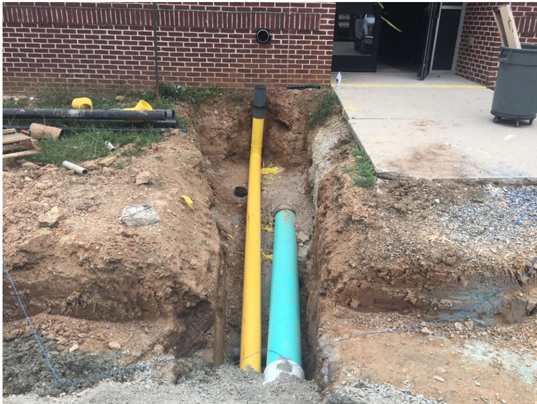
View of new gas line and repaired roof drain/storm sewer connection.
