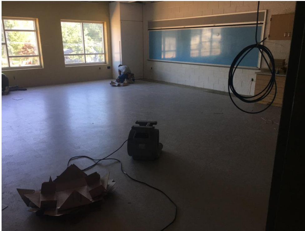
View of new classroom with flooring laid.
