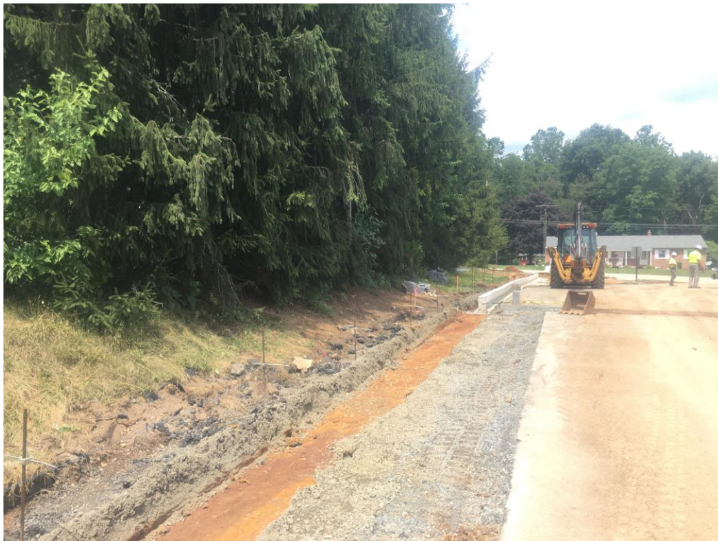
View of pine trees along Rear Parking Lot after trimming back.
