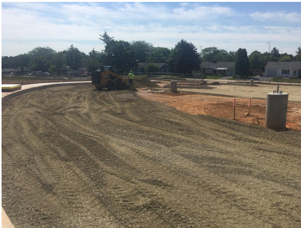
View of stone being spread on Front Parking Lot.
