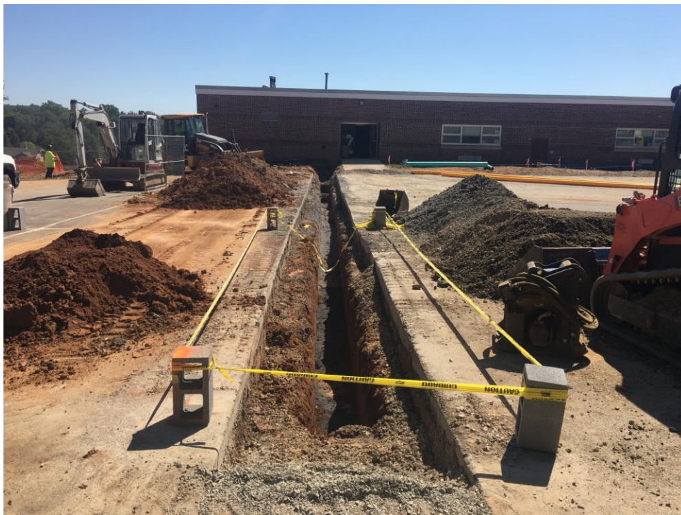
View of excavation for new gas line.
