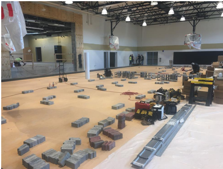
View of new Gym floor being laid. Note weights to keep it flat while gluing.
