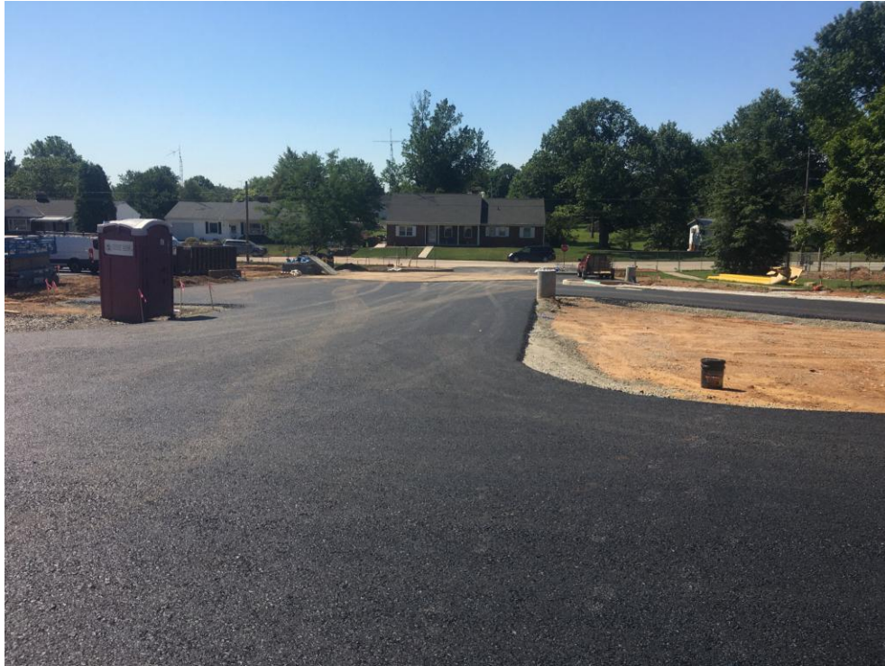
View of Front Parking lot after asphalt base was laid.
