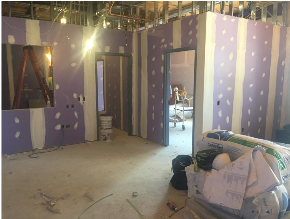
View of new Admin area.
