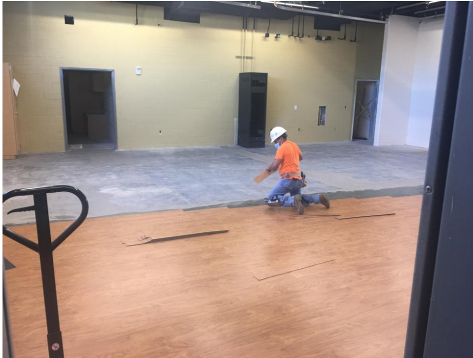
View of new floor being laid on the Platform/Music Classroom.
