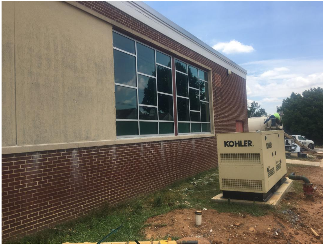
View of new Cafeteria windows.
