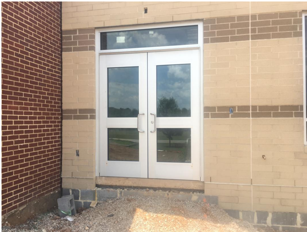
View of new doors at playground exit.
