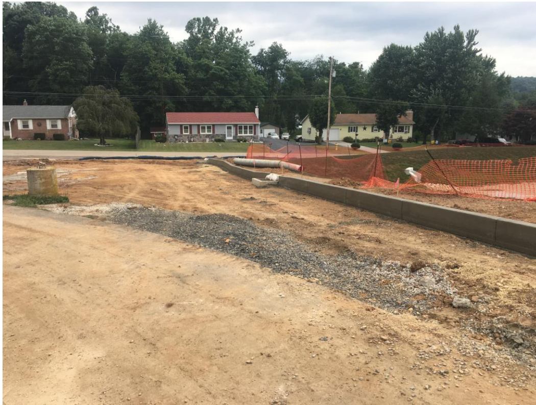
View of curb being poured at Rear Parking Lot.
