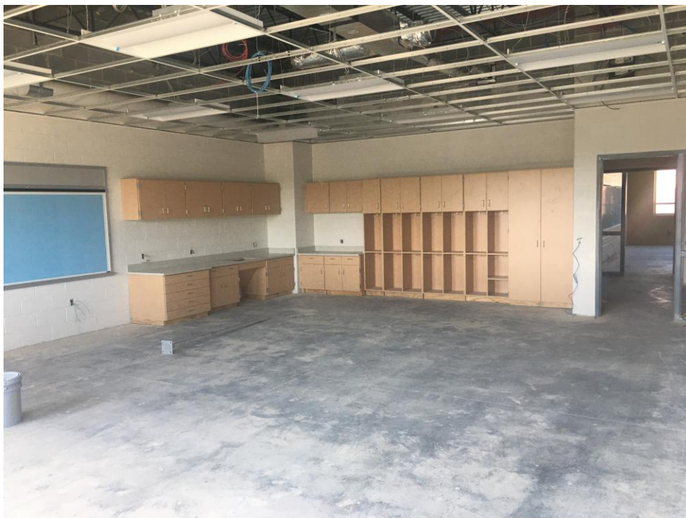
View of classroom in new wing.
