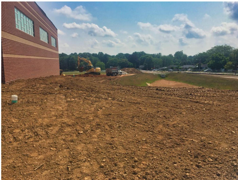
View of final grading being done at Gym.
