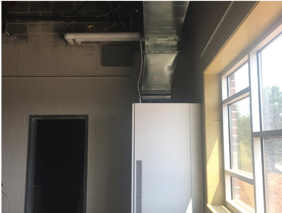
View of ductwork and piping being installed on room AC units.
