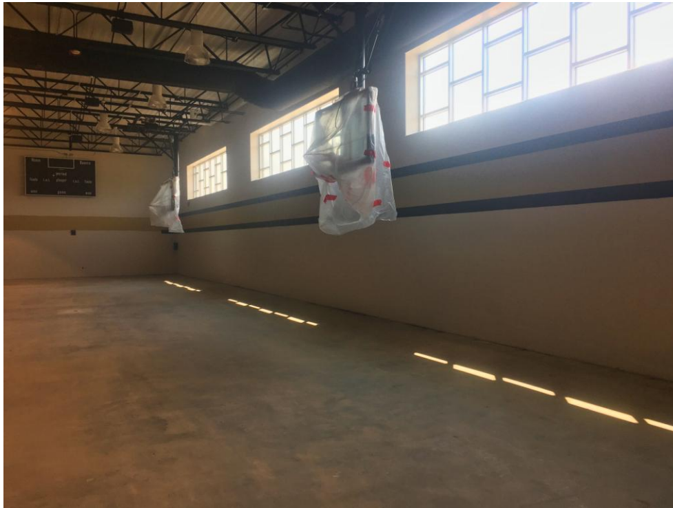
View of new backboards and wall painting in Gym.
