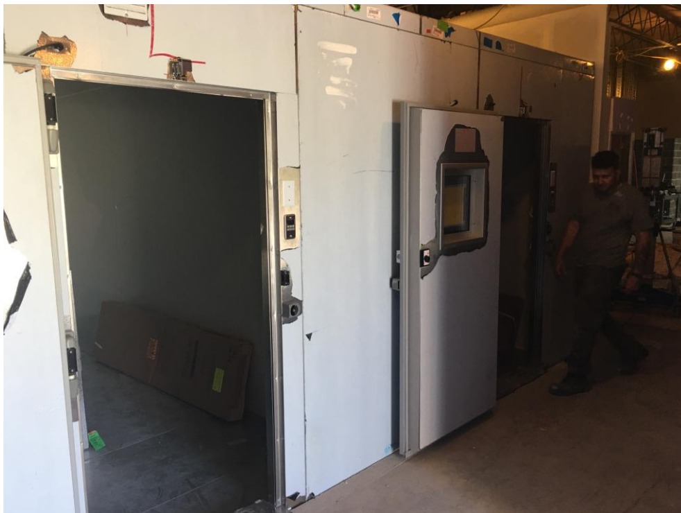
View of new Walk-Ins, in Kitchen.
