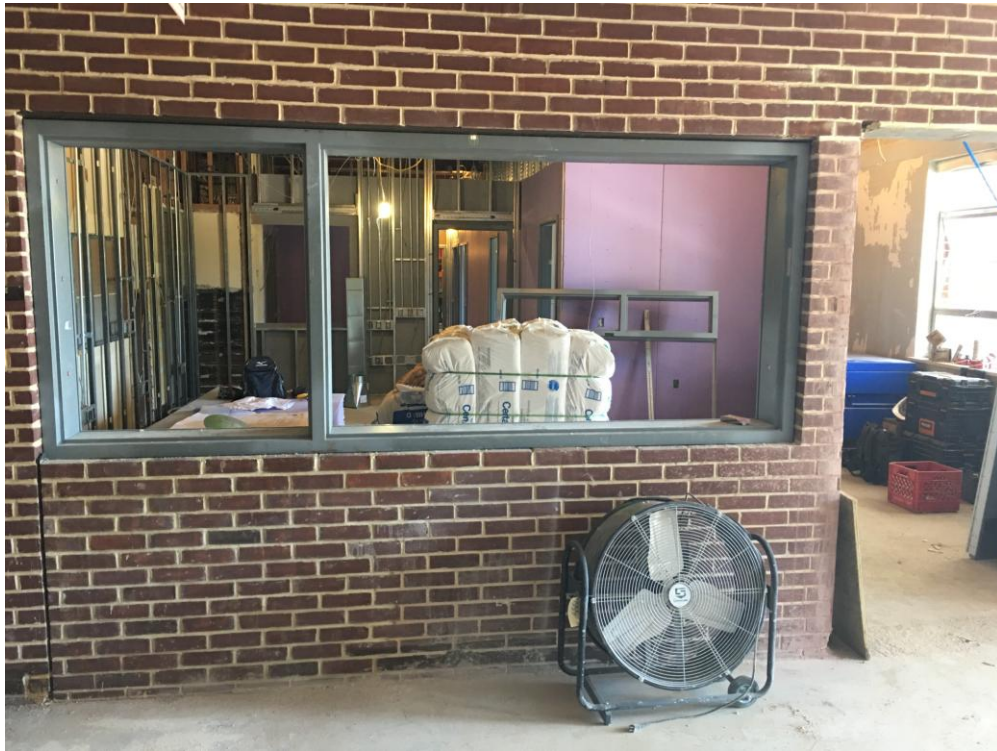
View of new entrance into Admin Suite.
