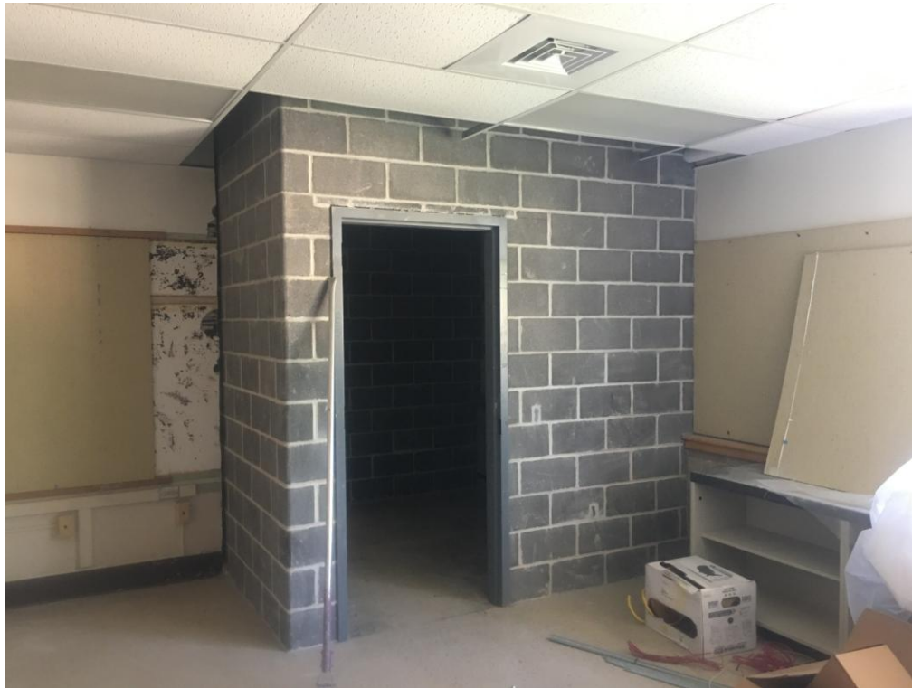
View of new Sensory Room between Behavior and Autistic Classrooms.
