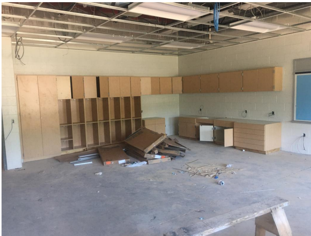
View of casework being installed in a new classroom.
