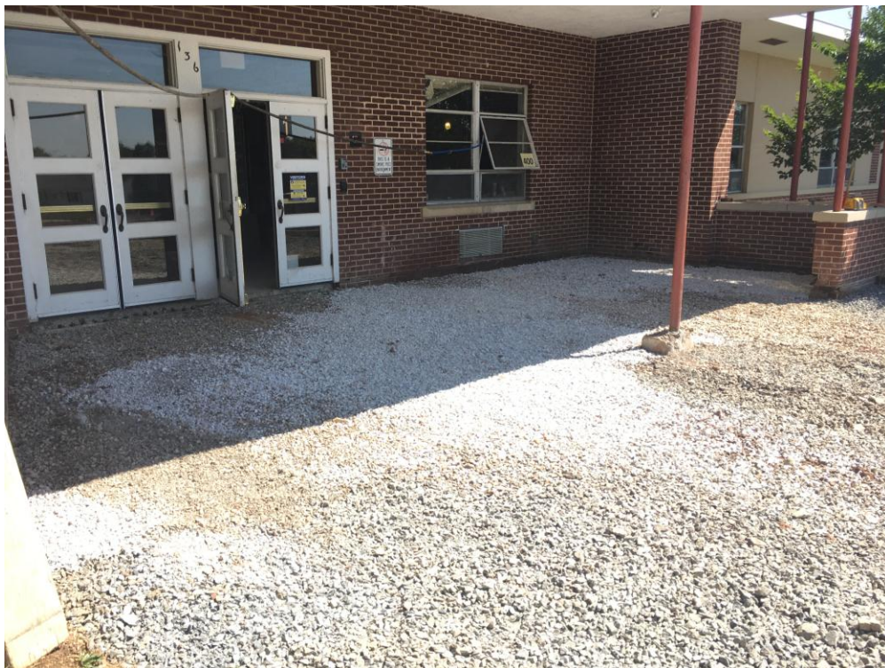
View of front entrance after removal of old concrete.
