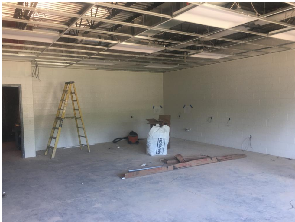
View of ceiling grid and light installation in a new classroom.
