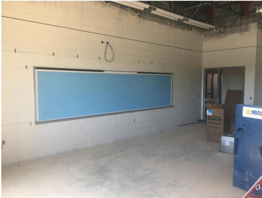
View of whiteboard installation in a new classroom.
