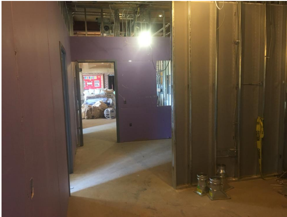
View of drywall work in Admin Suite.
