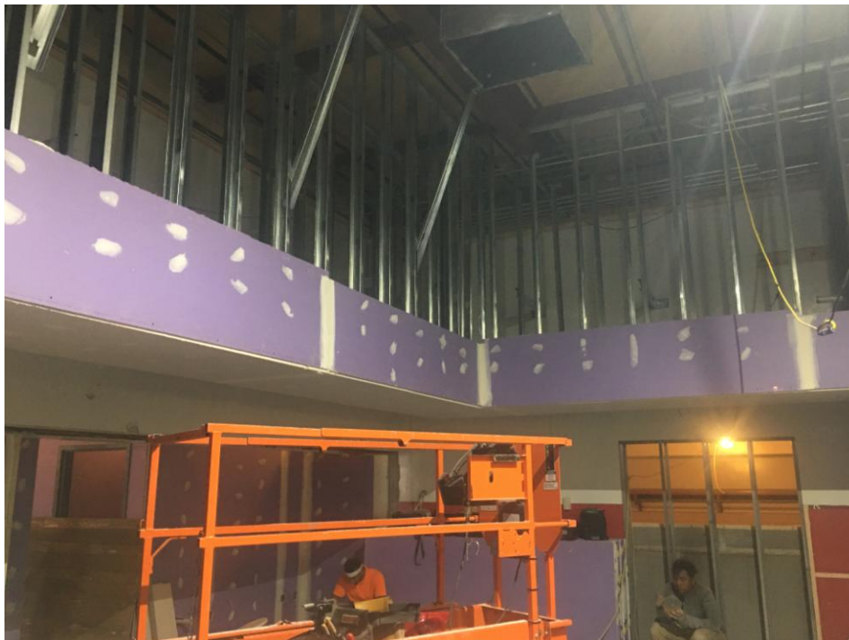
View of drywall work in Kitchen area.
