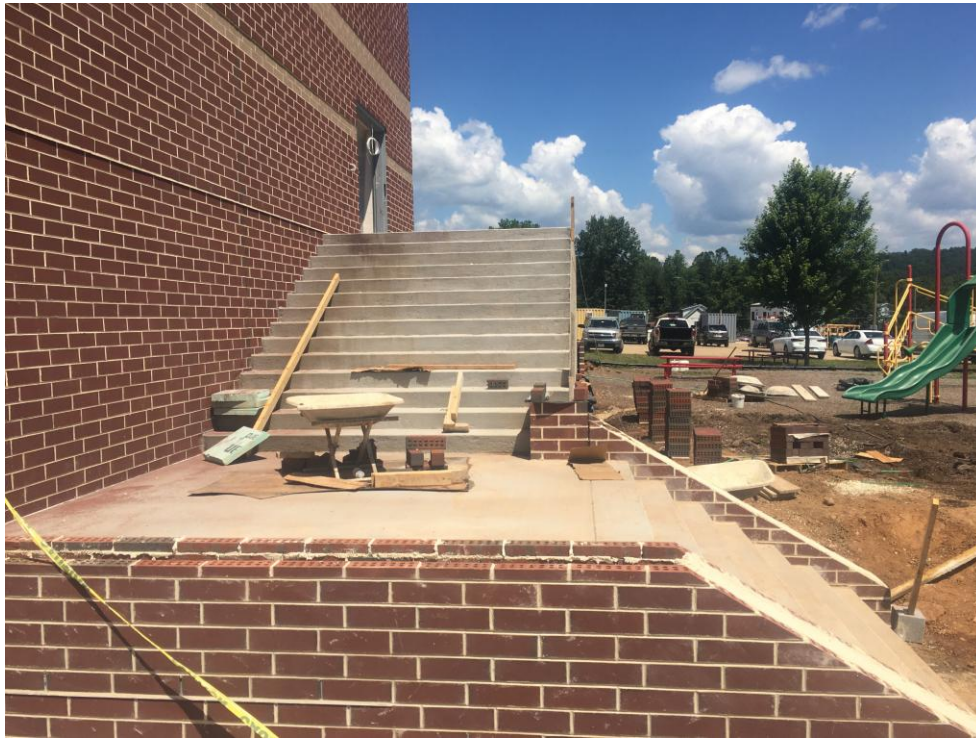
View of exterior Gym stairs.
