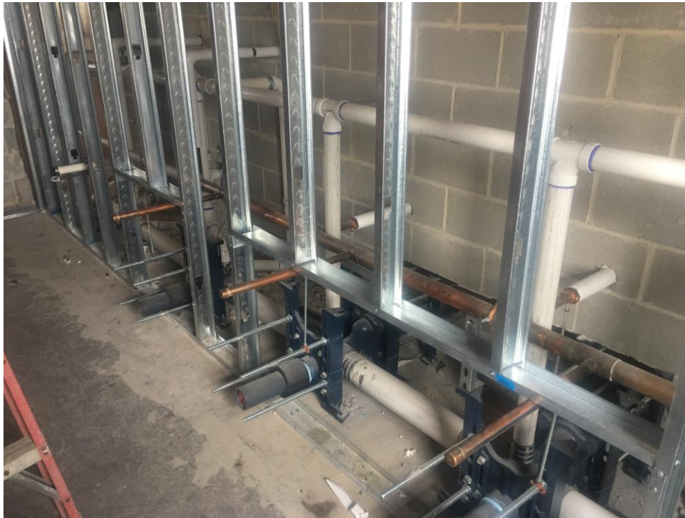
View of renovated Restroom across from Administration.
