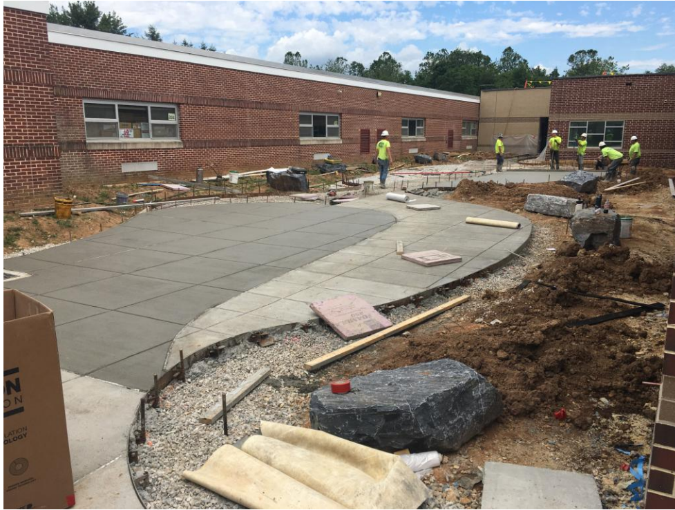
View of Classroom Addition Courtyard.
