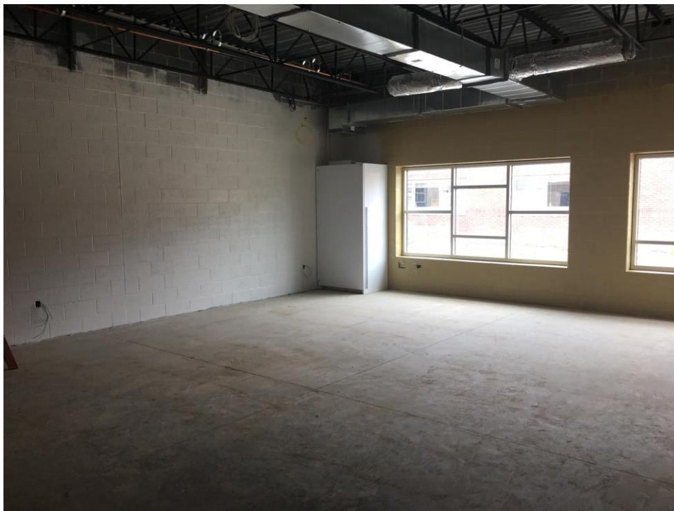
View of new Classroom with AC unit.
