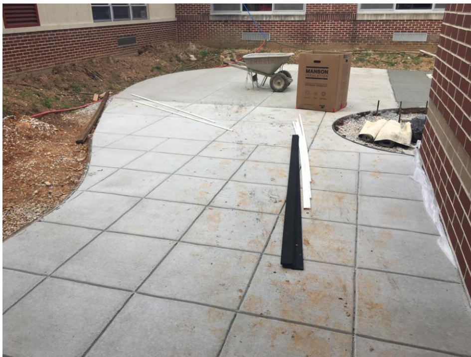
View of Classroom Addition exit to Courtyard.
