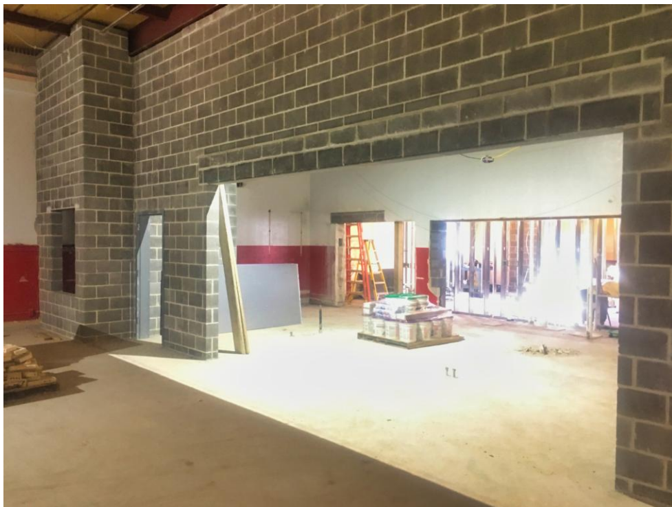
View from Cafeteria into Food Court/Serving Area.
