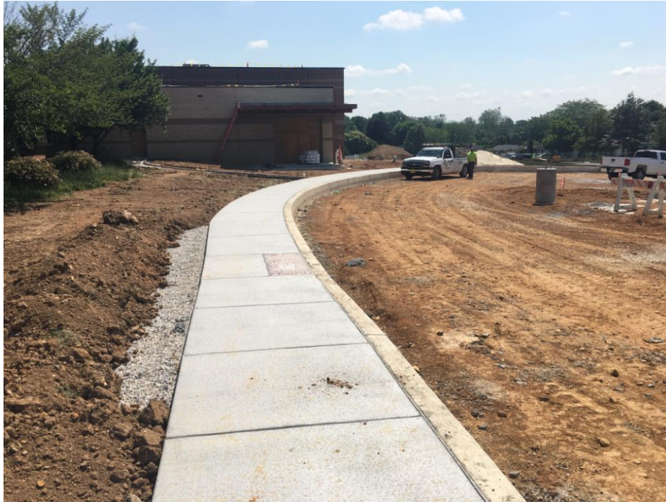
View of front sidewalk towards Gym.
