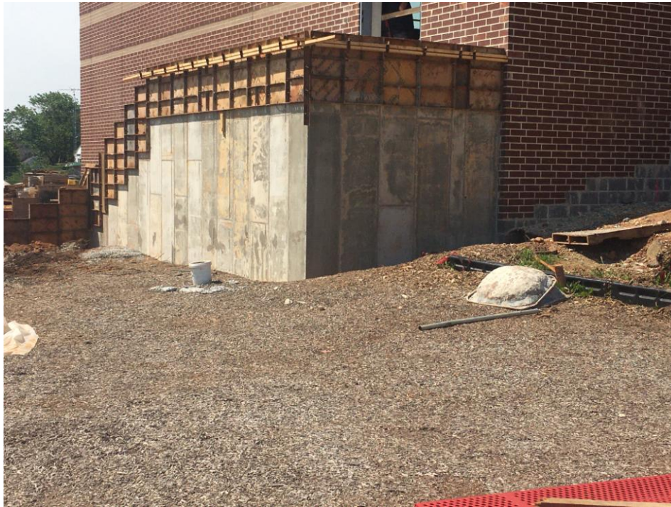
View of exterior Gym stairs being formed.
