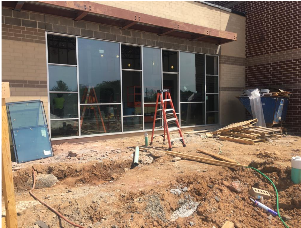
View of installation of storefront glass at Gym entrance.
