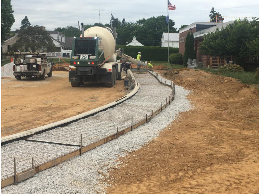
View of new sidewalk being poured at front entrance.
