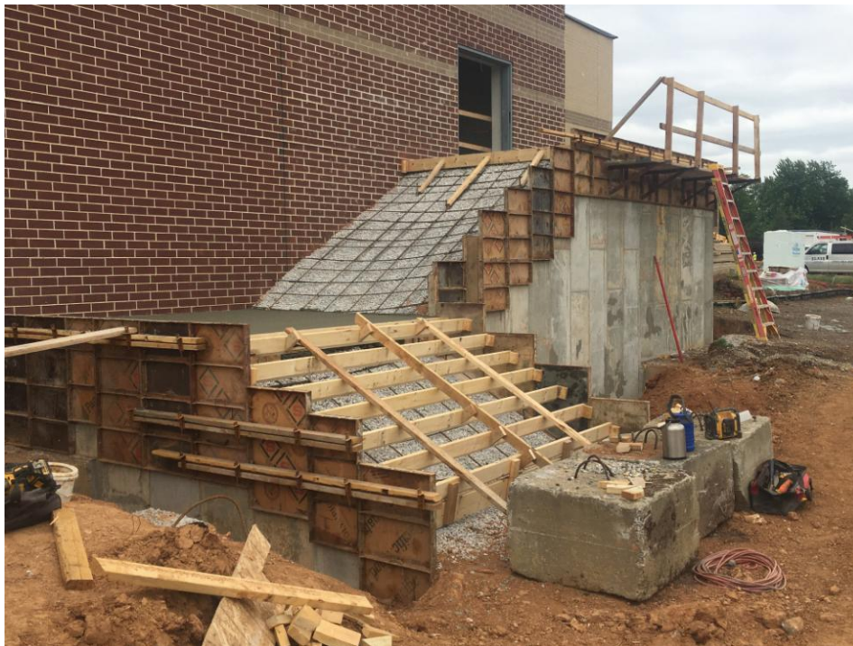
View of exterior Gym stair risers being formed.
