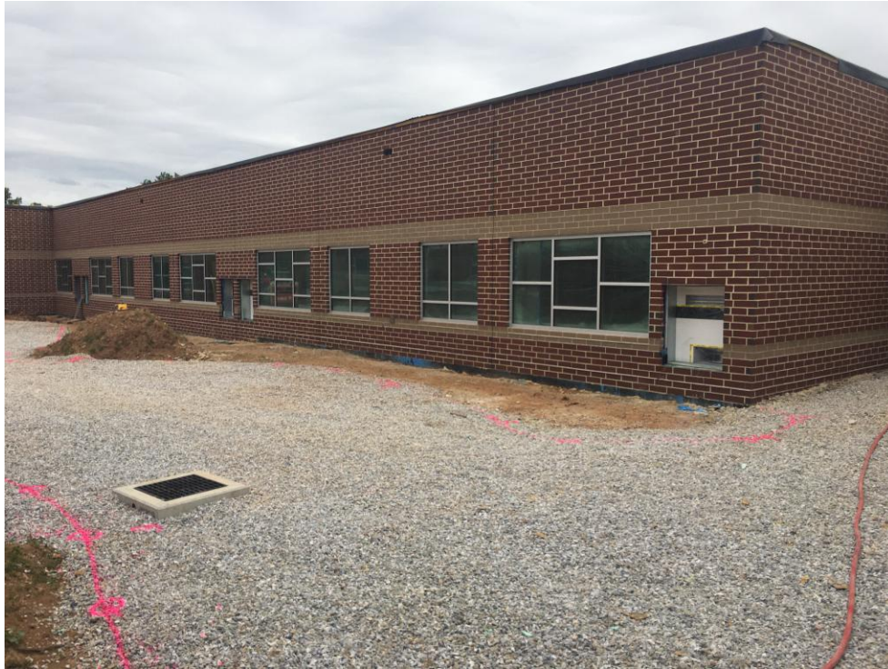
View of new Classrooms from new Courtyard.
