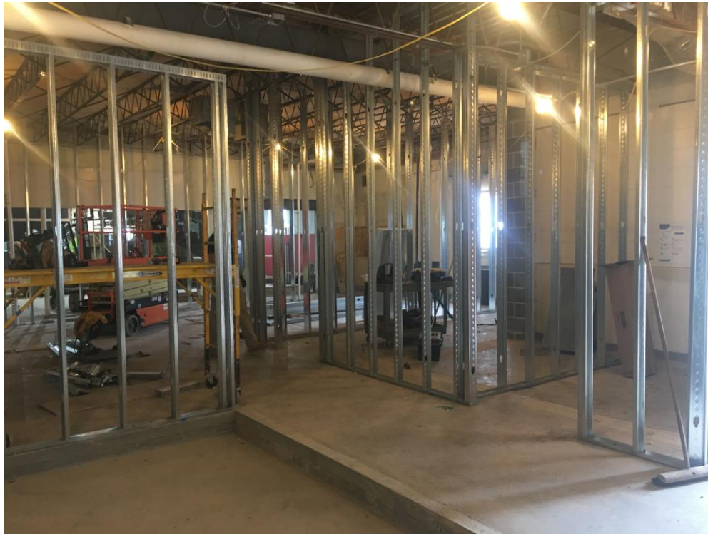
View of framing for new Kitchen offices and Slab for Walk-In Coolers.
