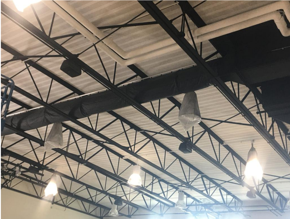
View of Gym ceiling and joists after painting with duct sock in place.
