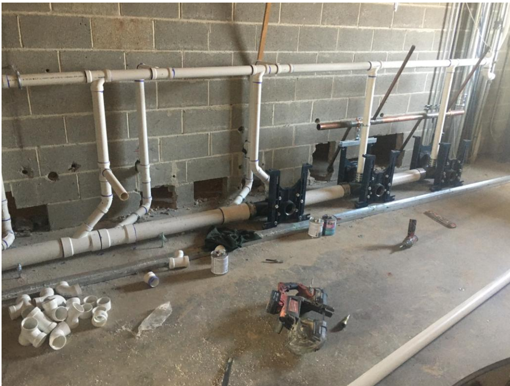
View of piping for renovated Bathrooms across from Admin Suite.
