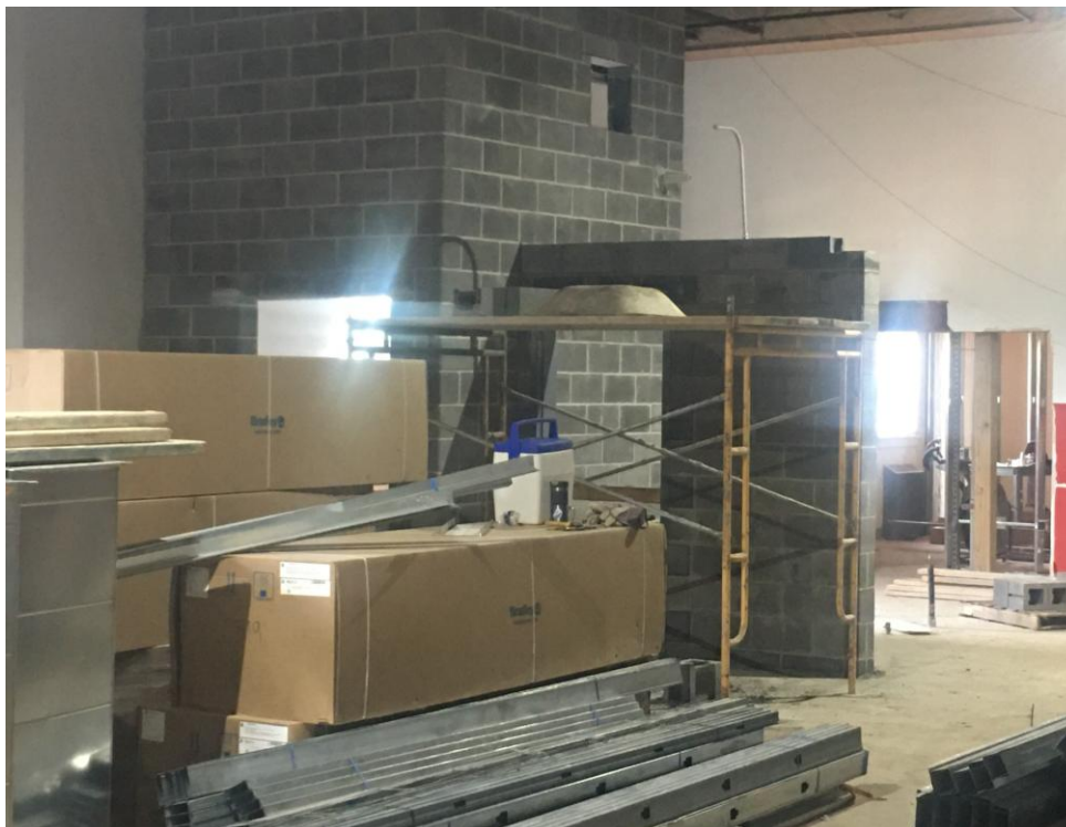
View of masonry walls being erected in Cafeteria/Kitchen area.
