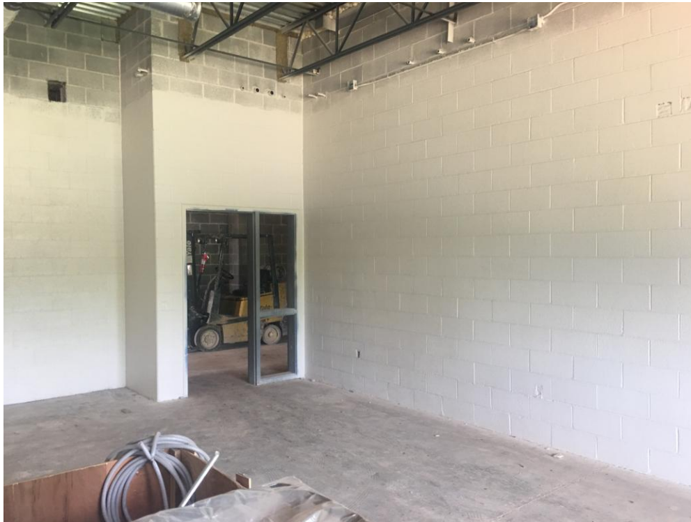
View of one of the new classrooms.
