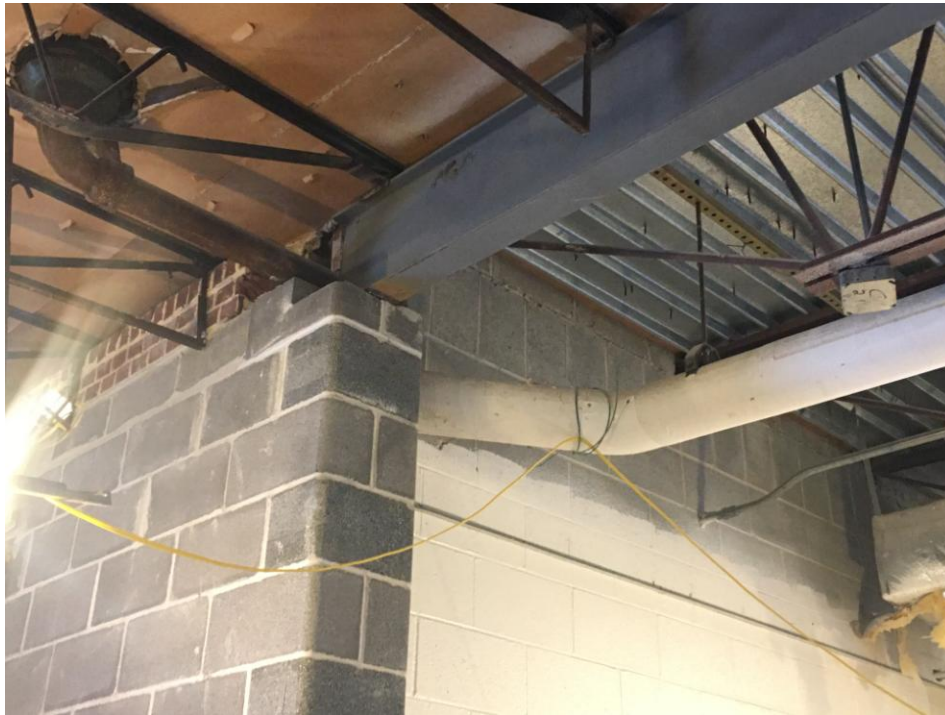
View of new beam between in Kitchen.
