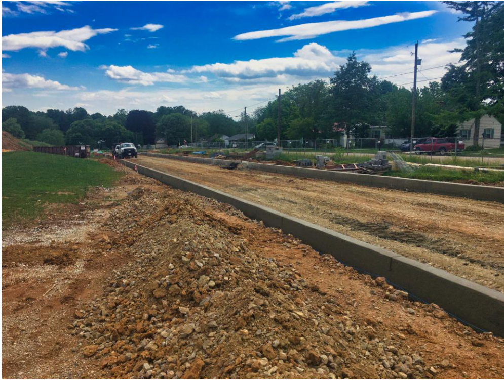
View of new curbing at new entrance drive on Fohl St.
