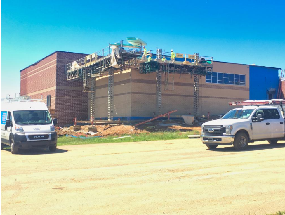
View of North and East side of New Gym.
