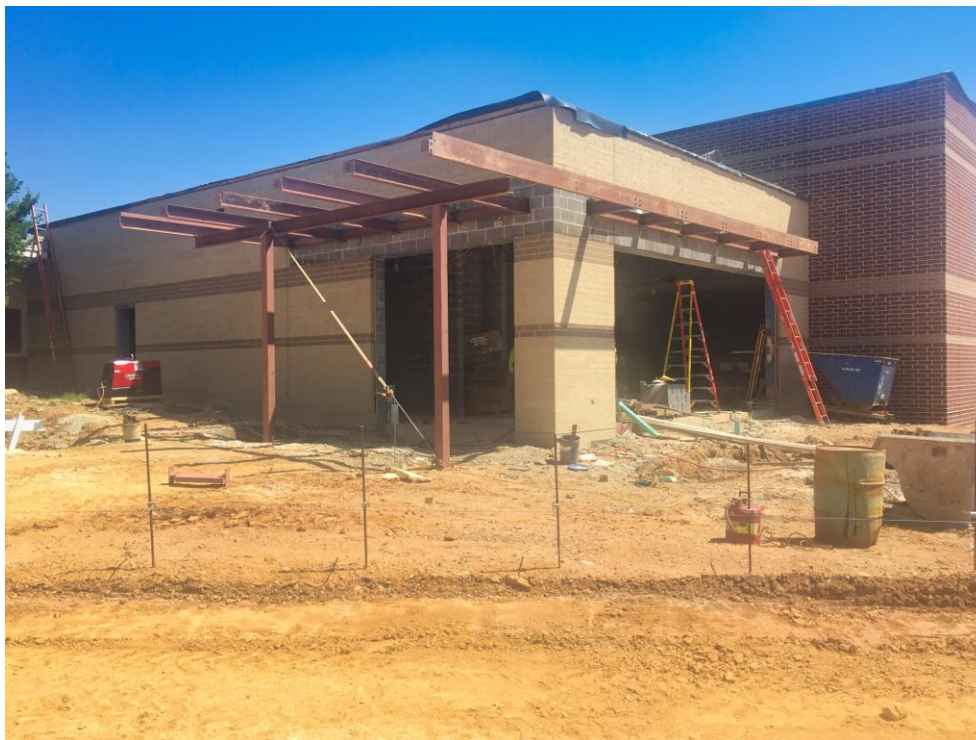
View of Gym entrance canopy being erected.
