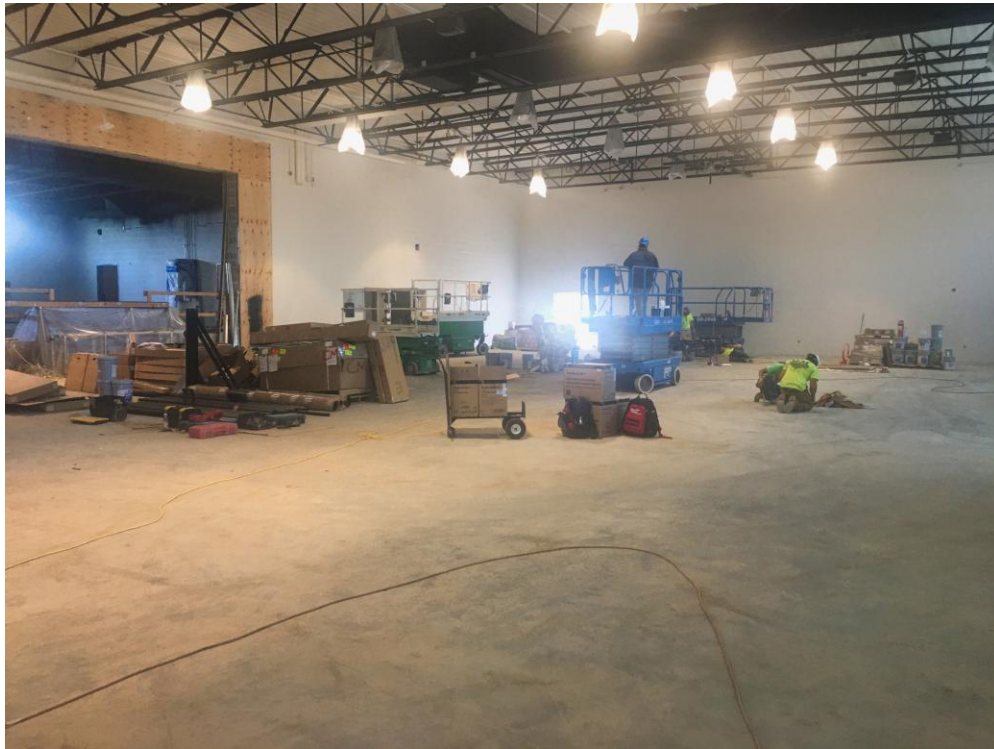
Interior view of Gym and Proscenium Façade of Platform..
