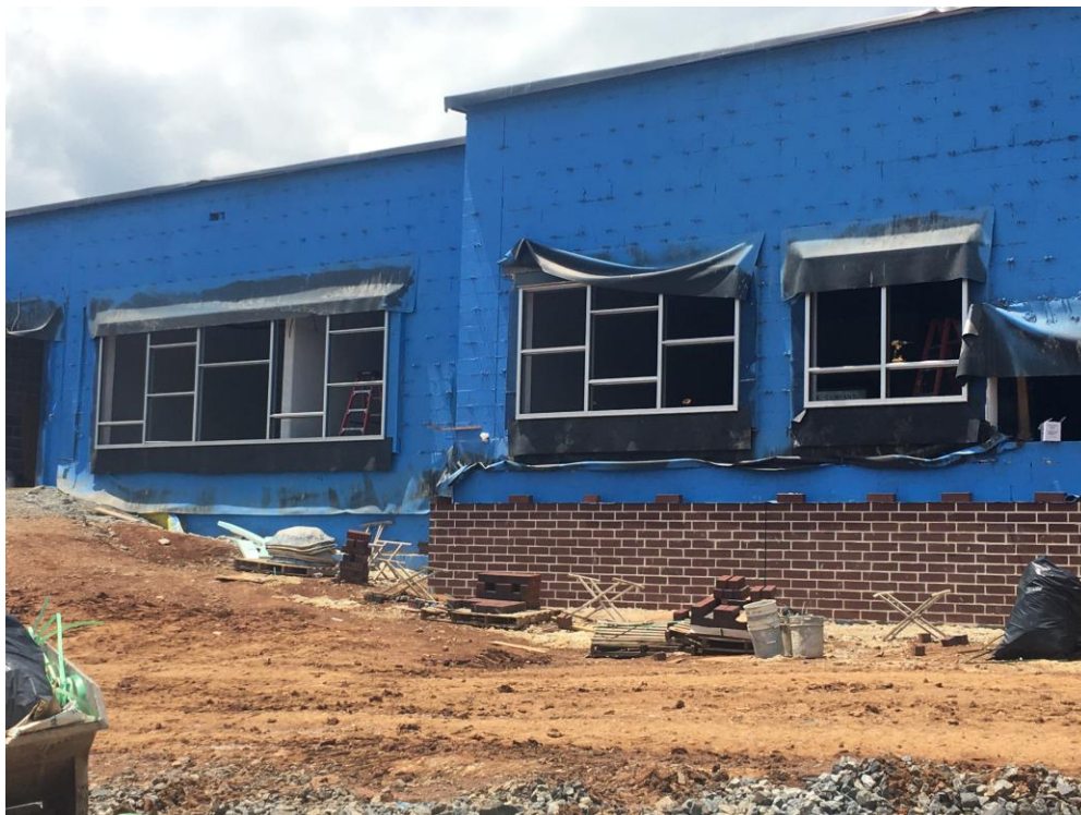
View of new windows on East side of Classroom Addition.
