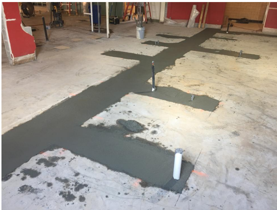
View of plumbing rough-ins for new Kitchen Equipment.
