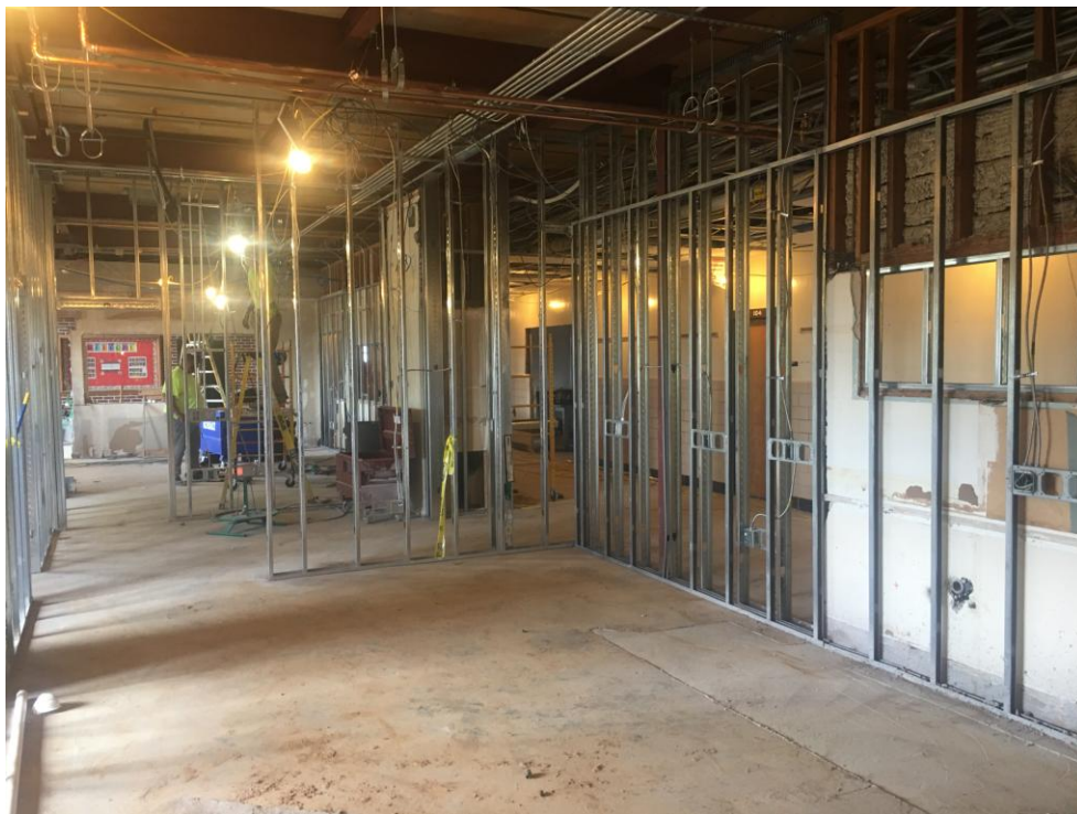
View of Administration Suite prior to start of drywall.
