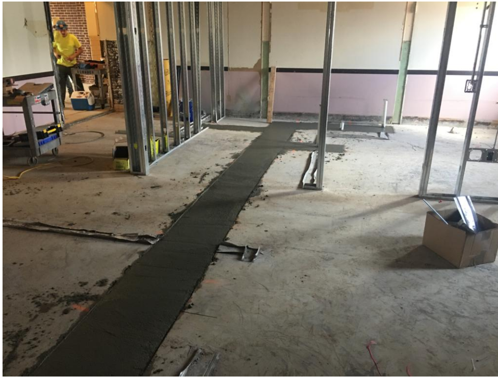
View of plumbing rough-ins in Nurse's Suite.
