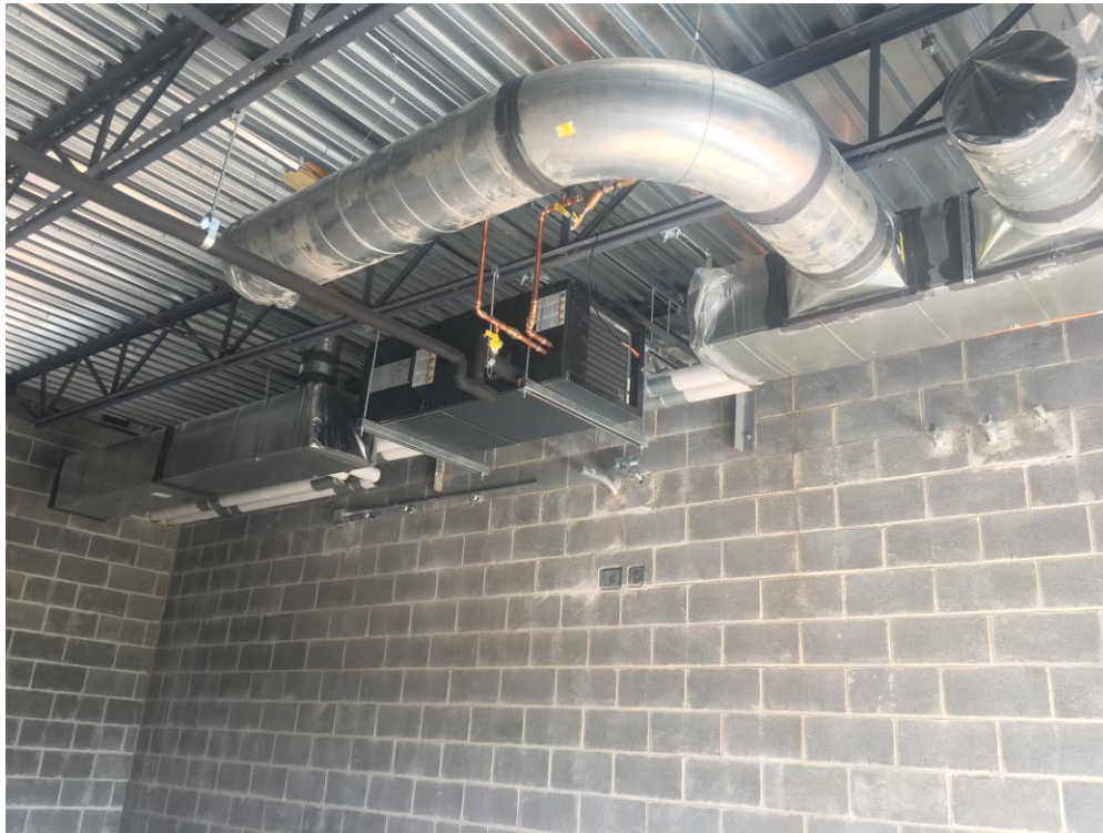
View of duct work being installed in new Gifted Classroom.
