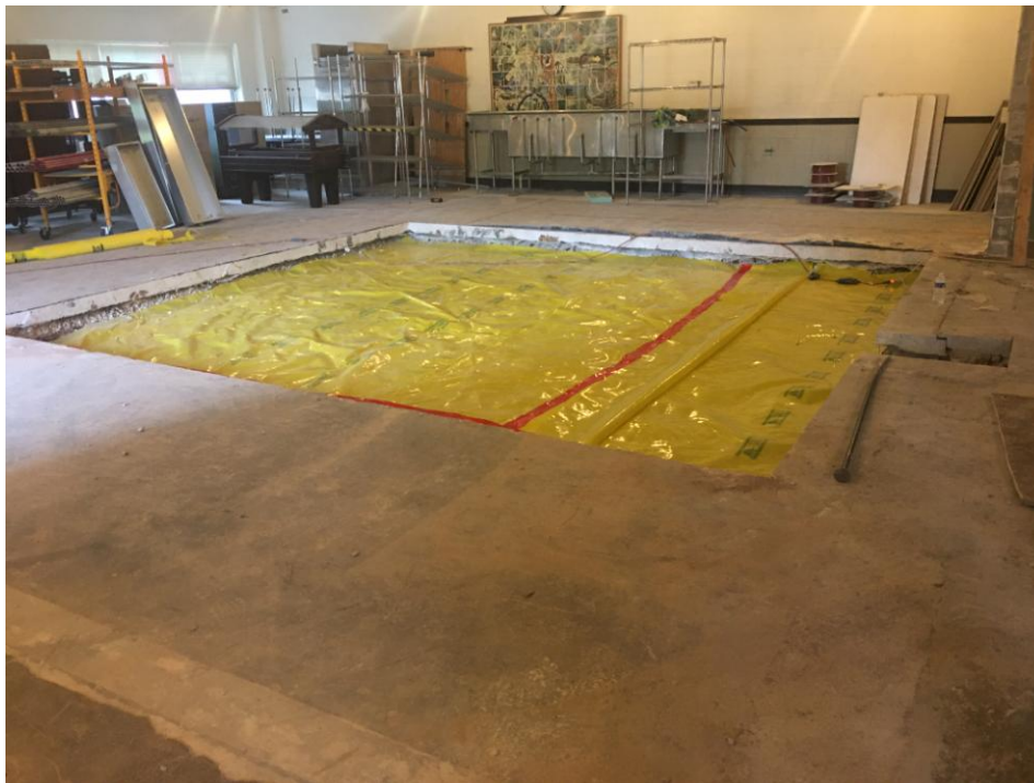
View of area prepped for concrete for the new walk-ins.
