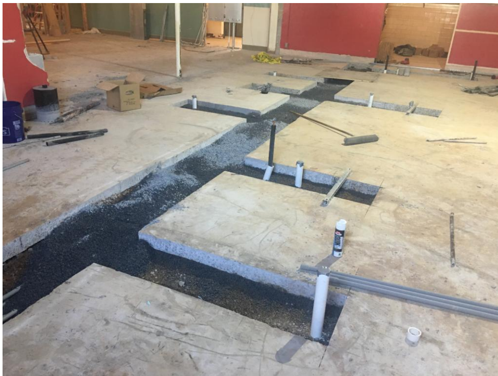
View of installed waste lines in Kitchen/Serving Line.
