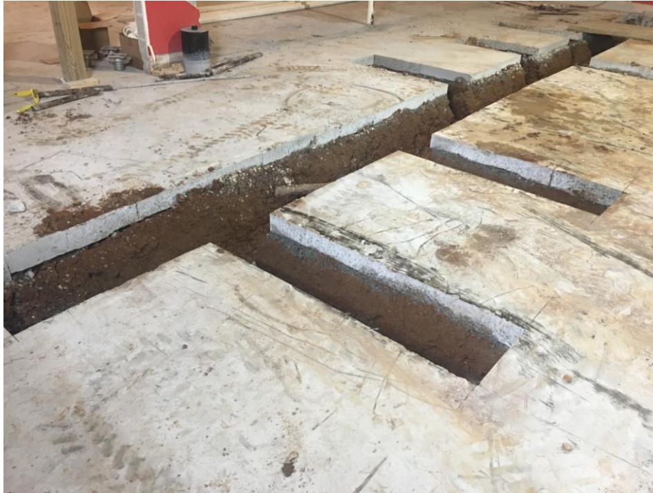
View of trenches for new Kitchen/Serving Line equipment.
