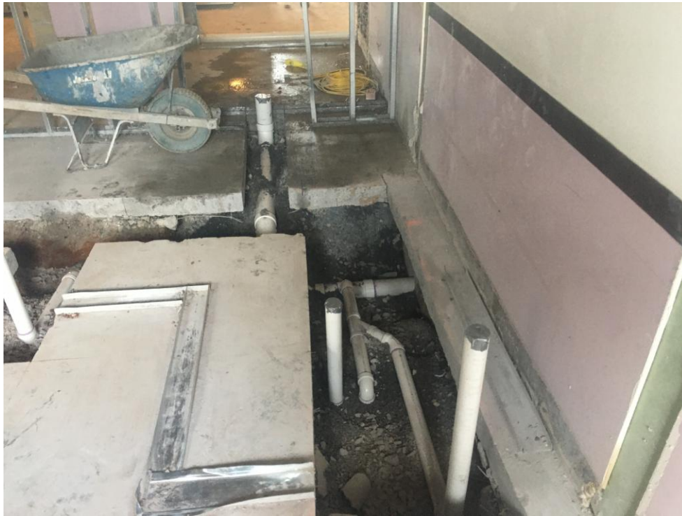
View of plumbing work in Nurse's Suite.
