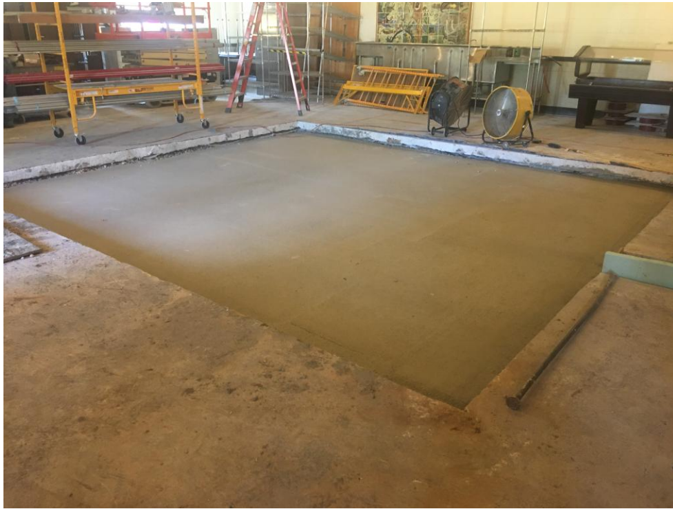
View of new slab for walk-ins.
