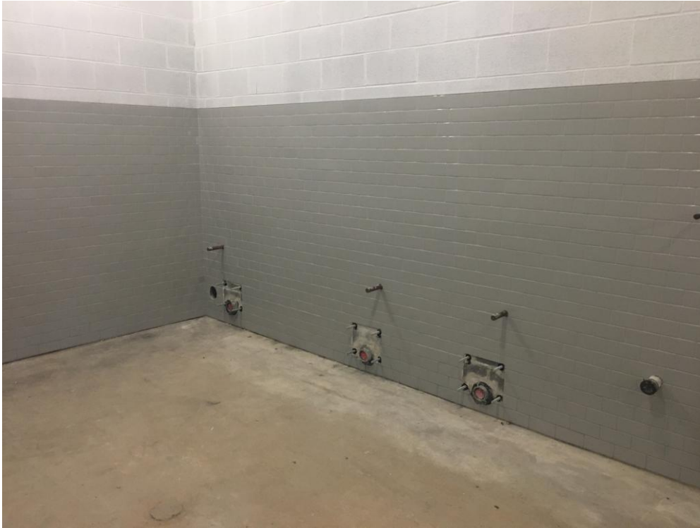
View of tile installed in new Gym Male Bathroom.
