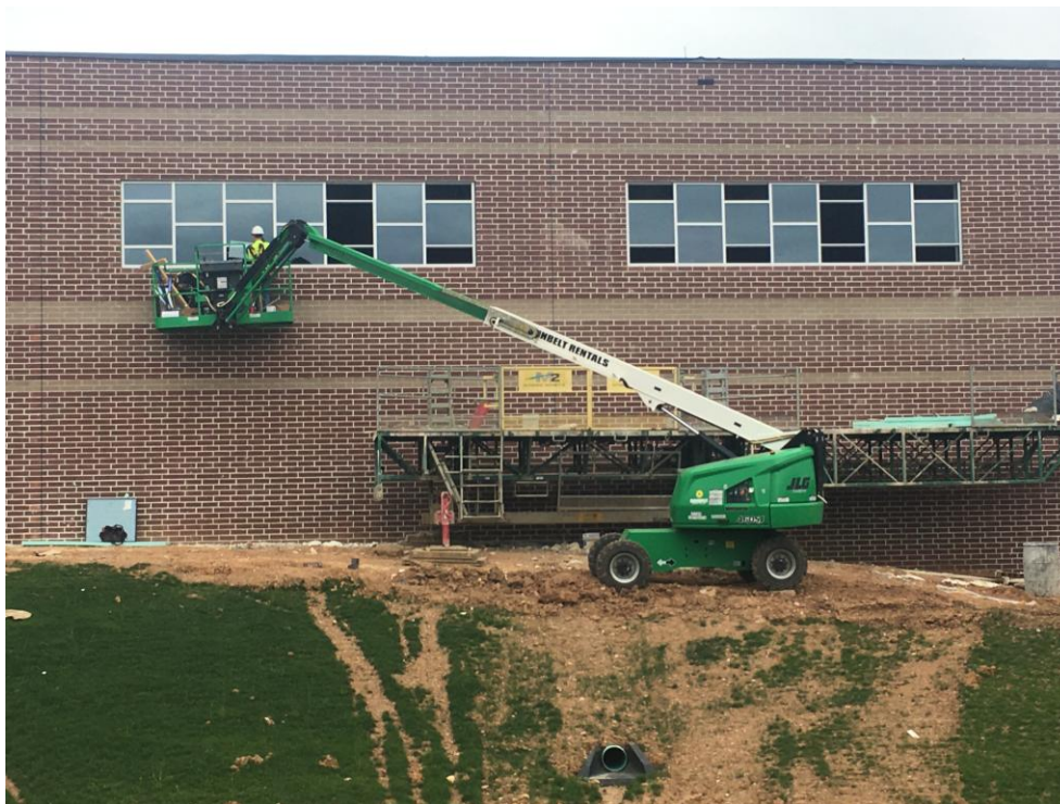
View of windows being installed in the South wall of the Gym.
