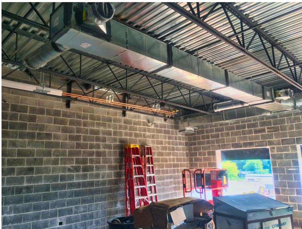
View of duct work being installed in a new classroom.
