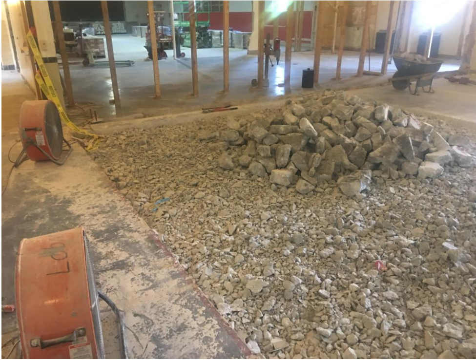
View of floor demo for new walk-ins, in the kitchen..
