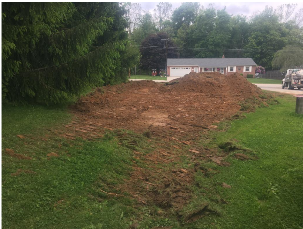
View of beginning of grading along West side of rear lot.
