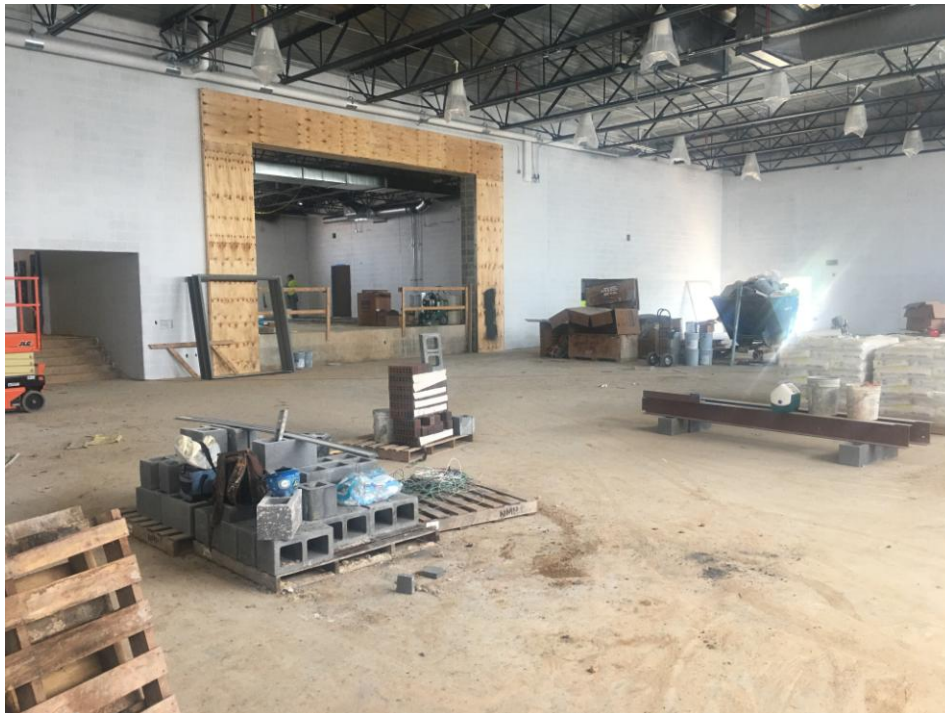
View of the Platform framing in the new Gym.
