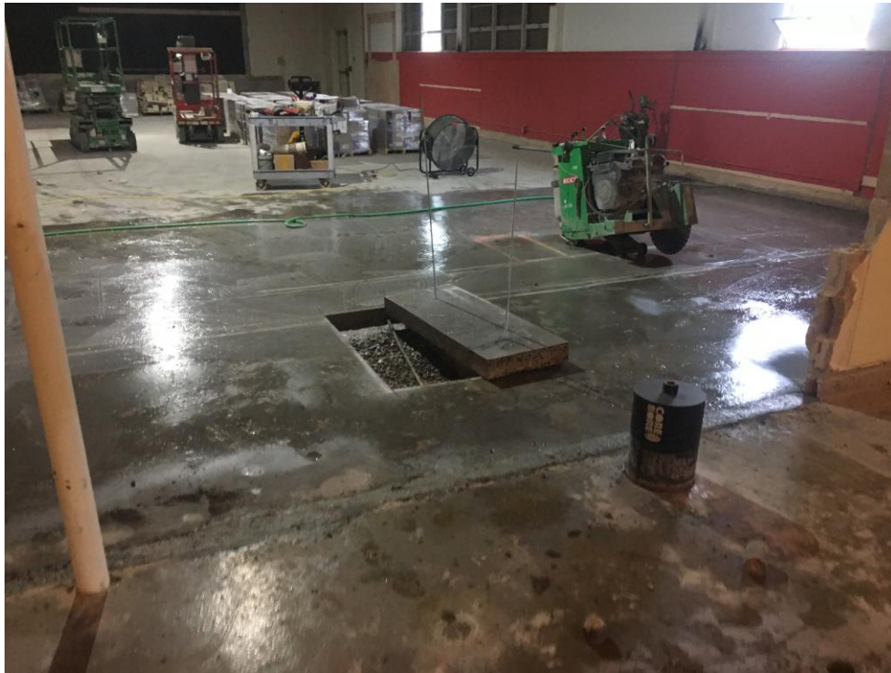
View of floor cuts being done for new Kitchen equipment.
