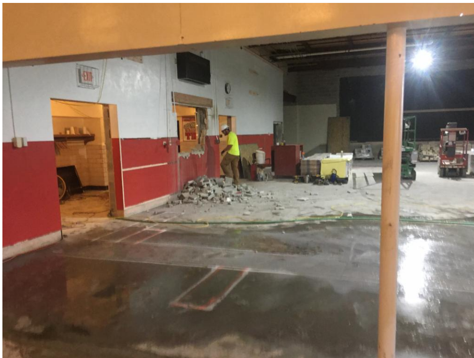
View of new doorway being opened into new Cafeteria area..
