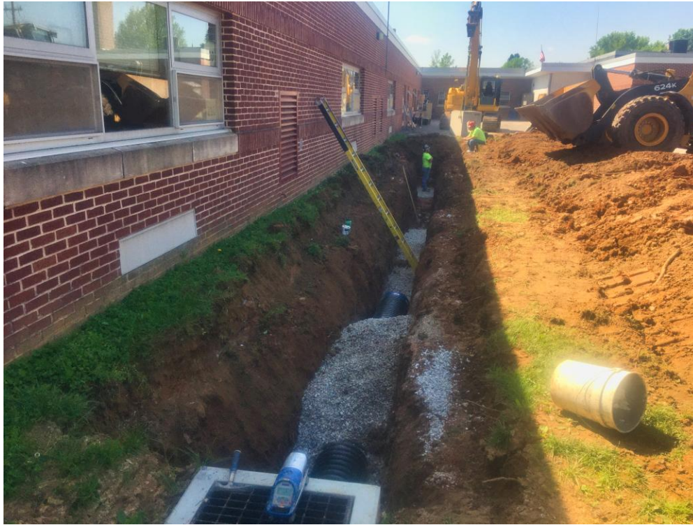
View of new storm sewer line on West side of existing building.
