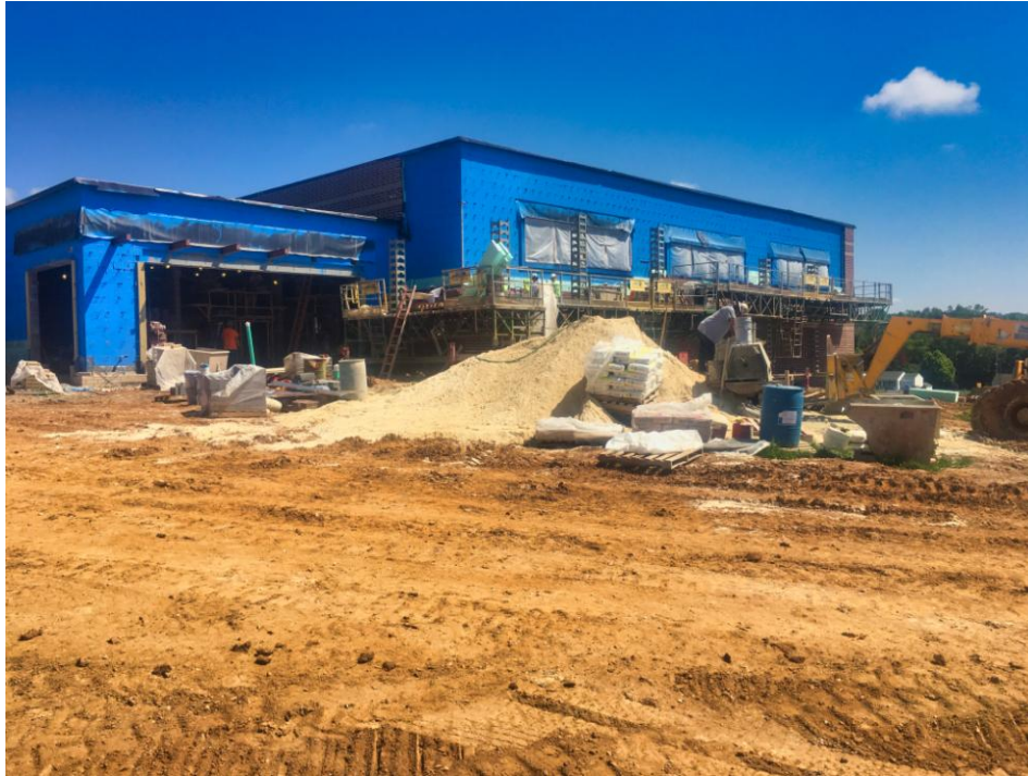
View of brick installation on the South wall of the new Gym.
