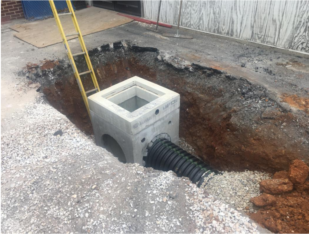
View of new storm inlet at rear entrance of old storage room.
