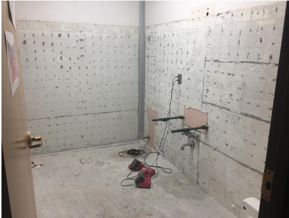
View of s Staff Bathroom after tile has been removed.
