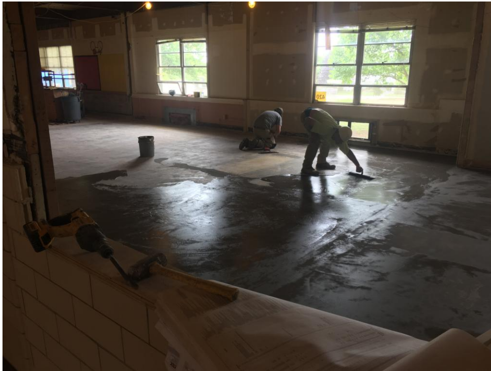
View of mastic being encapsulated in Existing Building.
