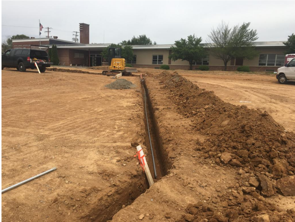
View of conduit being installed for new parking lot lighting.
