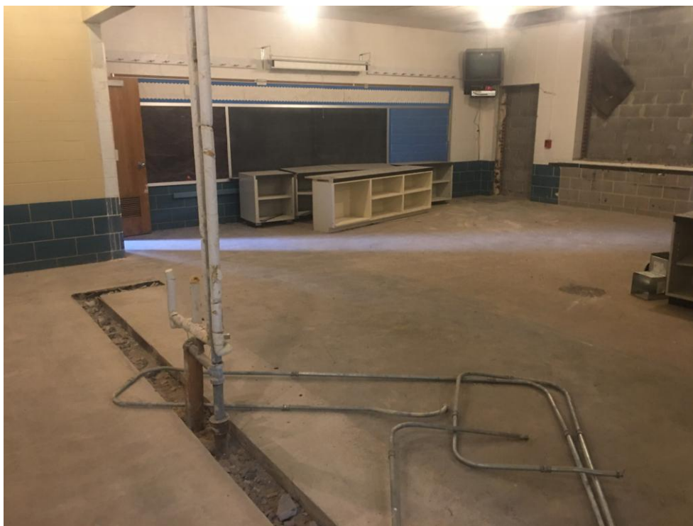
View of Music Classroom with wall removed.
