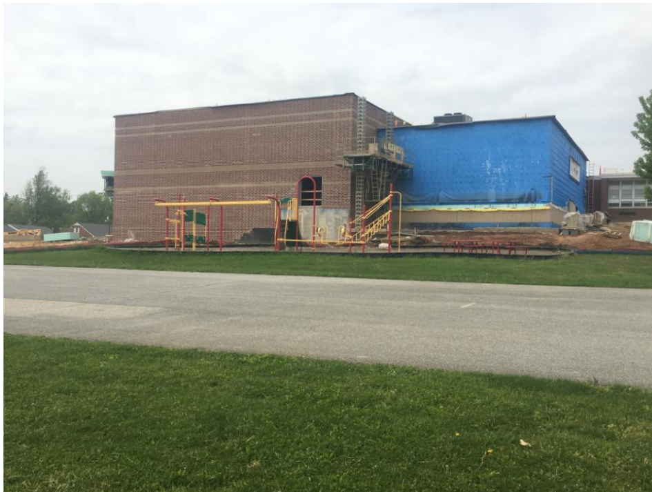
View of East wall of new Gym.
