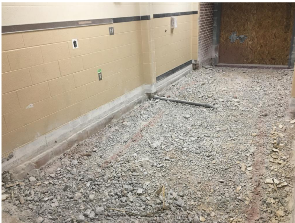
View of sewer line that will need to be replaced in connection to new building.
