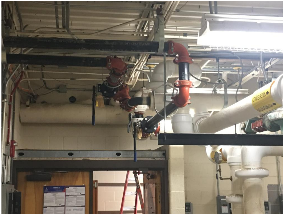
View of new heating pipe connections in existing boiler room.
