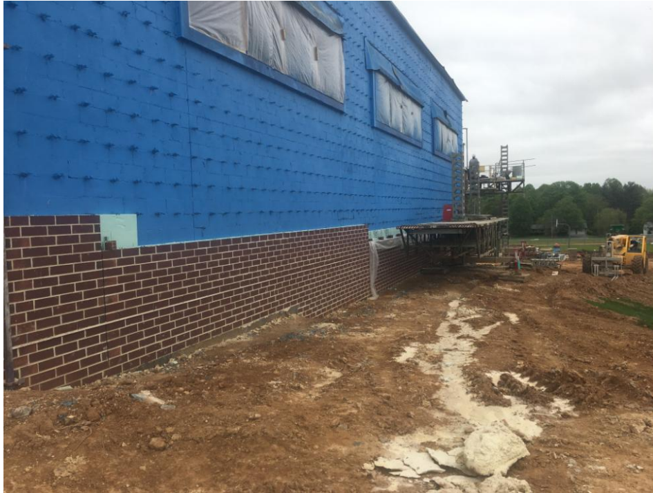
View of brick installation on South wall of new Gym.
