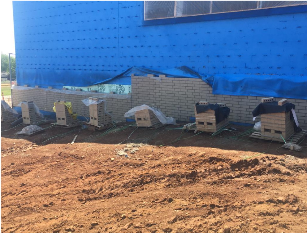
View of exterior brickwork starting on North wall of new Gym.
