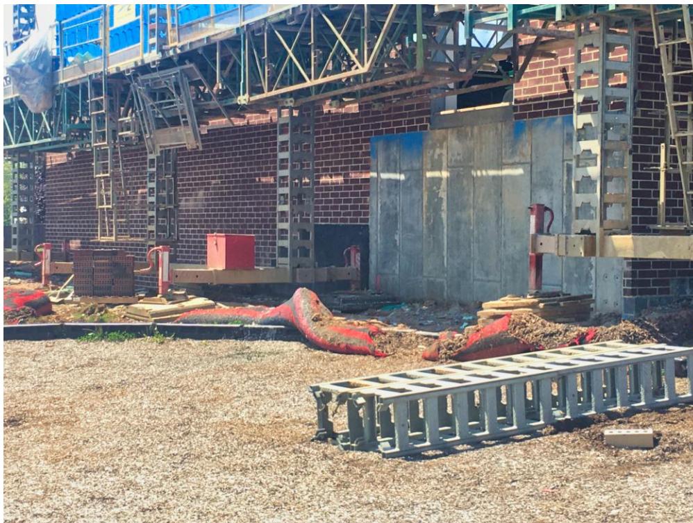
View of exterior brickwork starting on East wall of new Gym.
