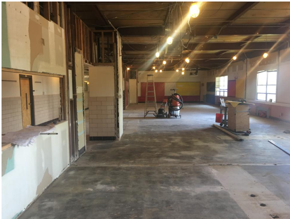
View of completed demolition on the South side of the building. You are “standing” in the old Reception area looking East.
