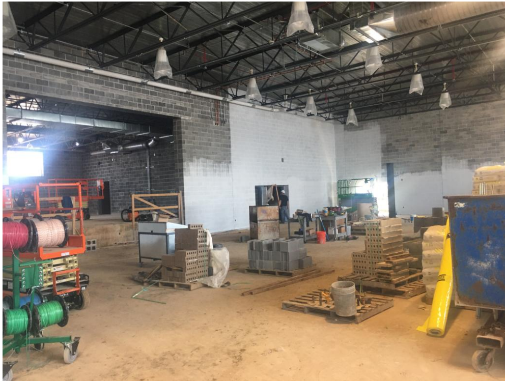
View of new Gym interior looking towards Platform. Note painting of walls has begun.
