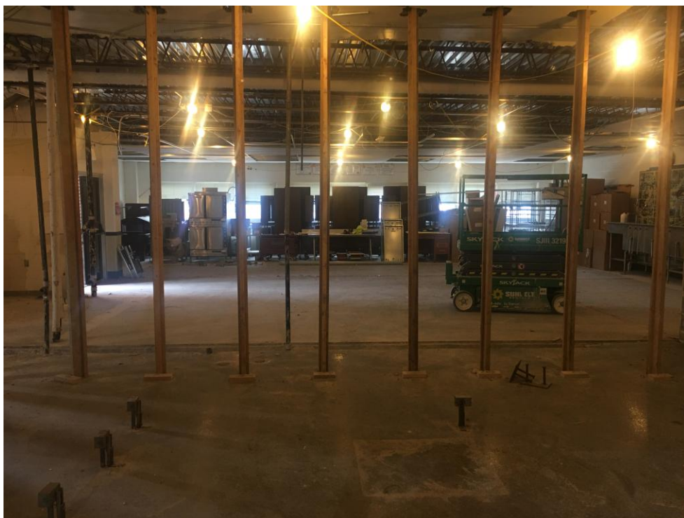
View from the old kitchen towards the cafeteria.
