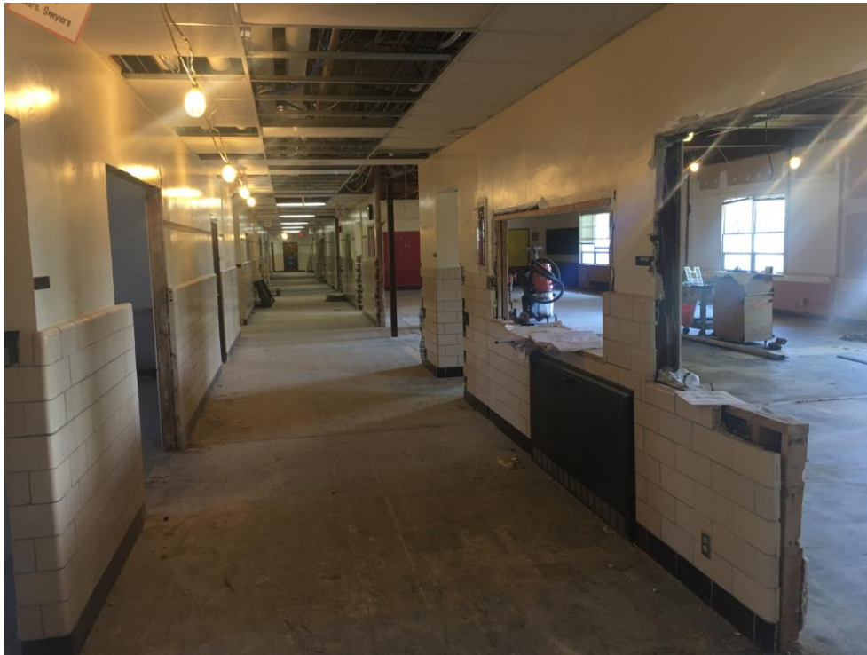
Same area, looking East, down the corridor.
