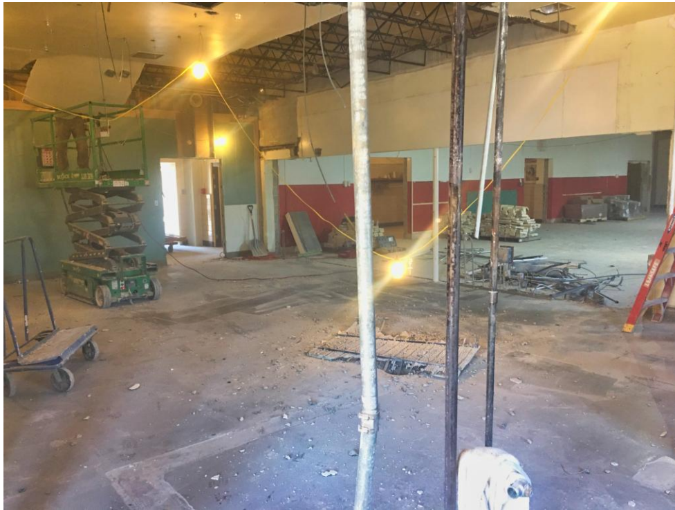
View from old Kitchen into Old Gym.
