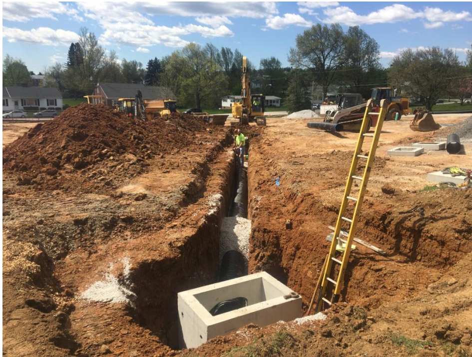
View of new storm sewer in front parking lot.
