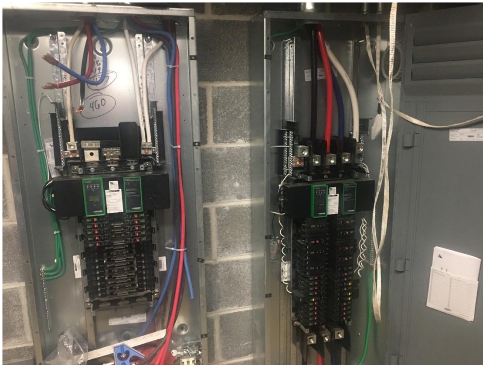
View of new electrical panels being wired.
