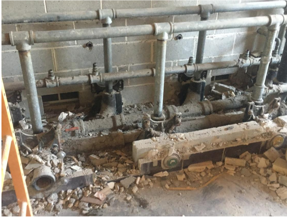
View of old sewer pipes grouted into concrete floor.
