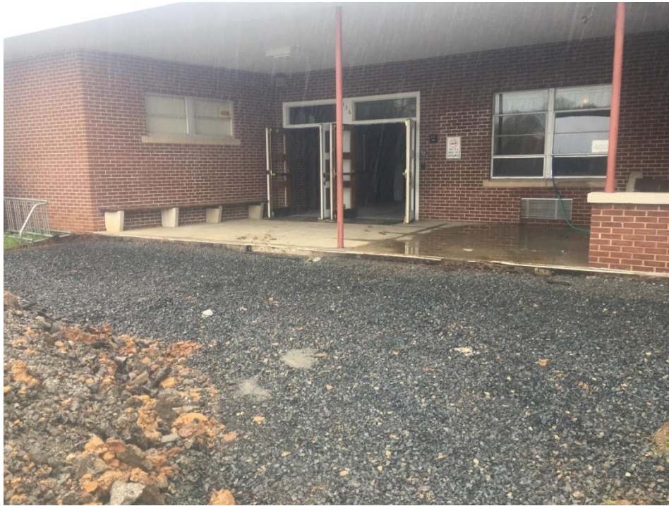
View of front entrance after concrete was removed.
