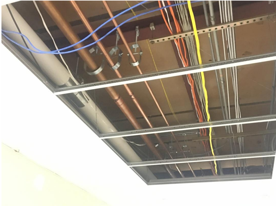
View of new piping in existing hall from Office towards New Gym.
