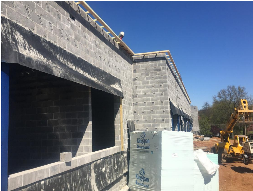
View of roof blocking being installed on Classroom Addition.
