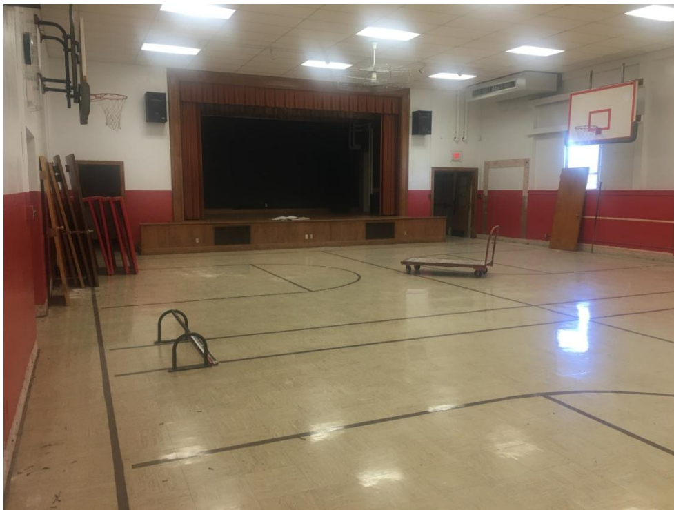
View of demolition work starting in existing Multipurpose Room.
