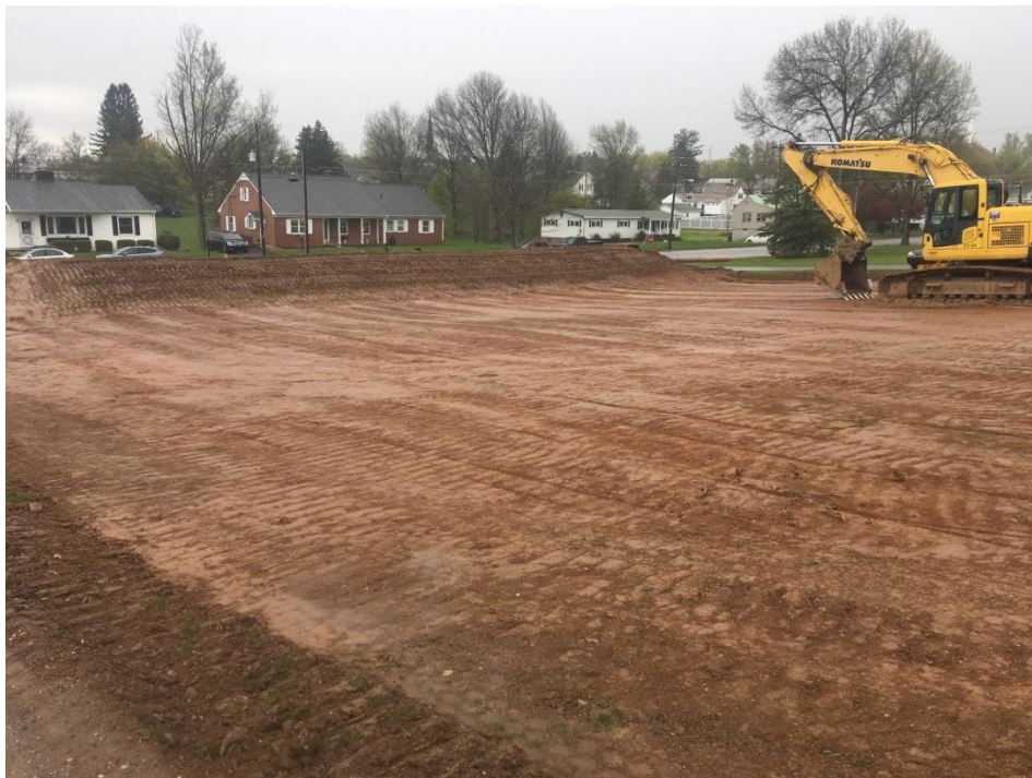
View of future front parking lot with topsoil stripped.
