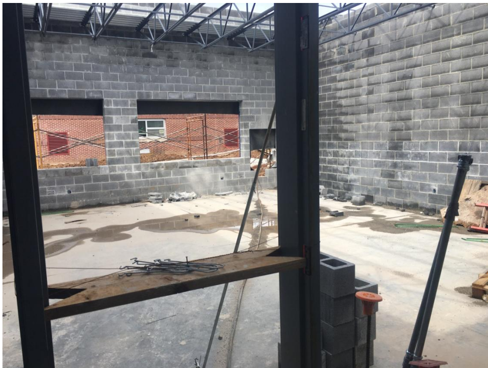
View of new Classroom further North without steel decking.
