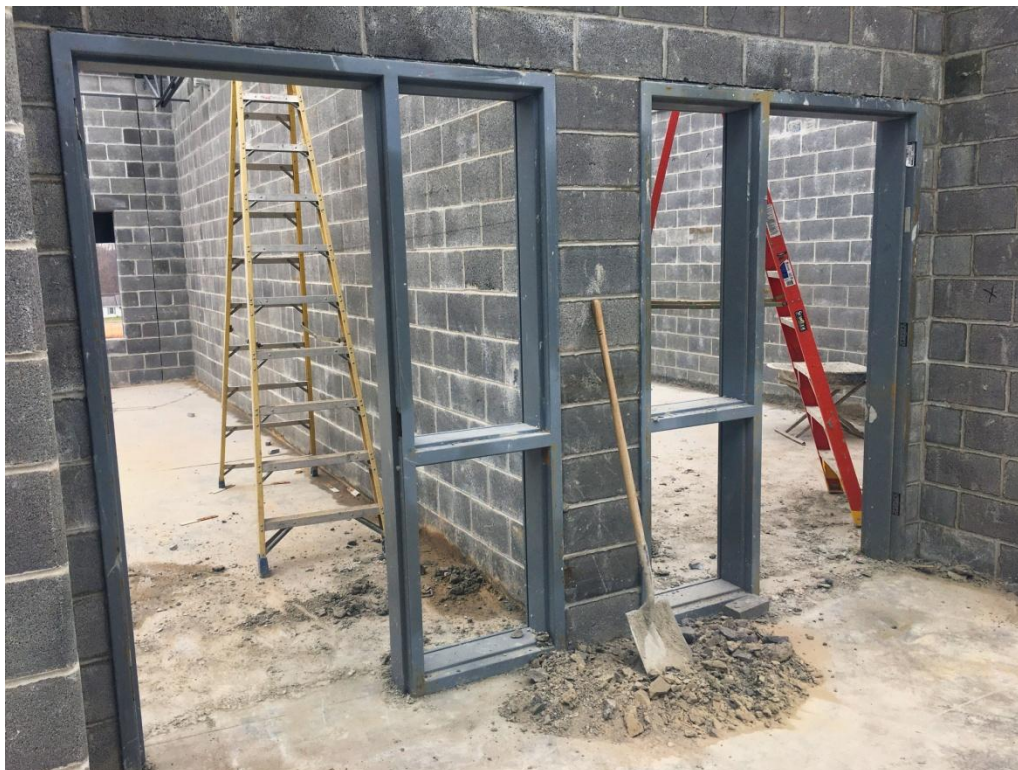
View of Classroom entrance doorbucks.
