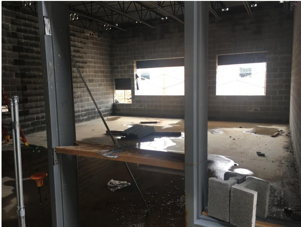
View of new Classroom and steel decking that was installed prior to shutdown.
