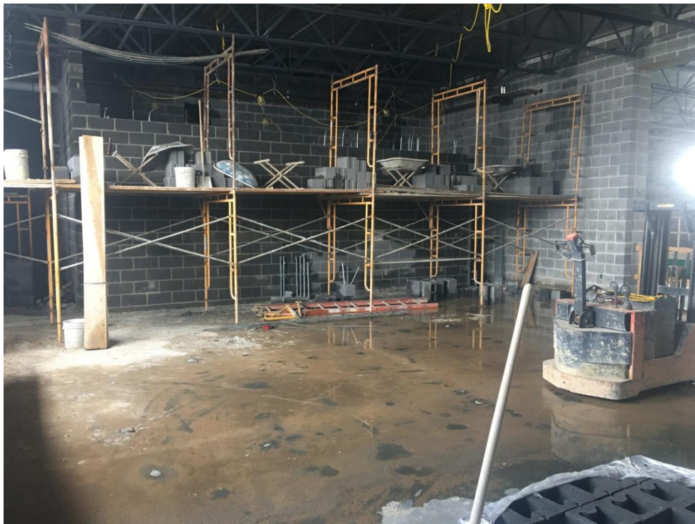
View of where Masons stopped on Stage Platform.
