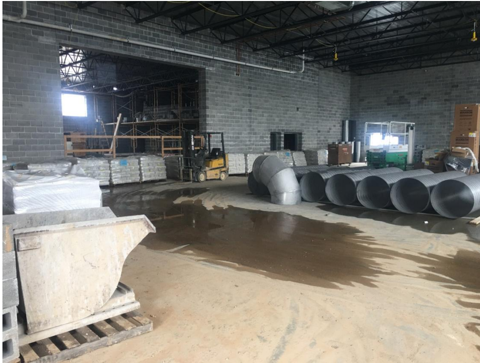
View of Gym interior.
