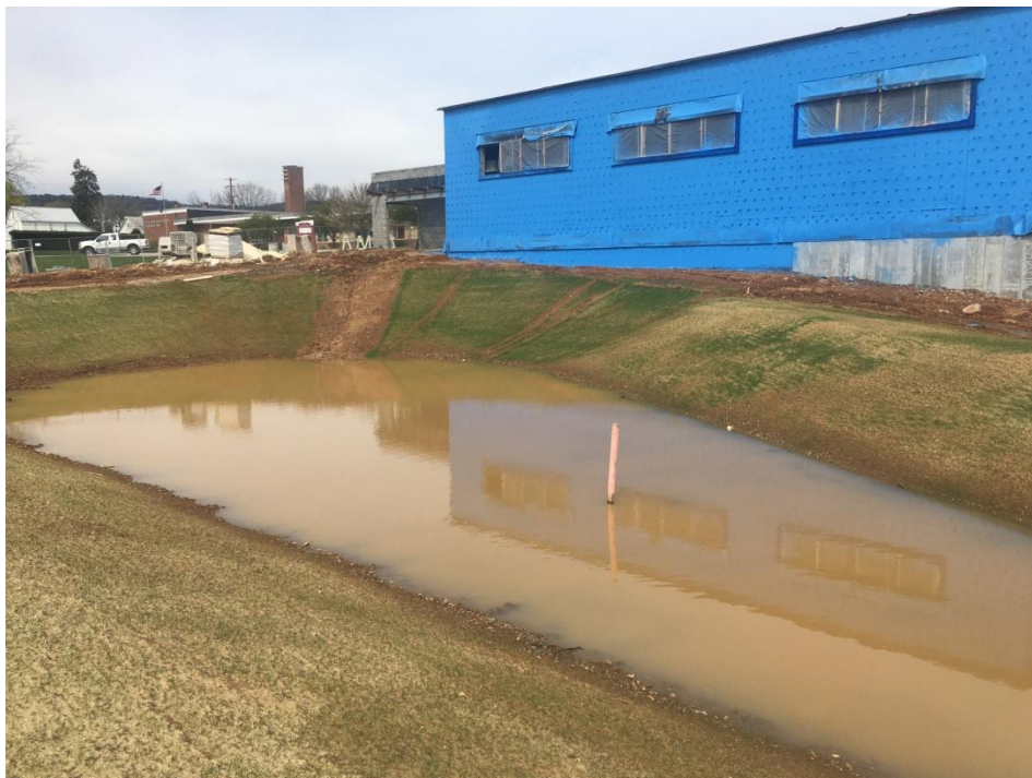
Detention Pond at South side of Gym showing grass growth.
