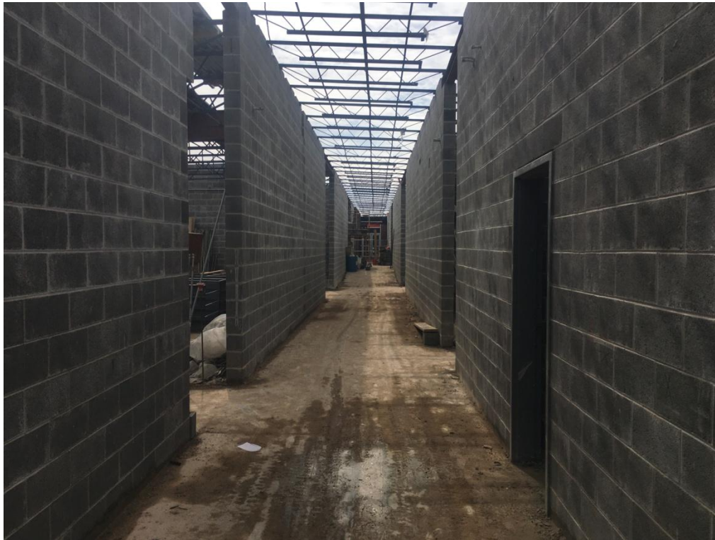
View of Classroom Addition north/south corridor.
