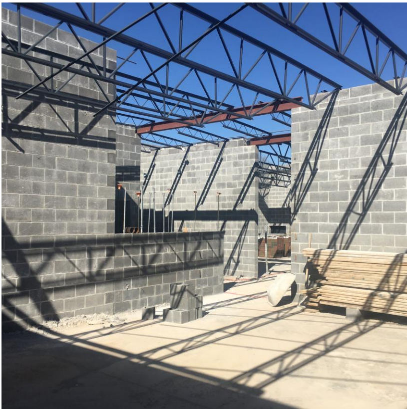
View of Classroom Addition showing steel joists.
