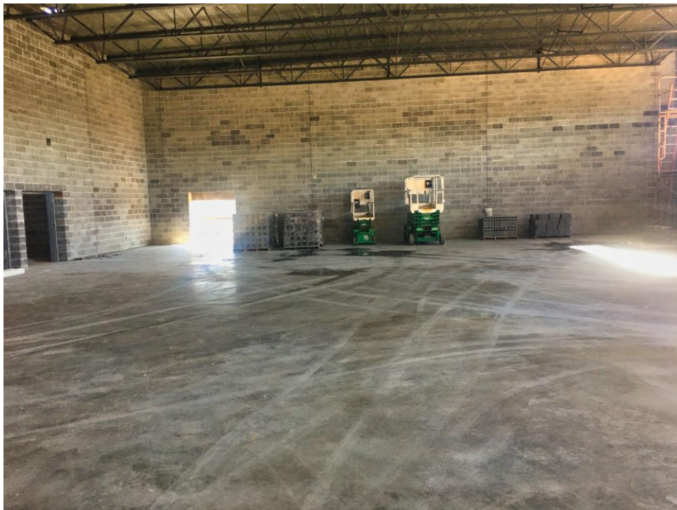
View of Gym interior facing East.
