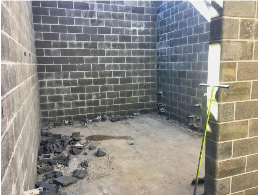
View of interior of Classroom Addition Bathroom.
