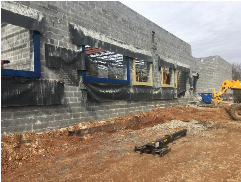
View of exterior of East face of Classroom Addition.
