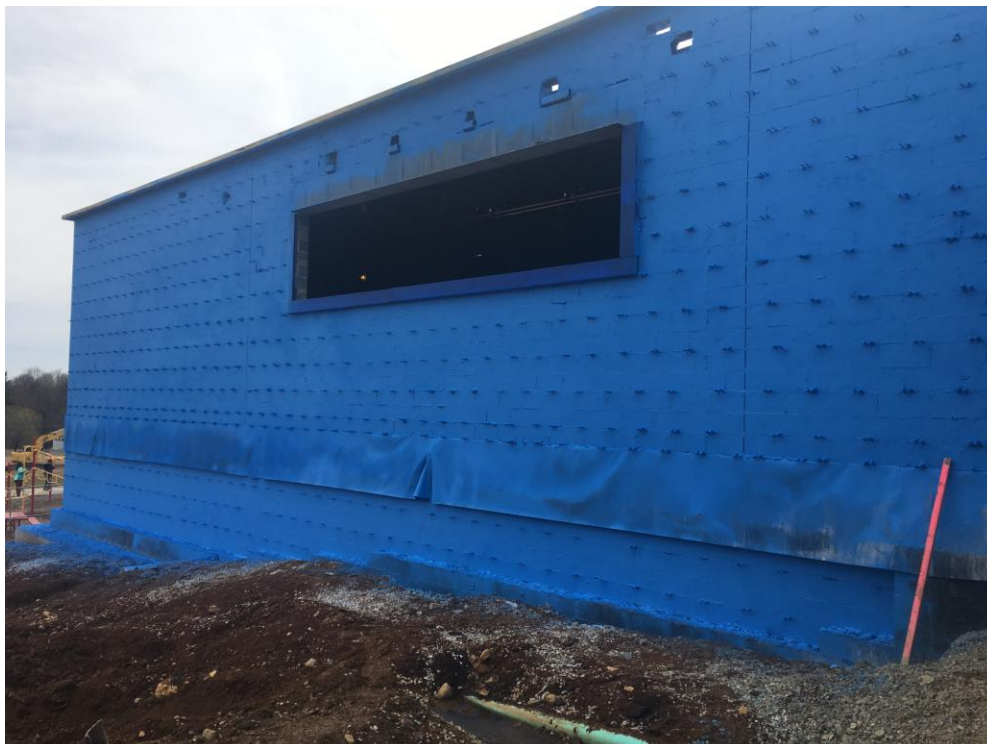
View of air infiltration barrier spray applied to Gym exterior walls.
