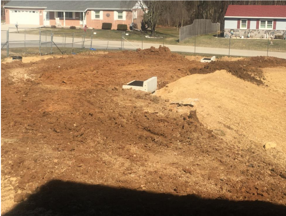
Topsoil being spread at Retention Ponds.
