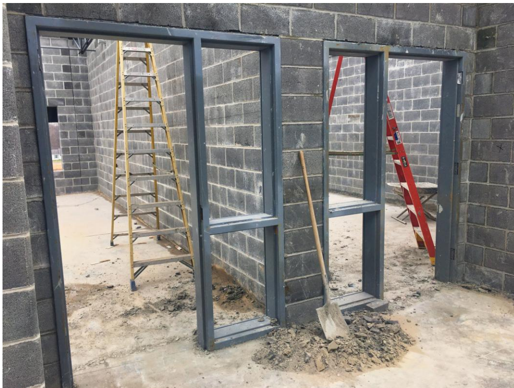
View of Classroom entrance doorbucks.
