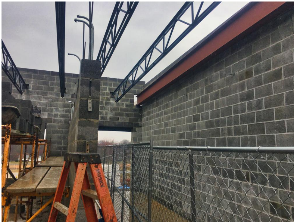
View of new corridor to playground facing East.
