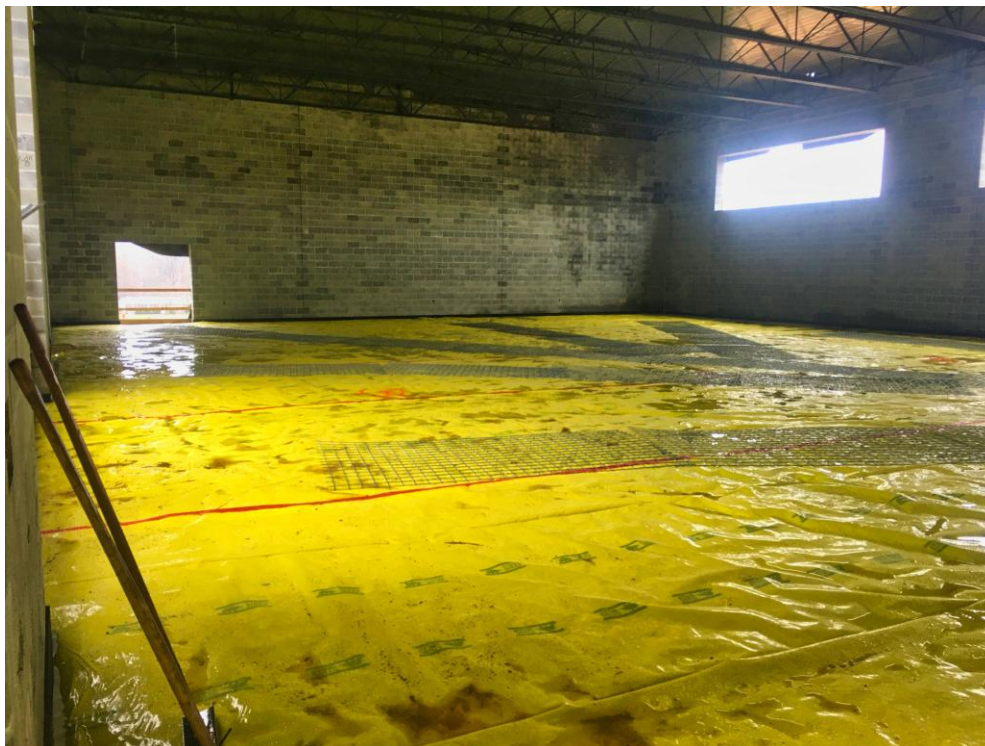
View of Gym ready to pour floor.
