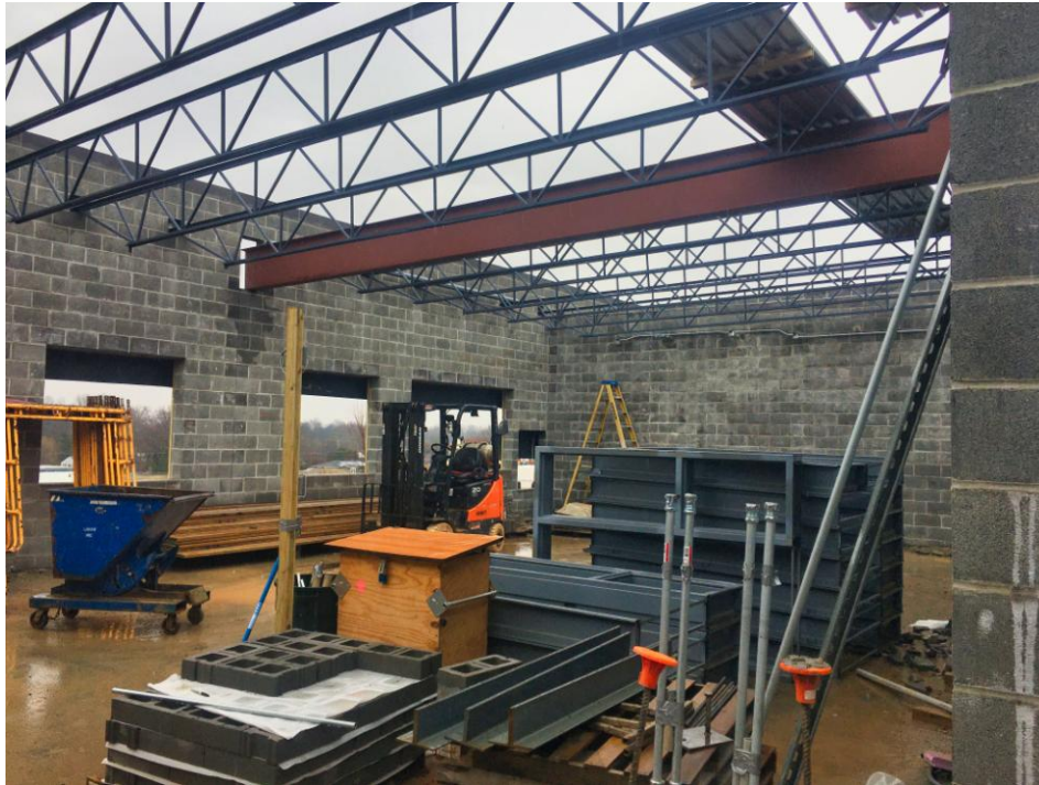
View of LGI Room showing support steel for moveable partition..
