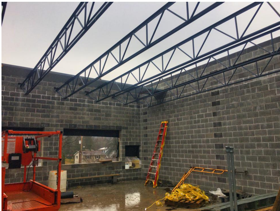
View of Classroom Addition facing East.
