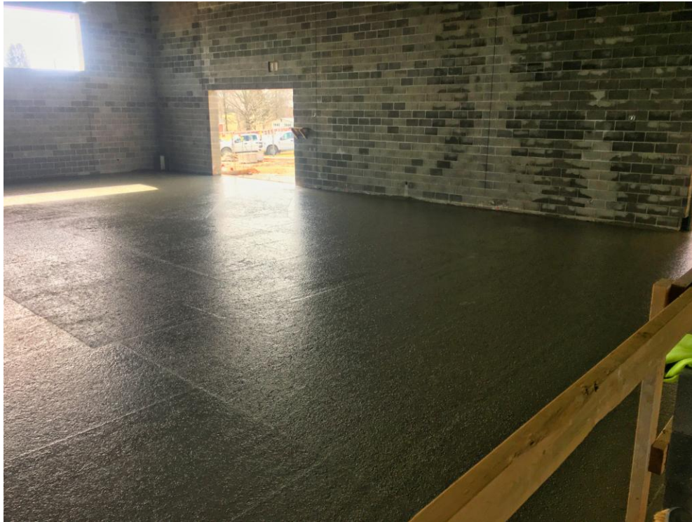
View of Gym floor facing Main Entrance Door, (West).
