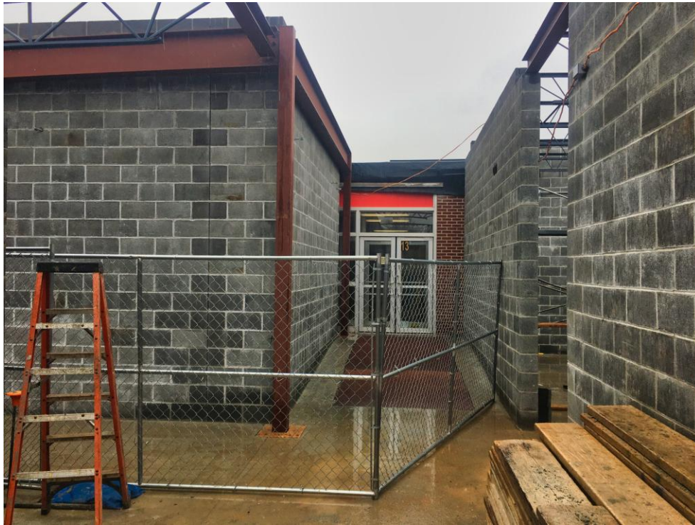
View of new corridor to playground facing existing building, (South).
