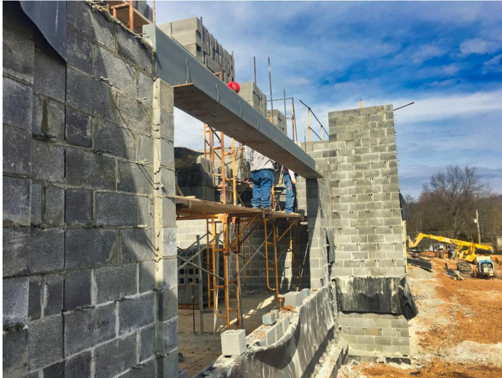
View along East wall of Classroom Addition showing steel lintel.
