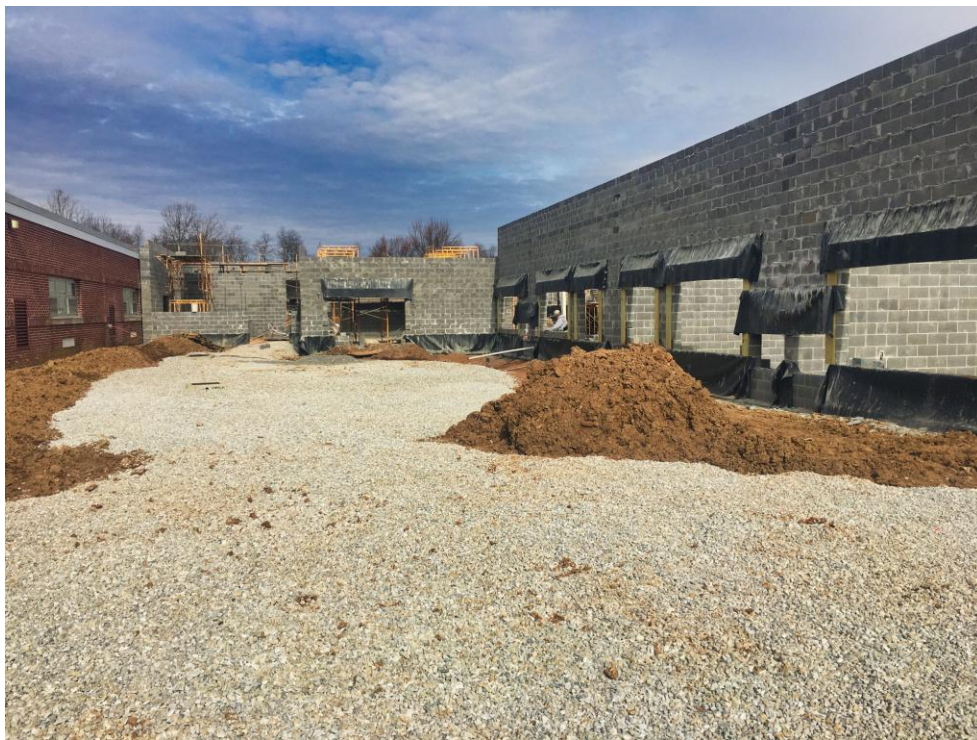
View of Courtyard between Existing Building and Classroom Addition..
