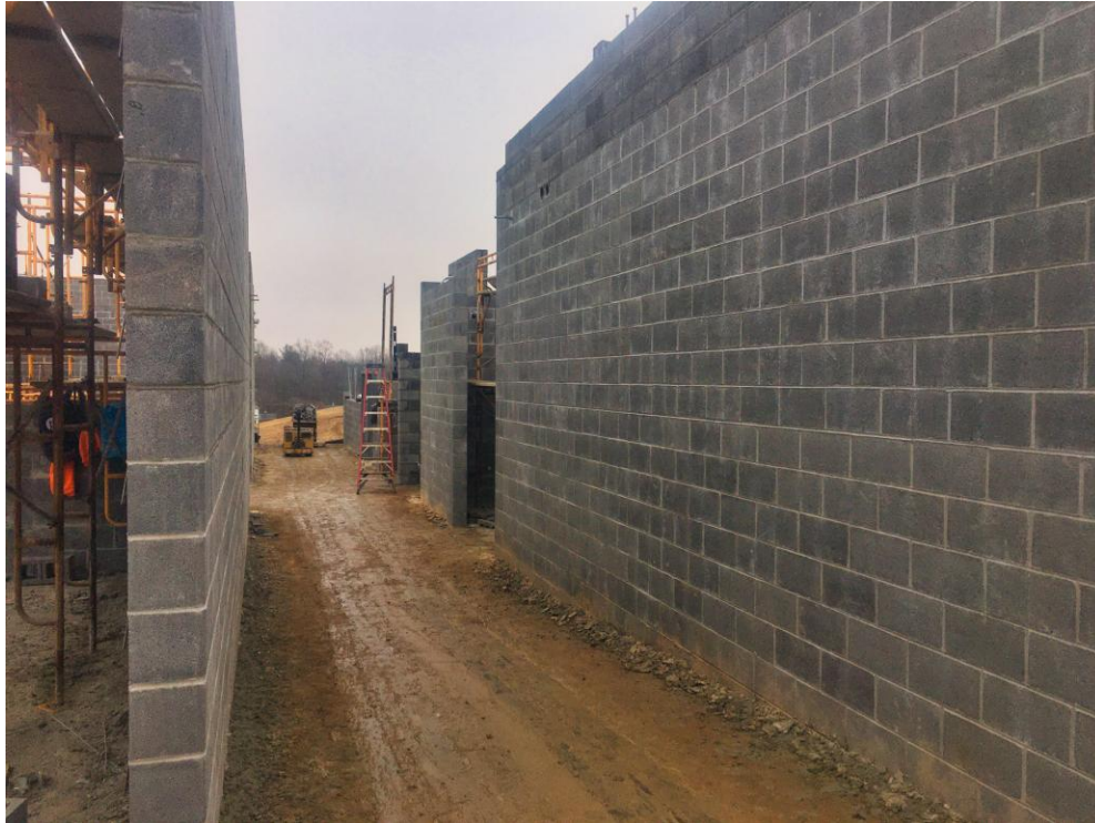
View of East/West corridor in Classroom Addition facing East.
