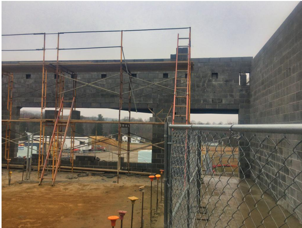
View of new corridor to Playground steps.
