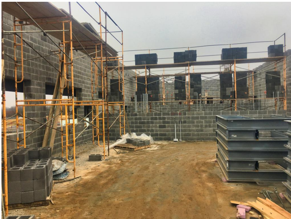
View of Classroom Addition interior facing South.
