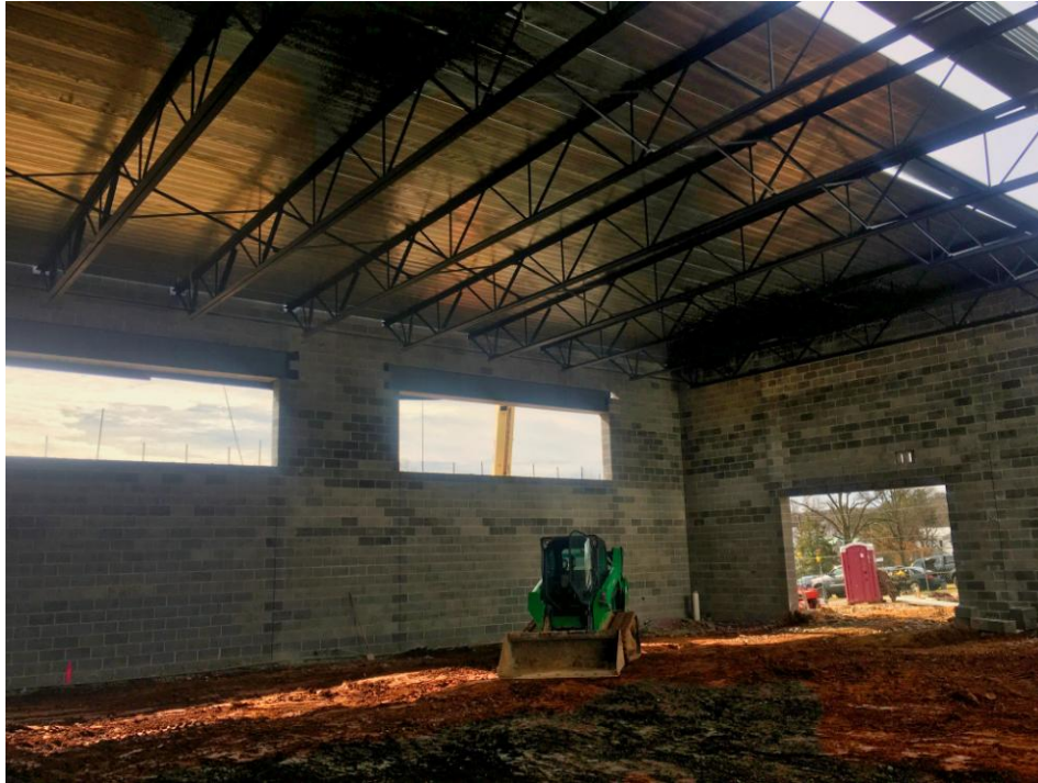
View of Gym facing entrance on West side.
