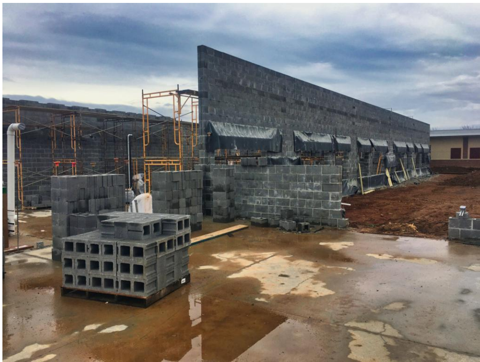
View of West exterior wall of Classroom Addition.
