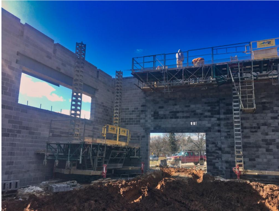
View of Gym interior facing West next day showing progress made.
