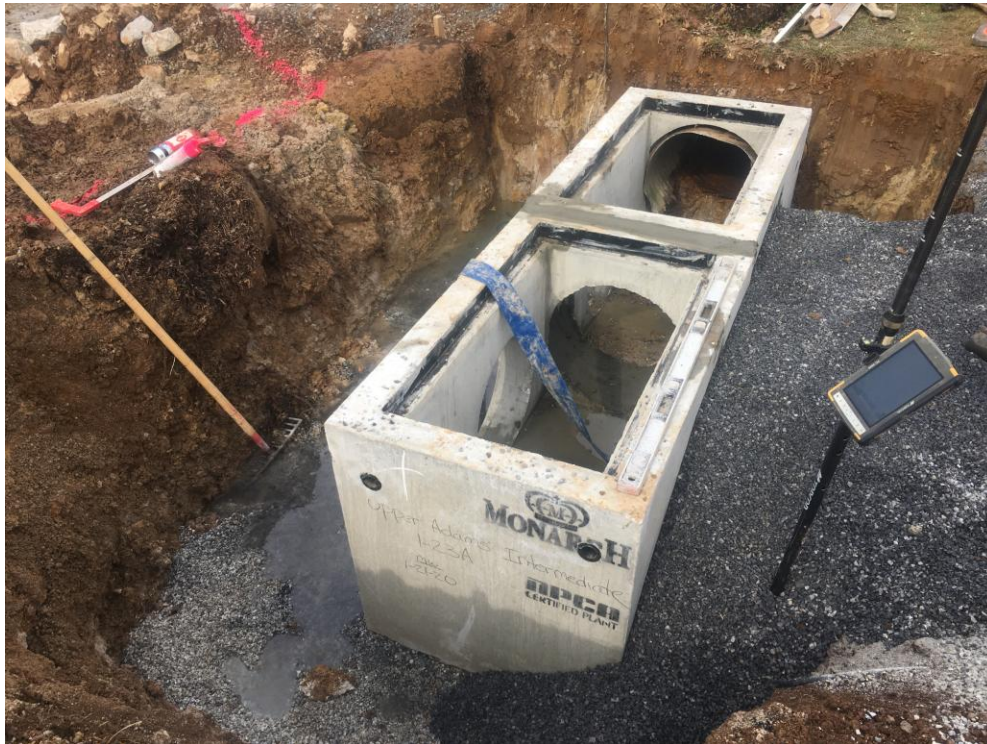
View of Inlet Basin being installed on Conewago St.
