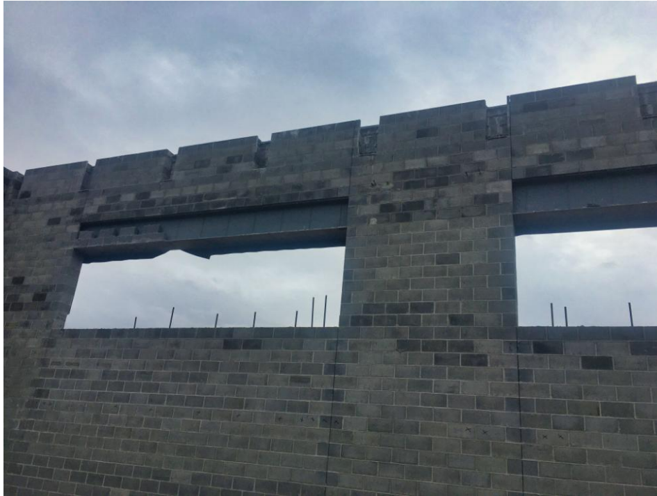
View of South wall of Gym Addition showing joist pockets.
