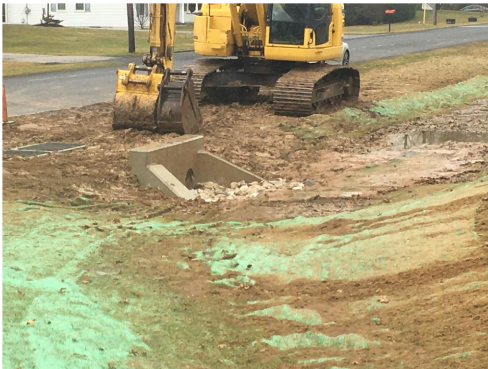
View of new Headwall for Conewago St Basin.
