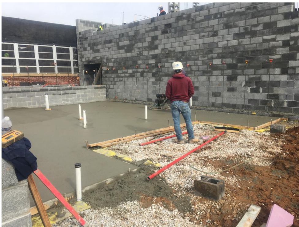
View of Gym Bathroom slab after pouring.
