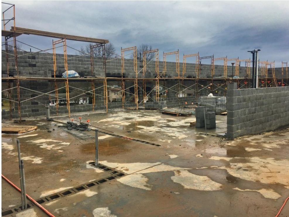
View of North wall of Classroom Addition.
