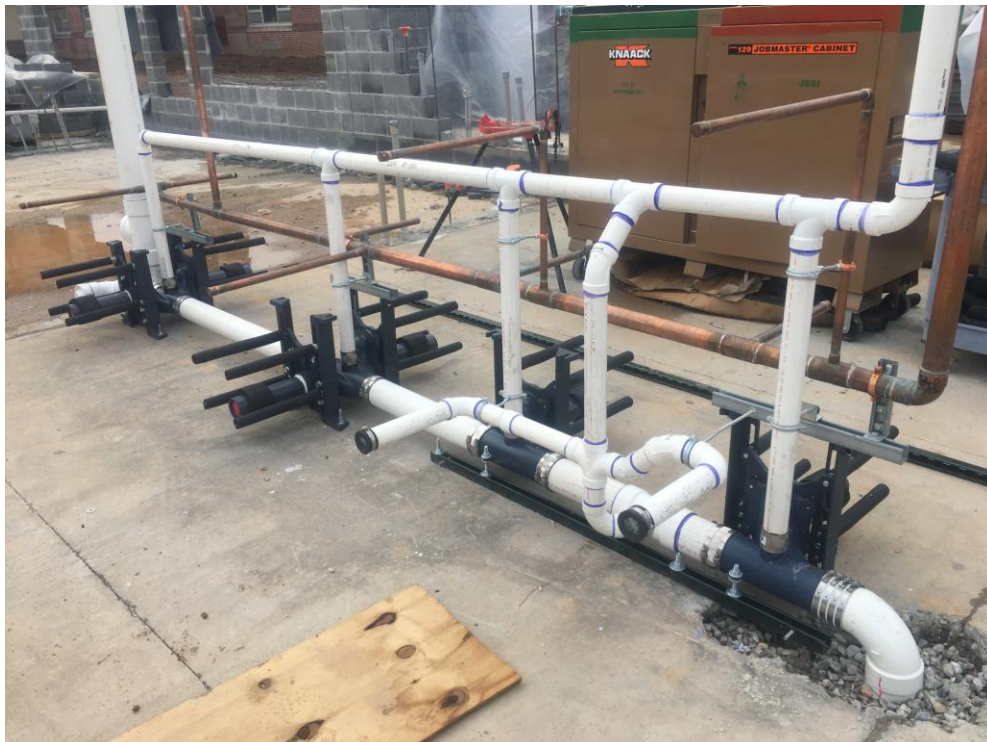
View of plumbing rough-in for Classroom Addition Bathroom.
