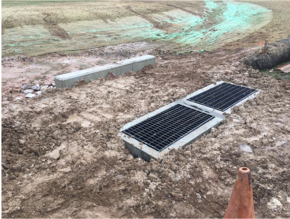
View of new Inlet Basin after installation and rough grading.
