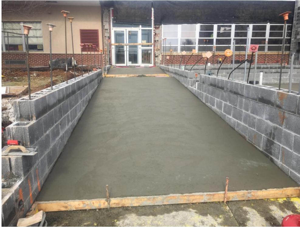
View of new corridor ramp at West end of Gym at existing building connection.
