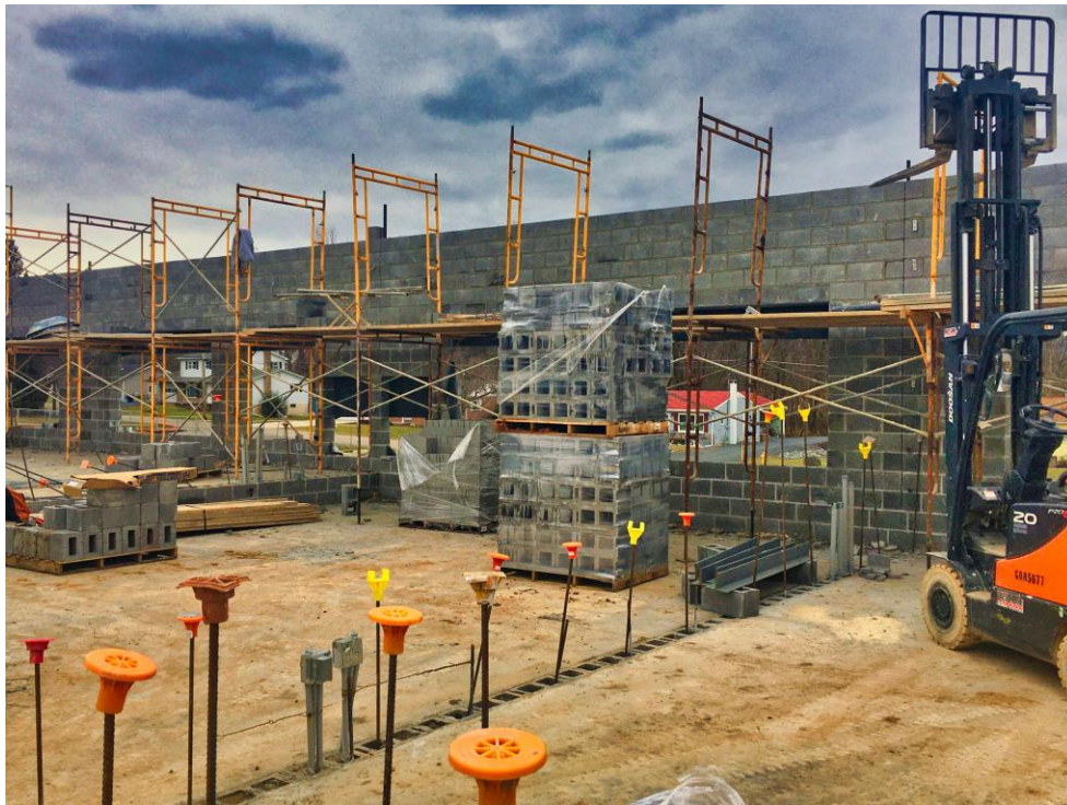
Interior view of east wall of Classroom Addition facing East.
