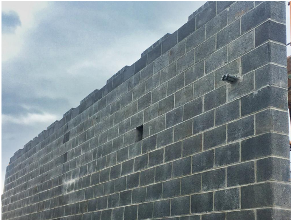
Interior view of corridor wall showing pipe penetrations and joist bearing plate notches.
