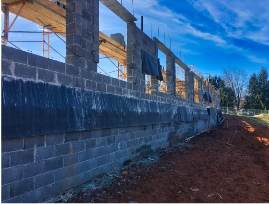
Exterior view of east wall of Classroom Addition facing North.
