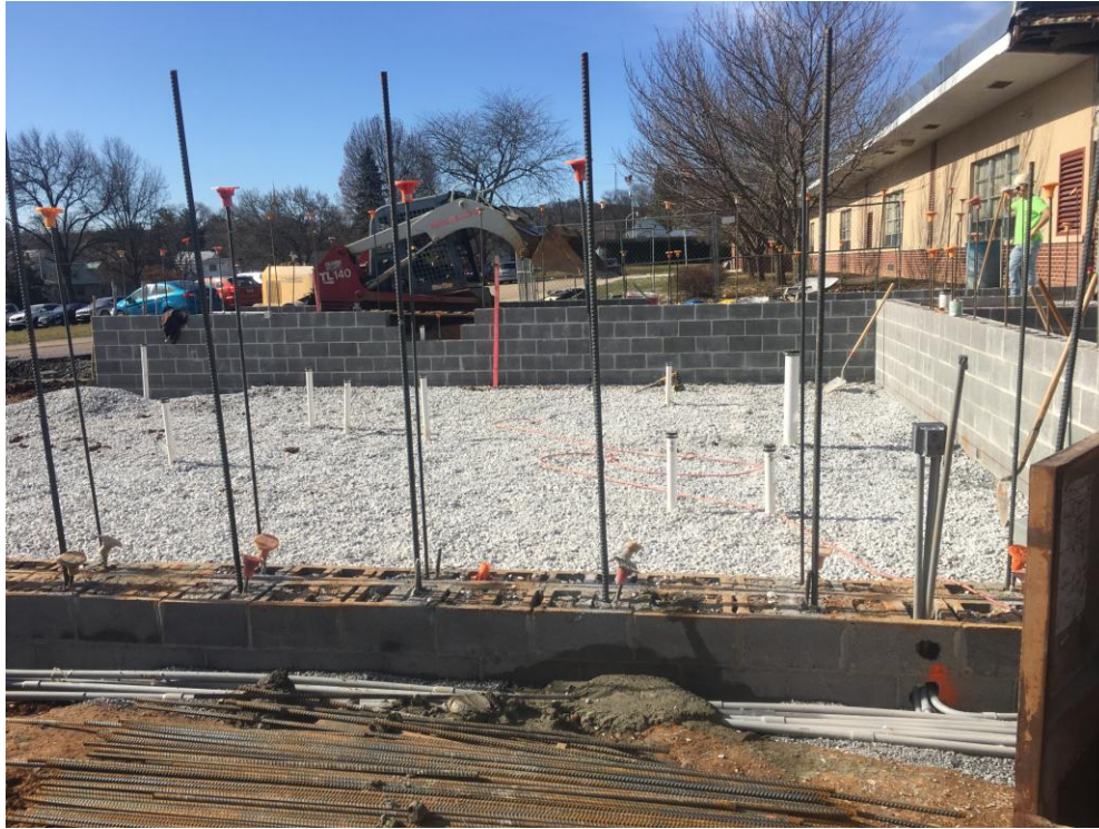
View of Gym Bathrooms being prepped for pouring of floor slab.
