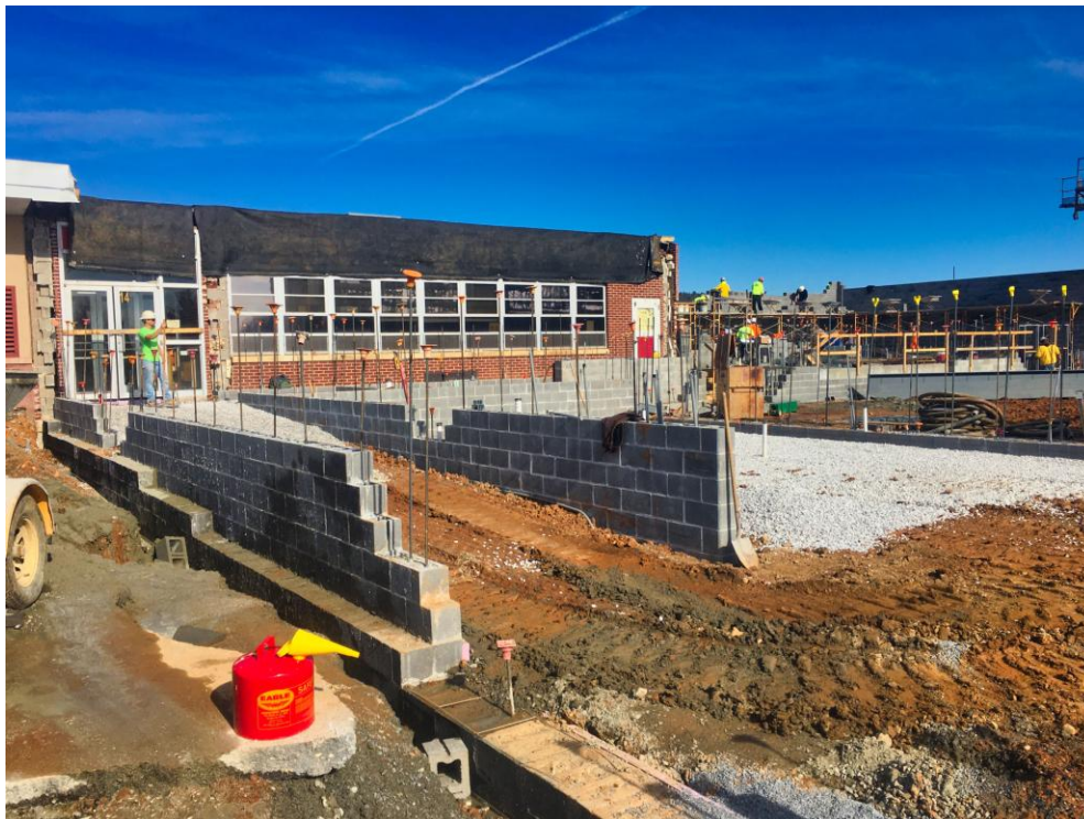
View of connection to Gym addition at southeast corner of existing building.
