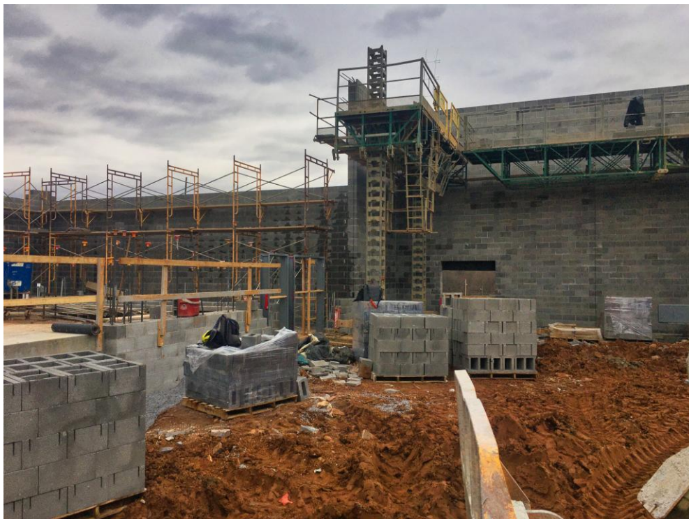
Interior view of east wall of Gym.
