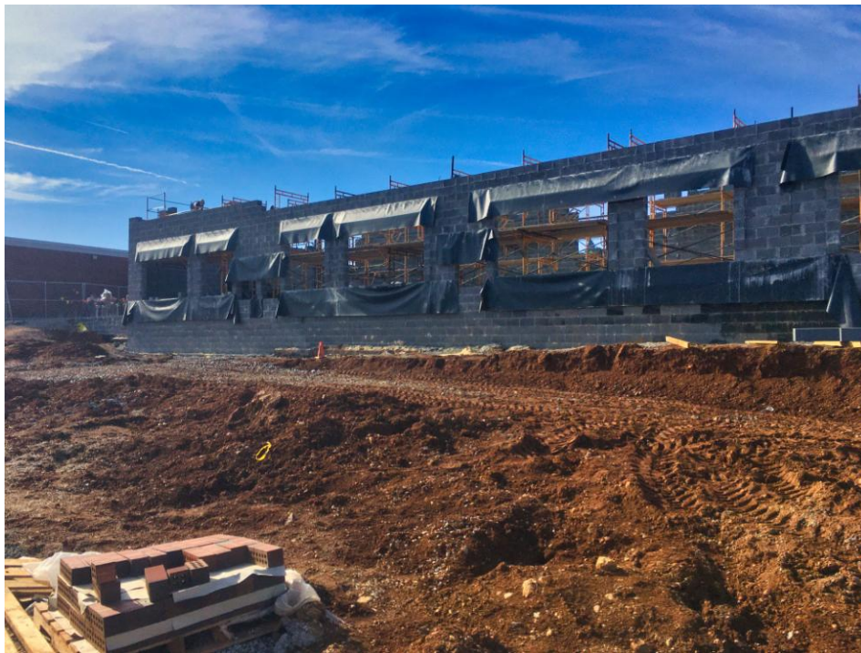
Exterior view of east wall of Classroom Addition.
