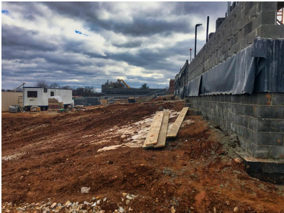
View of East side of Classroom Addition and North Gym wall.
