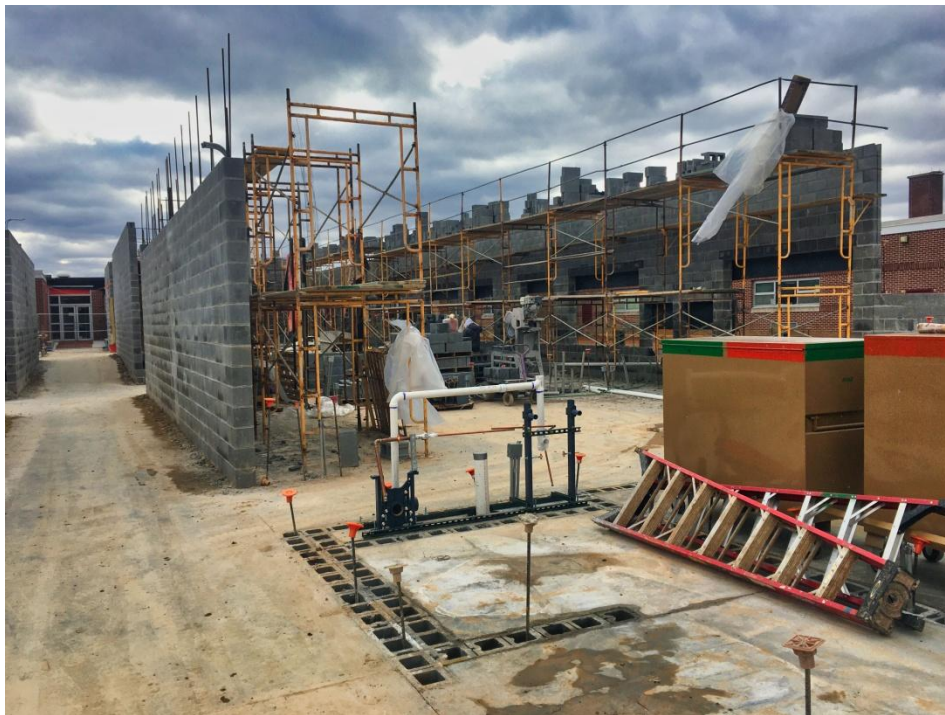
View of interior wall construction in Classroom Addition.
