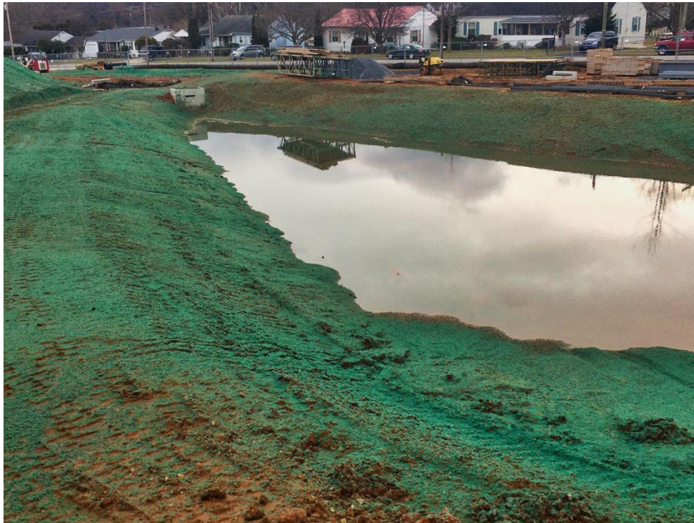
View of one of the Fohl Street Basins shown spray matting applied..
