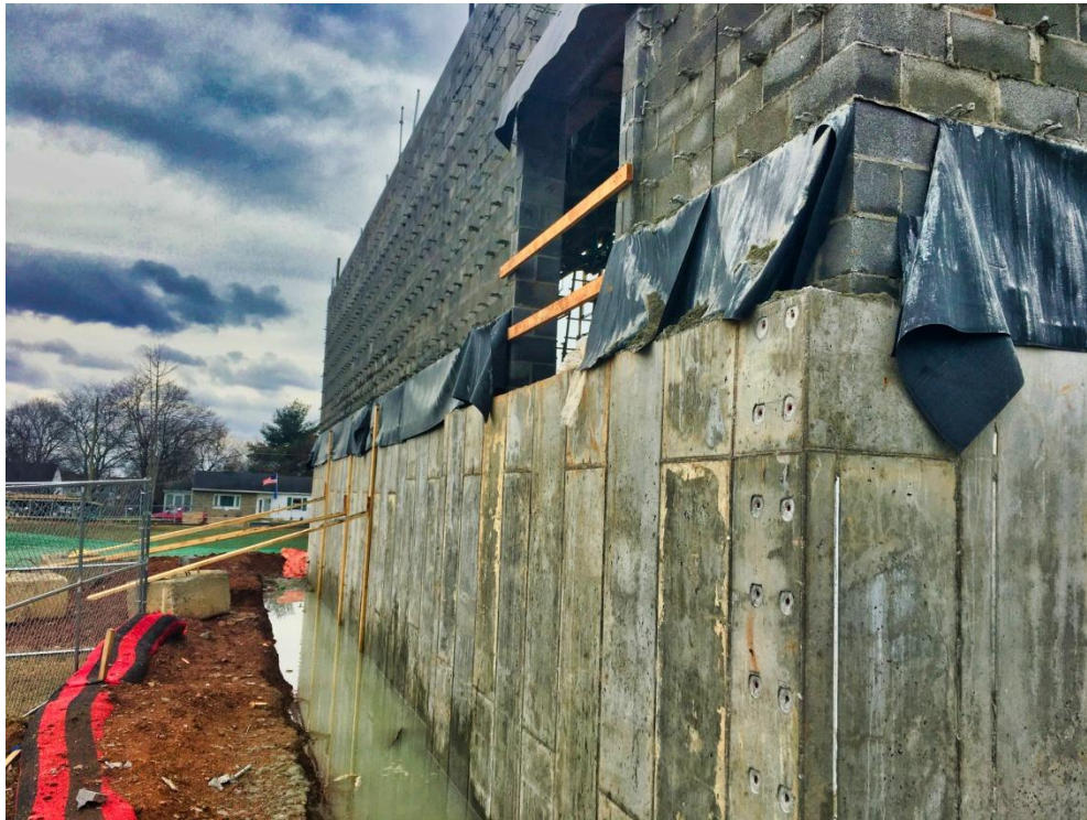
View of Gym retaining wall, East side.
