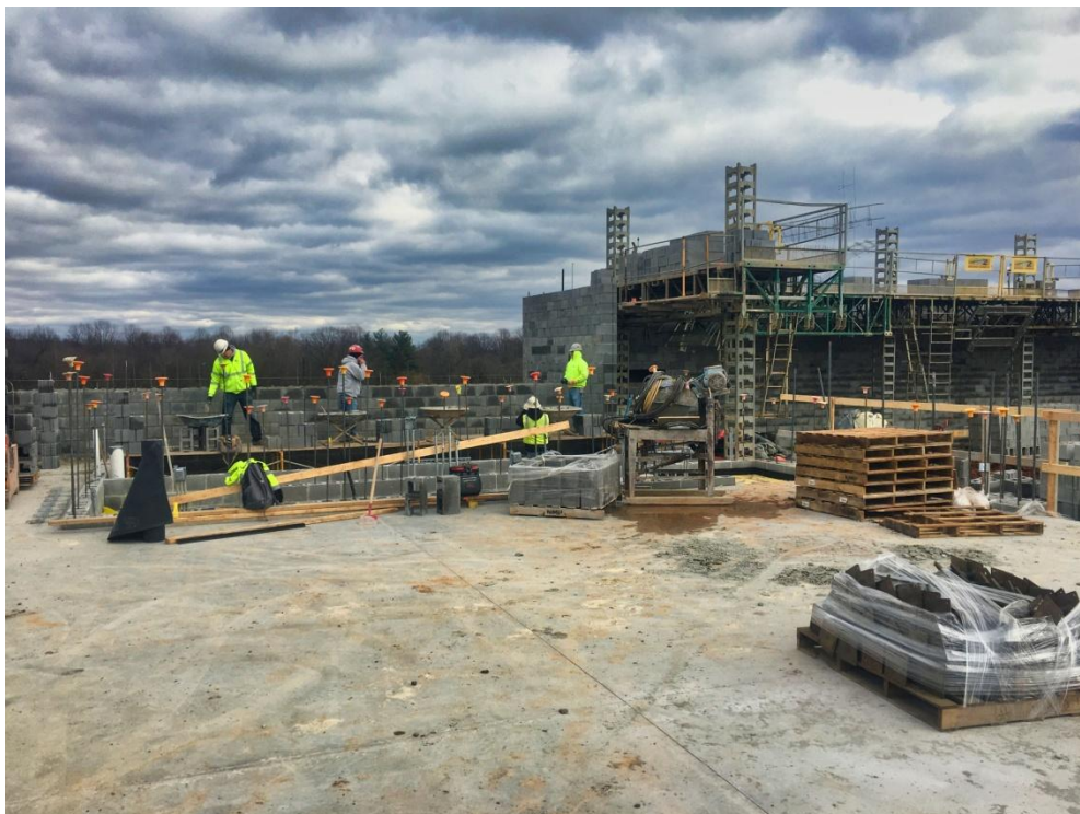
View of Gym walls being constructed..
