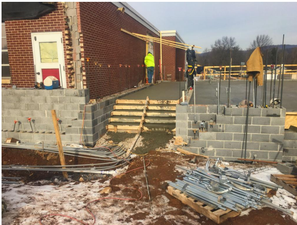
View of steps to Platform in Gym.
