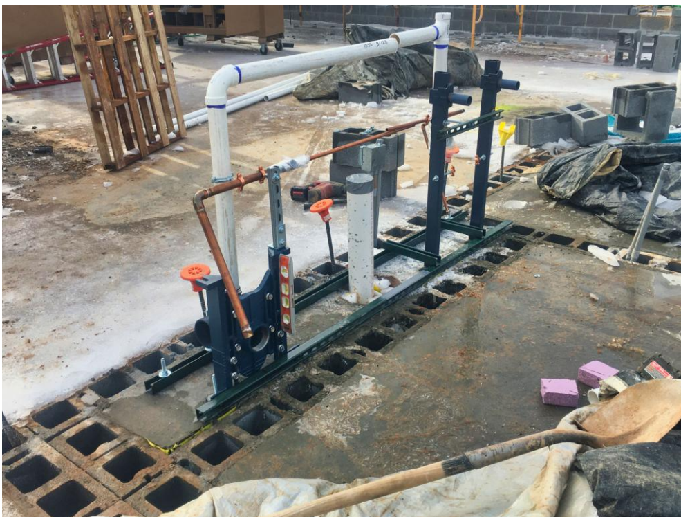
View of plumbing rough-ins in Classroom Addition Bathrooms.
