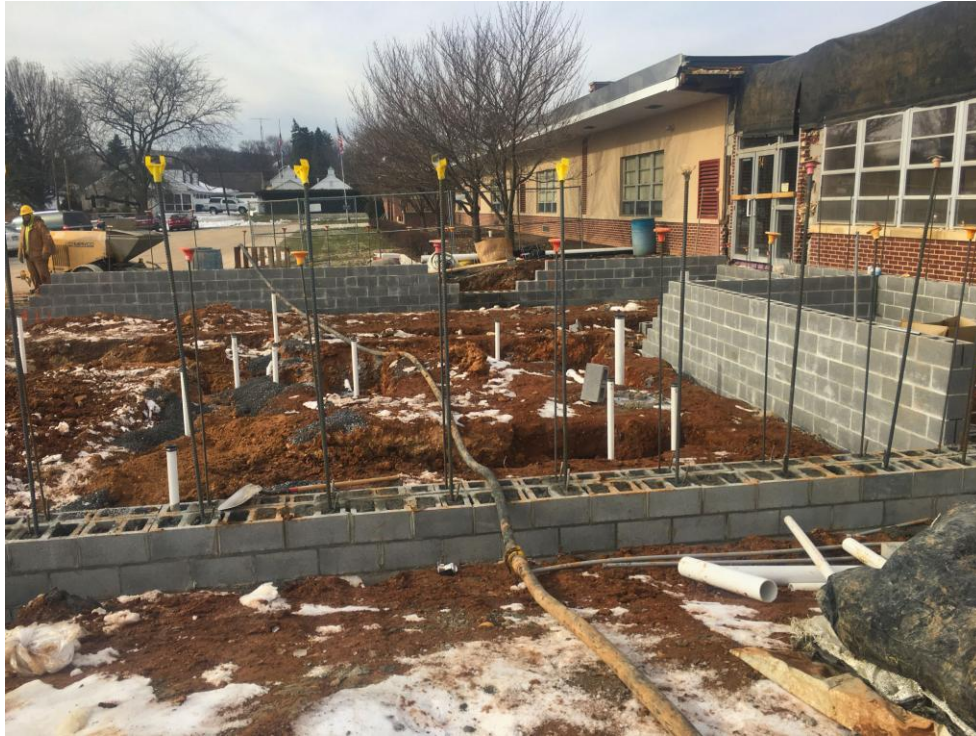
View of walls and plumbing rough-ins at Gym Bathrooms.
