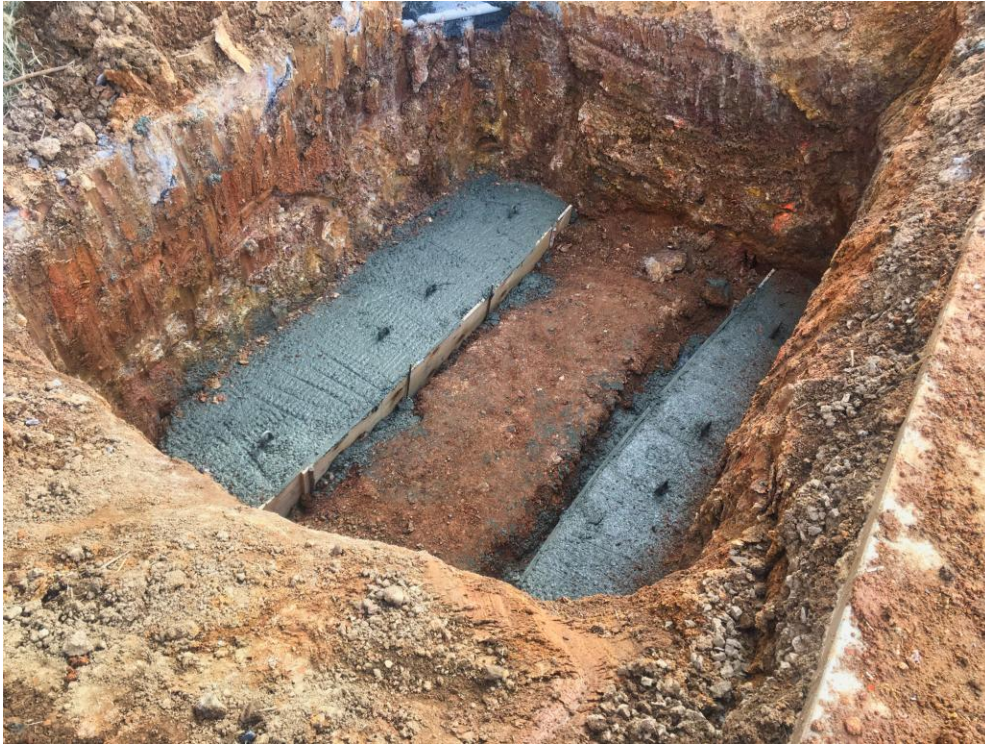
View of foundation for Grease Trap behind Kitchen.
