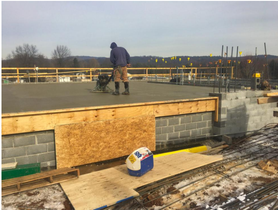
Platform slab being finished in Gym.
