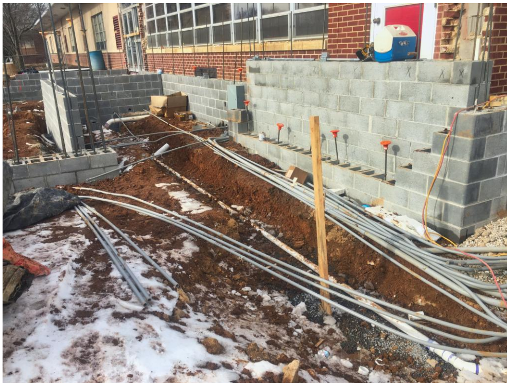
View of under slab electrical rough-ins in Gym Addition.
