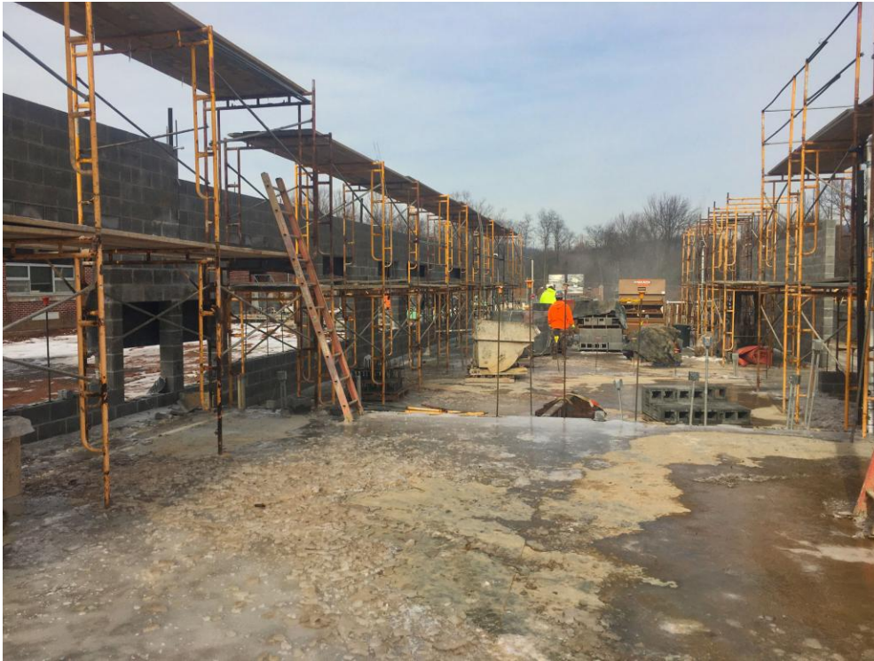
View of walls being erected in Classroom Addition.
