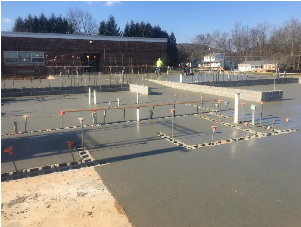
Second half of Classroom Addition slab being finished.
