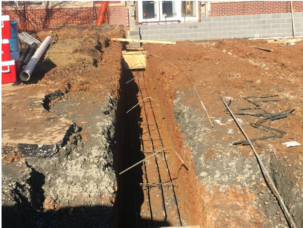
Final Exterior Gym footers being rebarred.
