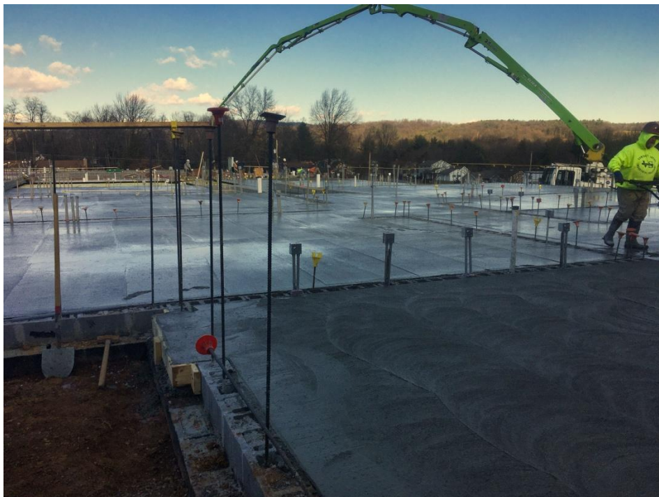
North half of Classroom Addition slab being poured.
