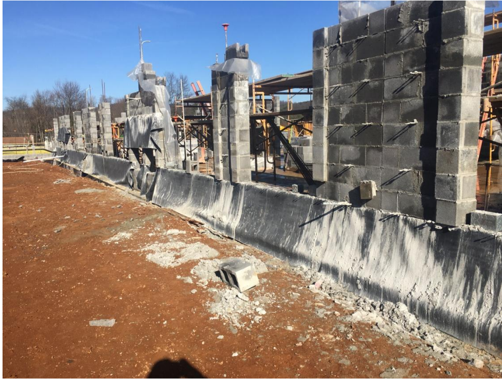
Exterior wall at Classroom Addition.
