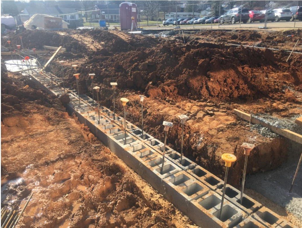
Foundation blocks being laid on Gym footers.
