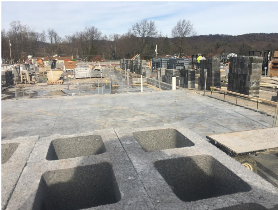
Block being staged on new floor in Classroom Addition.
