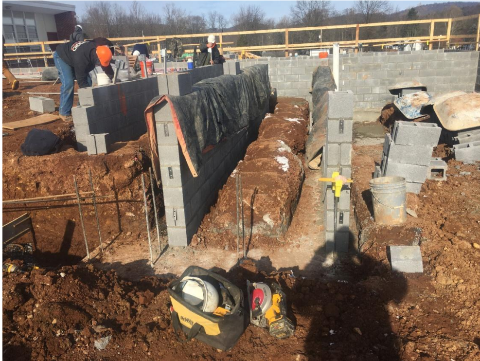
Block being laid for Gym Platform ramp.
