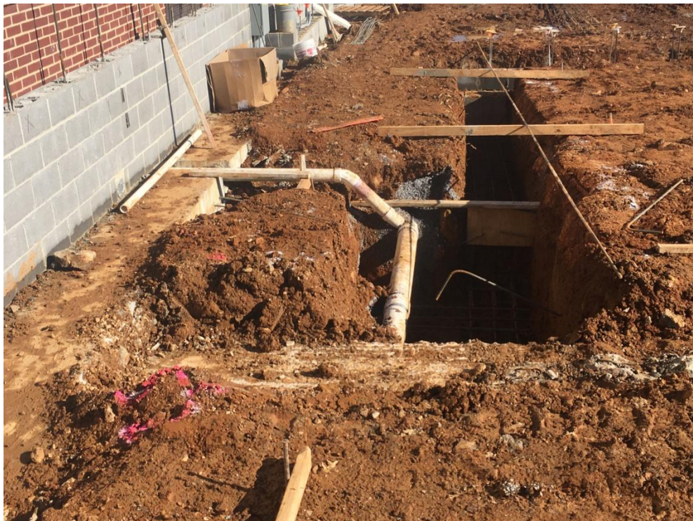
Plumbing rough-ins being installed in Gym area.
