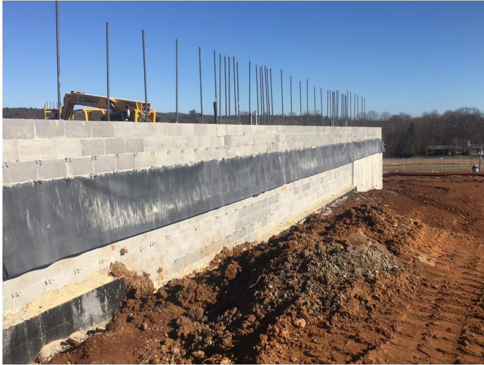
Block being laid at exterior Gym retaining wall.
