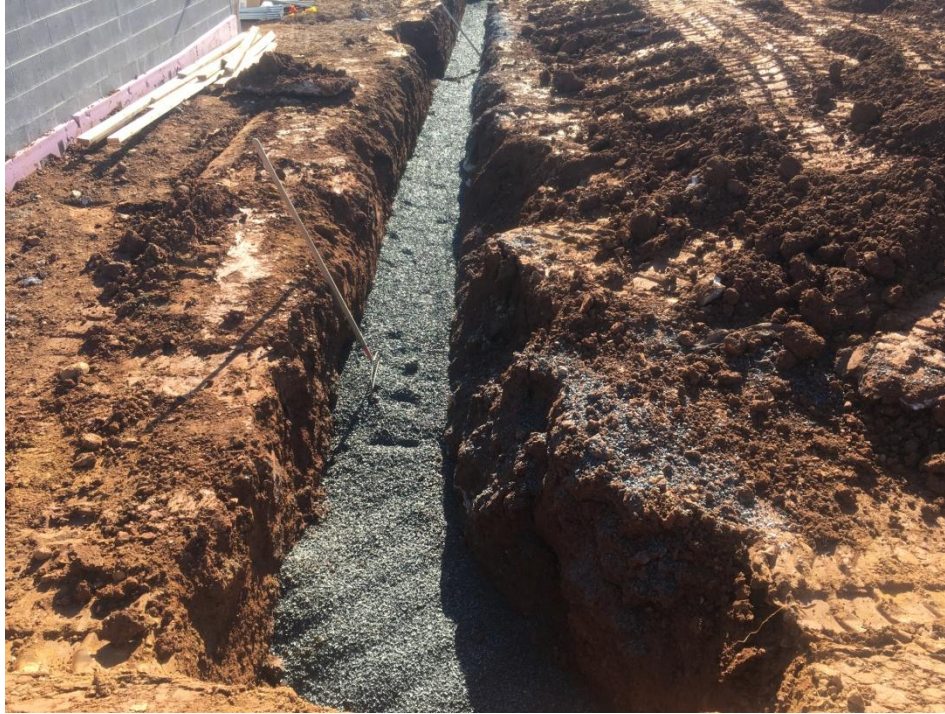
Trench stoned for footer pour at Gym.
