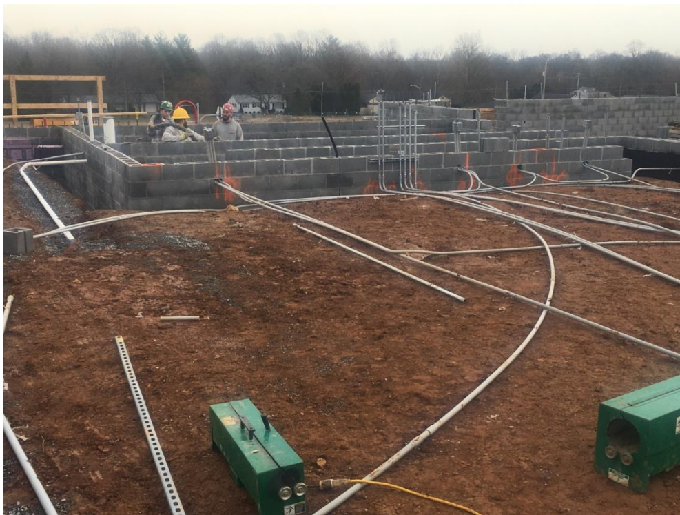
Electrical rough-ins being started in Gym.
