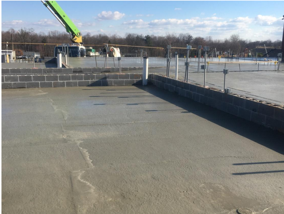
View of new slab after pour, prior to finishing.
