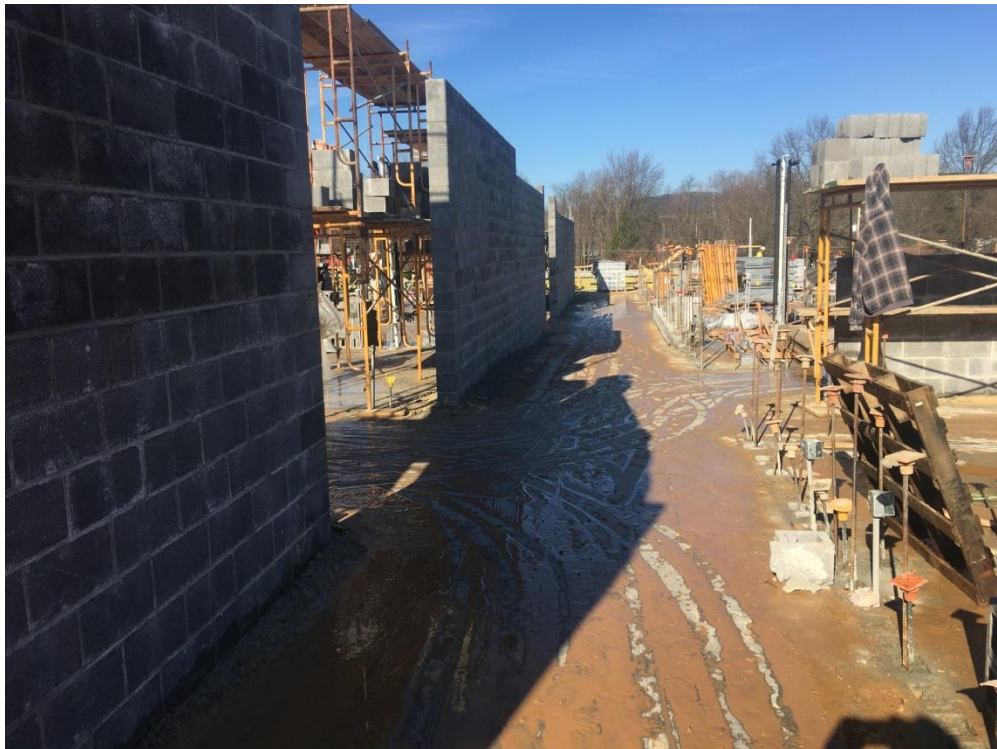
Interior corridor wall at Classroom Addition.
