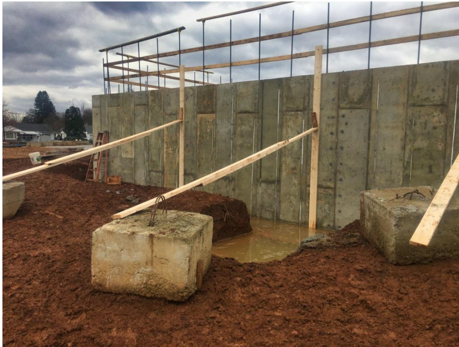
View of Gym foundation wall.
