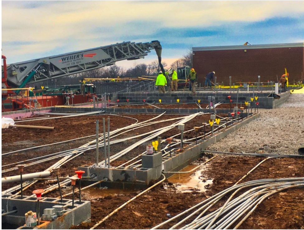
Classroom Addition slab being stoned prior to pouring floor.
