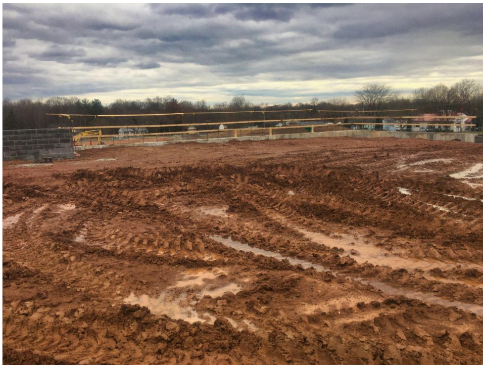
Gym area being backfilled.
