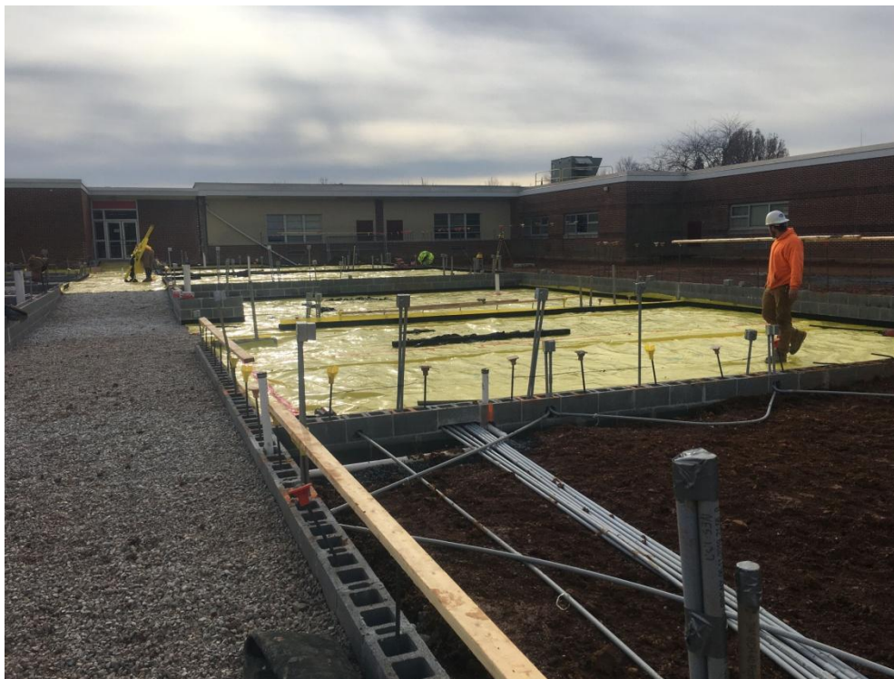
Vapor Barrier being applied.
