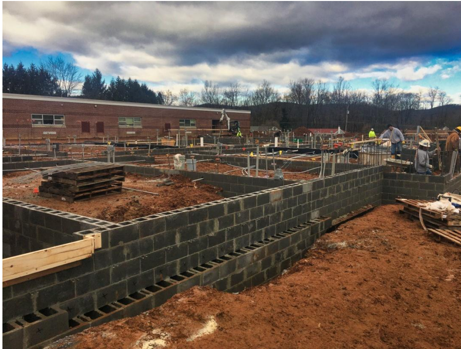
View of Classroom Addition with rough-in work being done.
