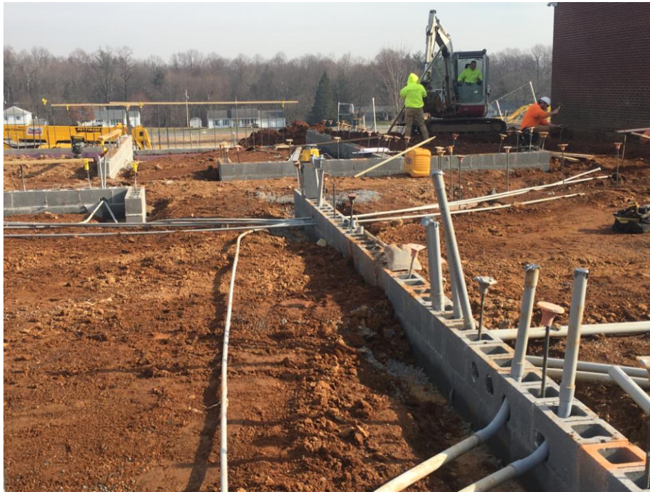
Classroom electrical being roughed in.
