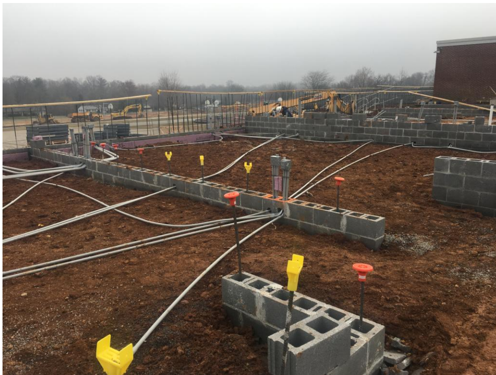
Electrical rough-in proceeding.
