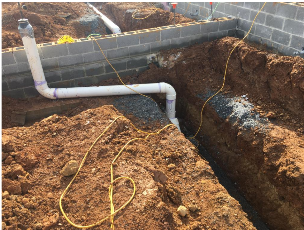
Connection from room to main sewer line.
