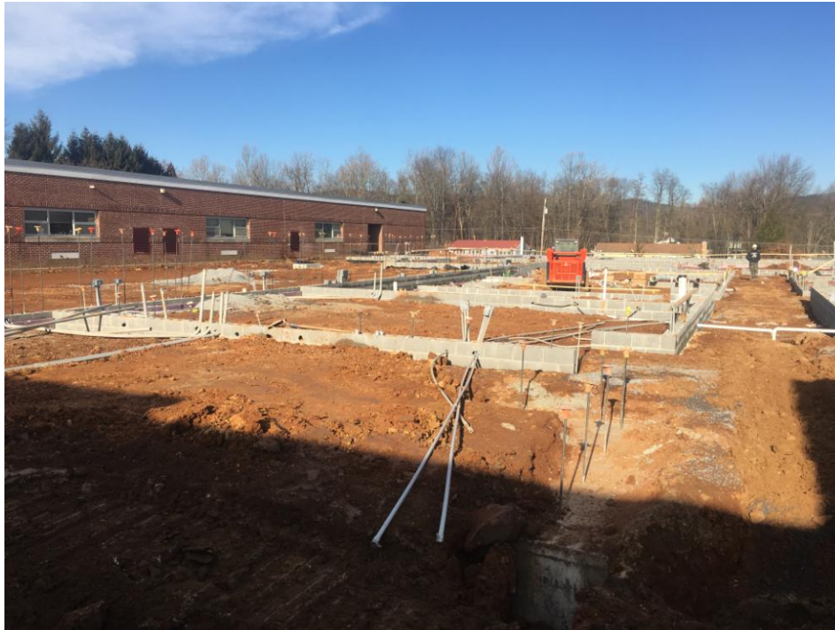
View of Classroom Addition with electrical rough-ins starting.
