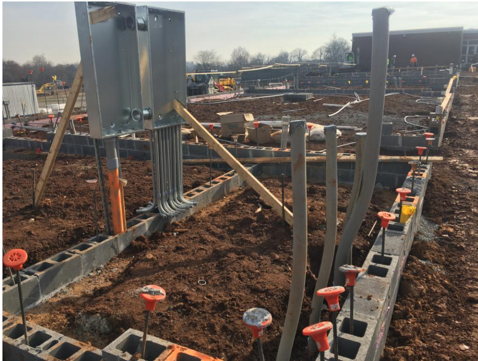
Classroom Addition Data/Electrical closet being roughed in.
