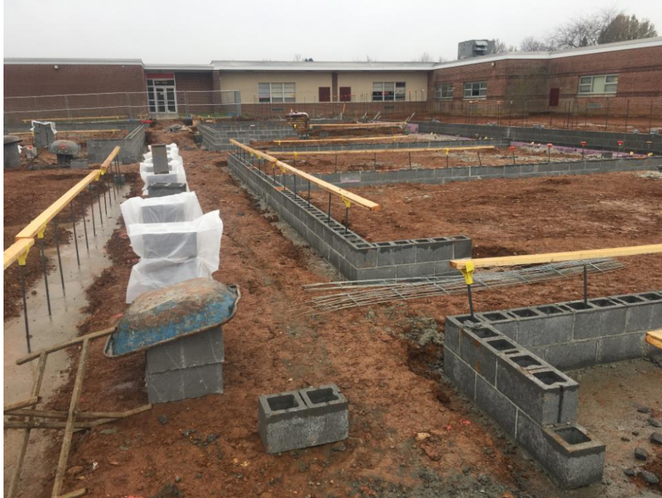
Classroom Addition walls being set.
