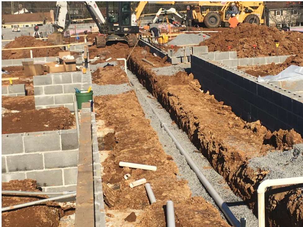
View of waste lines being installed under new corridor.
