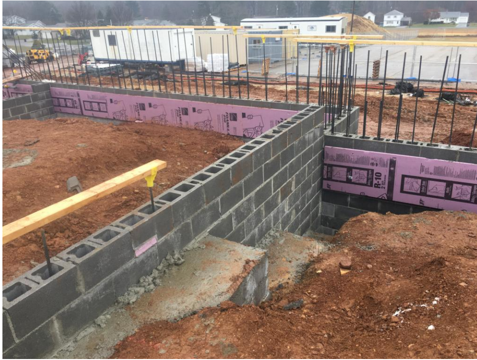
Classroom Addition South wall showing step footer.
