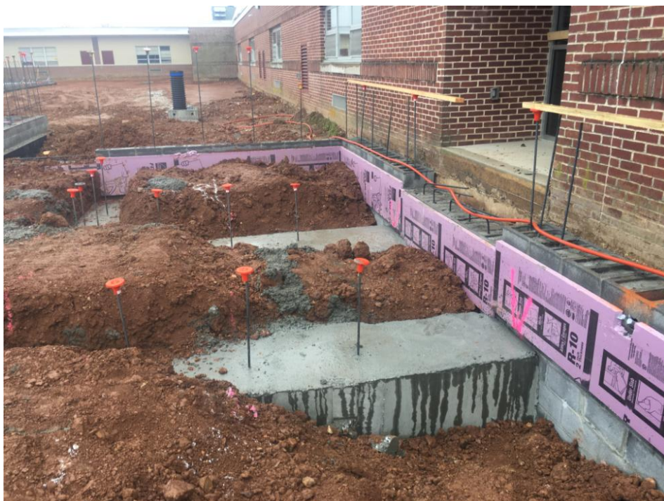
View of footers where new corridor attaches to existing building at Classroom Addition.
