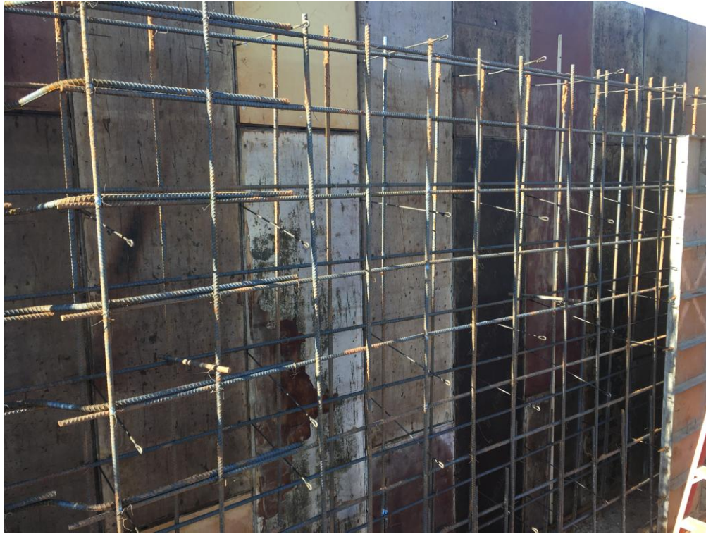
Close-up of rebar work at Gym retaining wall.
