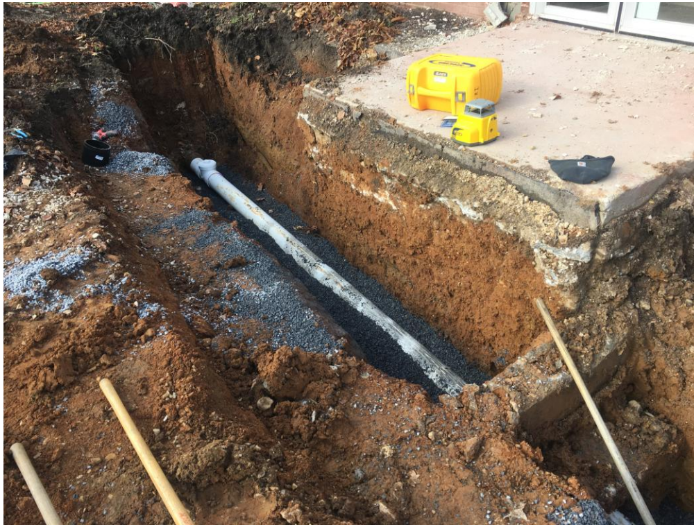
New piping being installed for room drain lines.
