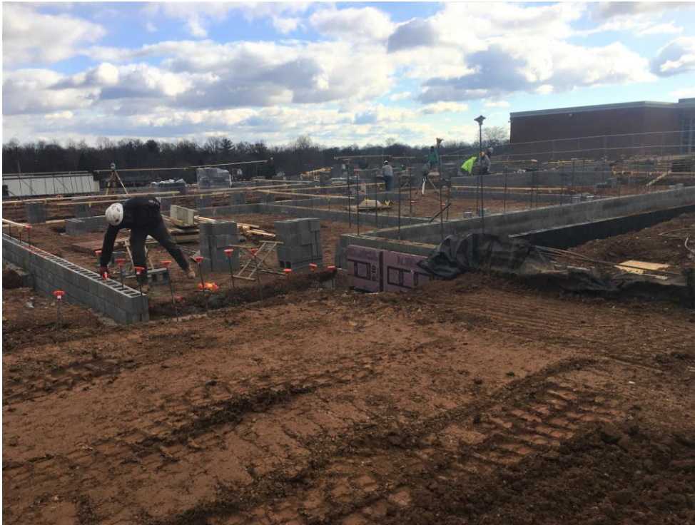
Interior walls being laid in Classroom Addition.
