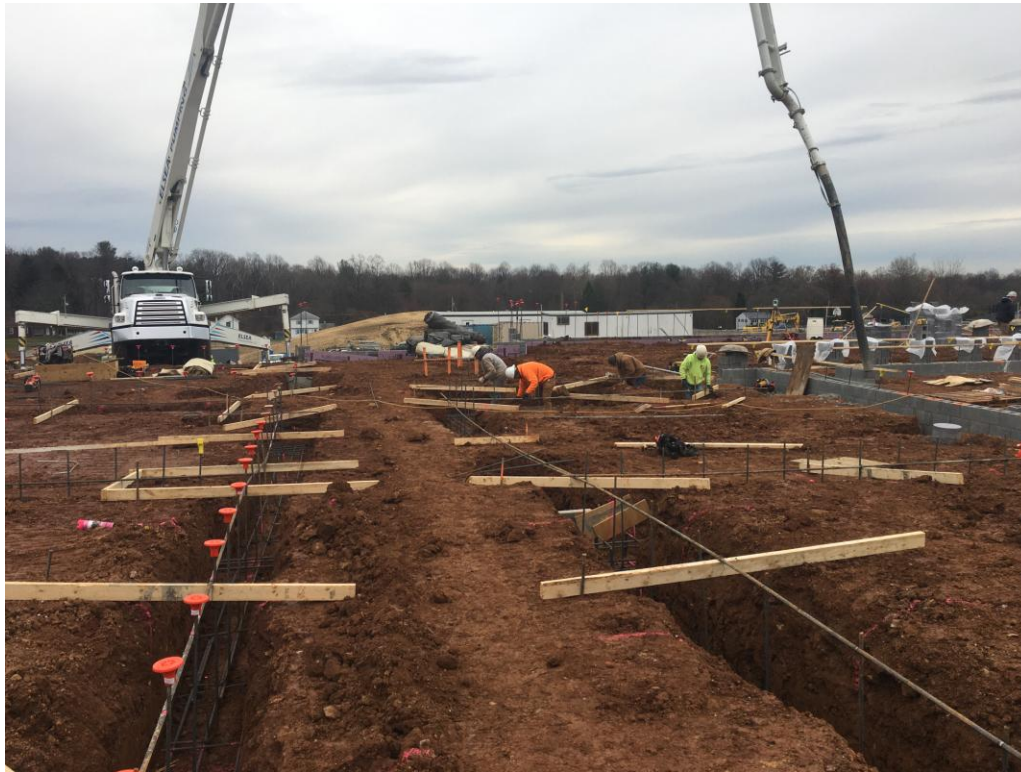
View of concrete being pumped into interior footers at Classroom Addition.
