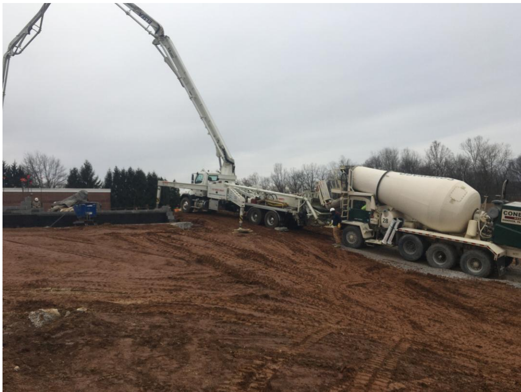
Second view of concrete pumping operation.
