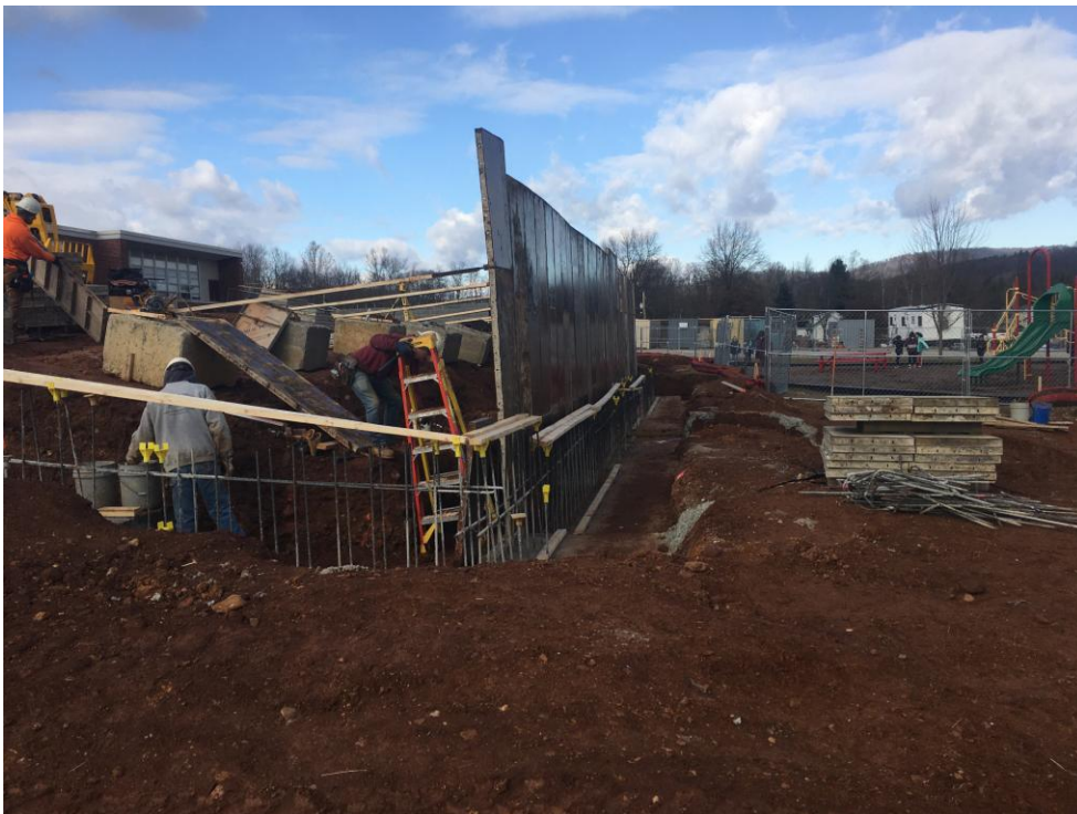
Forms being erected for Gym wall.
