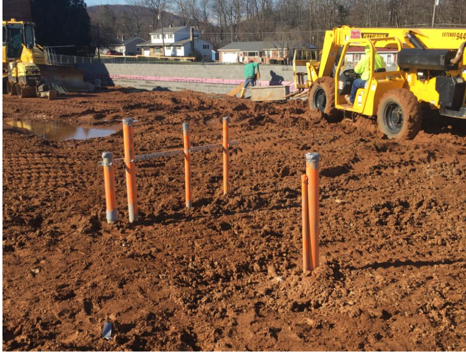
Conduits in place for Classroom Addition Electrical Room..
