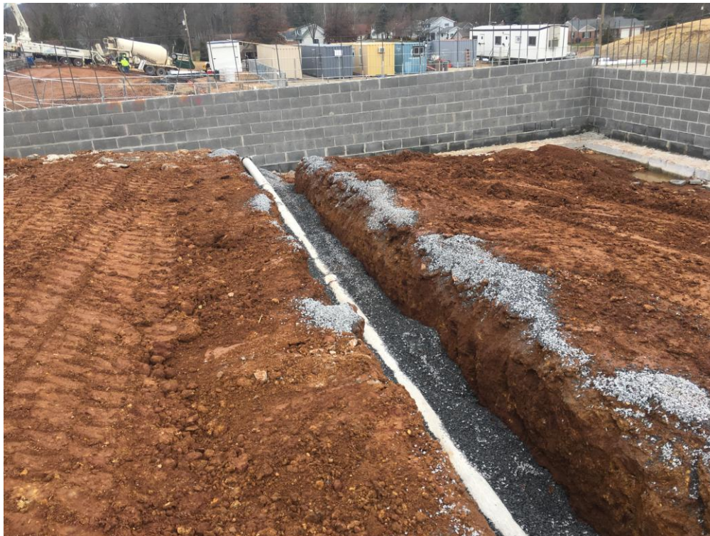
New Roof Drain line exiting through gym footer wall.
