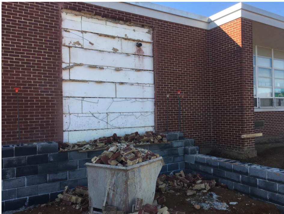
Preparation for opening into existing building for new Gym hall connection.
