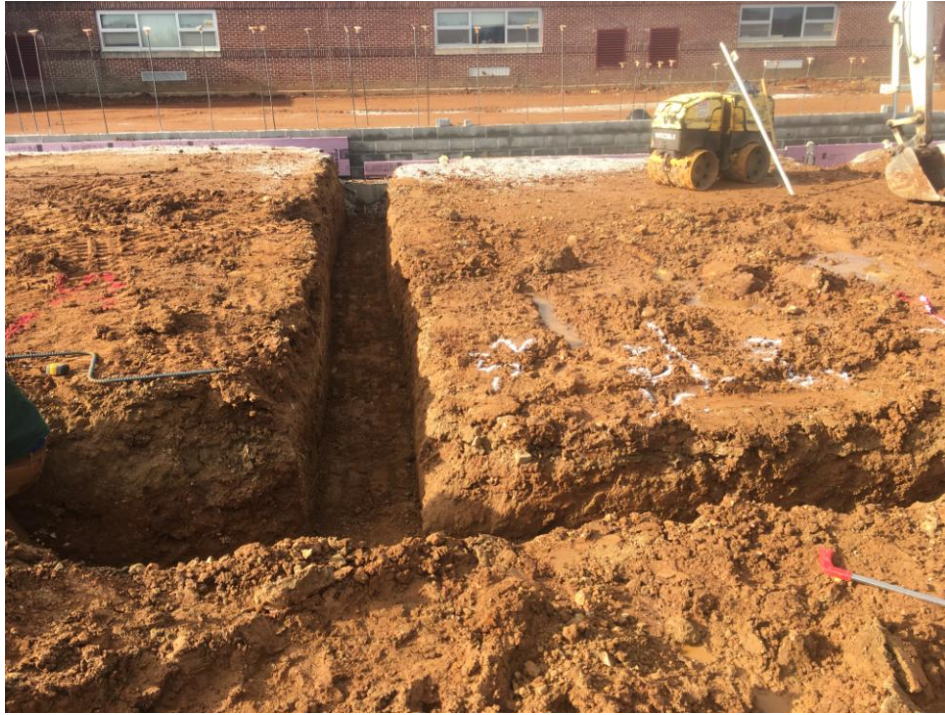
Trenching for interior footers in classroom addition.
