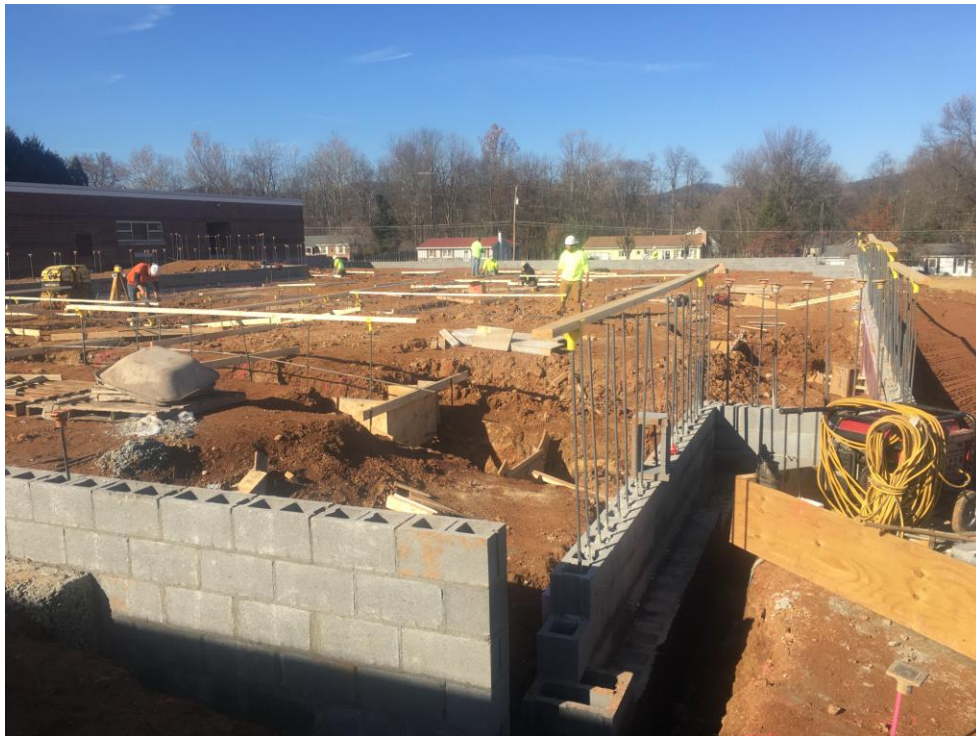
View of work on interior footers for classroom addition, viewed from new gym side of site.
