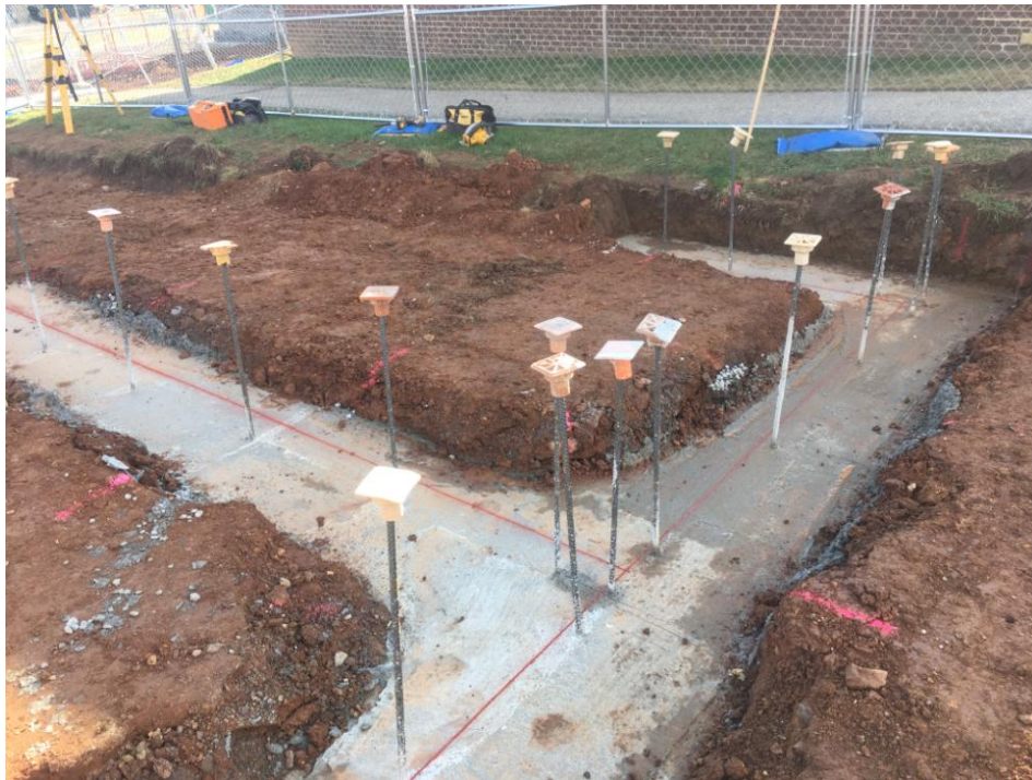
Start of interior footers for classroom addition.
