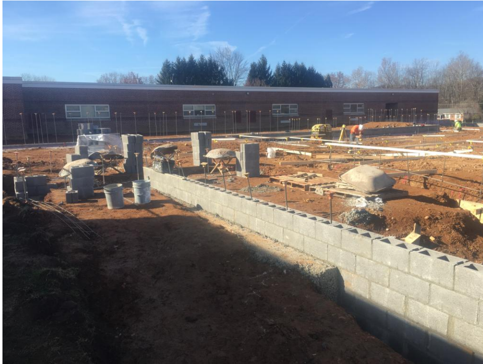
View of interior footers from building pad of classroom addition.
