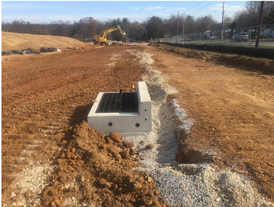
New catch basin in swale along Fohl St.
