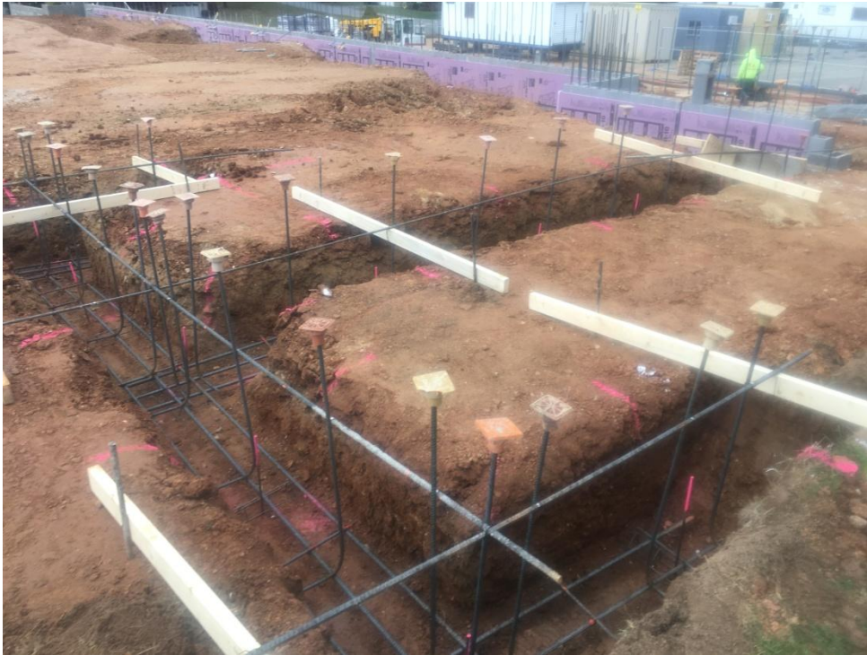
Interior footers for classroom walls being started.
