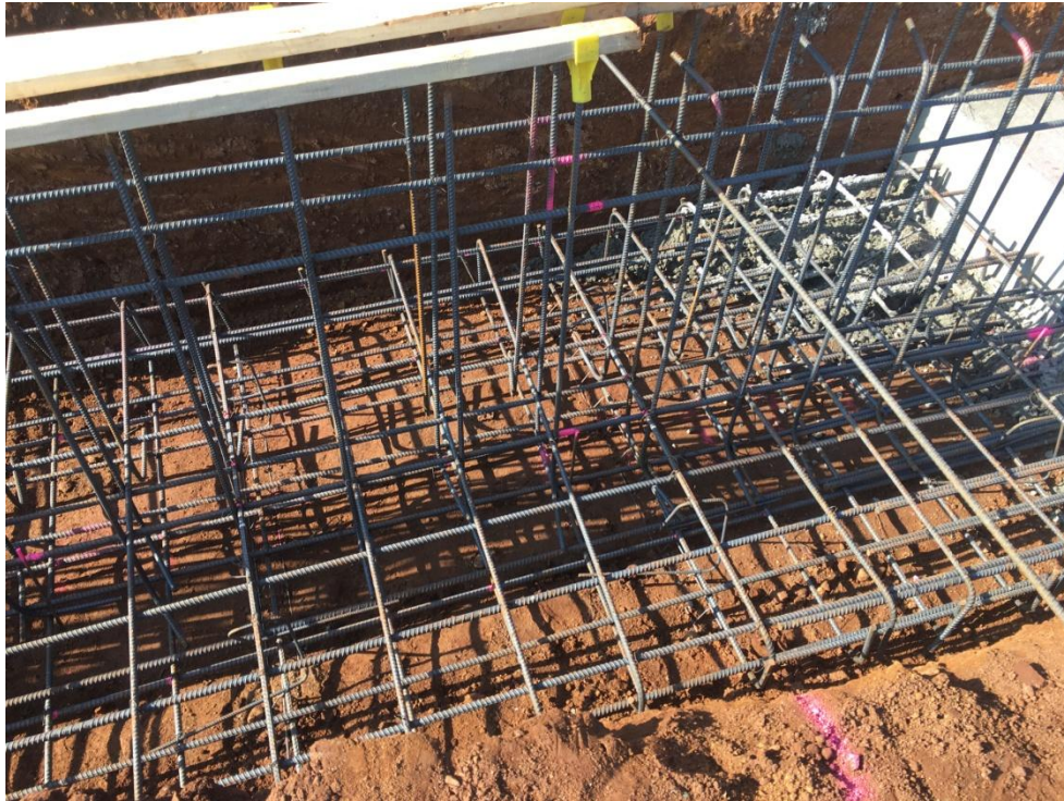
Detail of how rebar is tied for Gym footer on the Conewago St side of the building.
