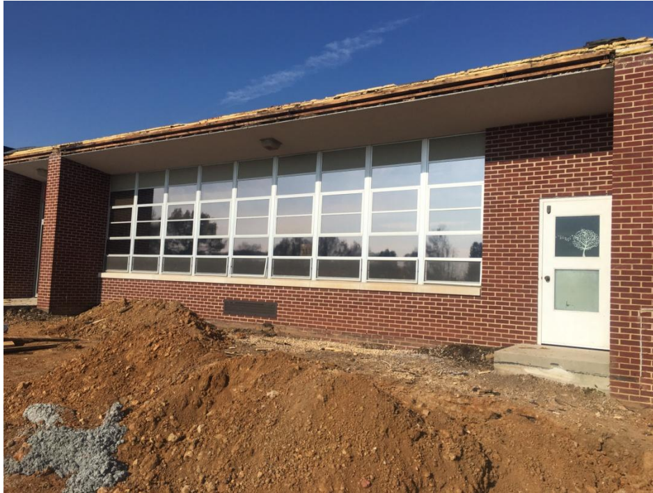
Overhang being removed at front by Band Room for new building connection.
