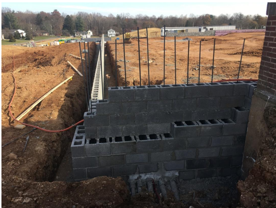
Completed foundation walls for new classroom addition at connection to the existing building.
