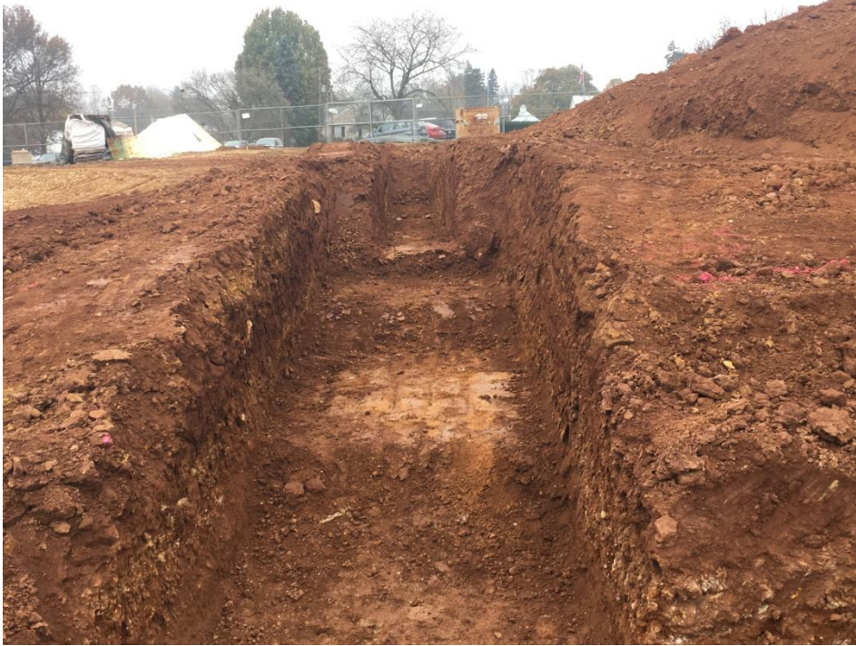
Footer trench for Gym on Fohl St side of building.
