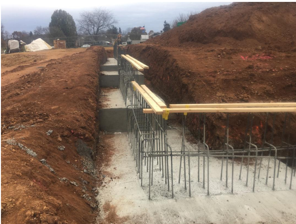
Same trench after rebarring and concrete pour.
