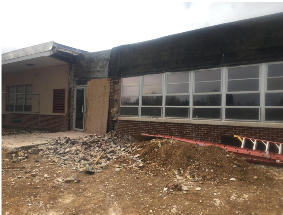
Sam area after overhang was removed and opening weatherproofed.
