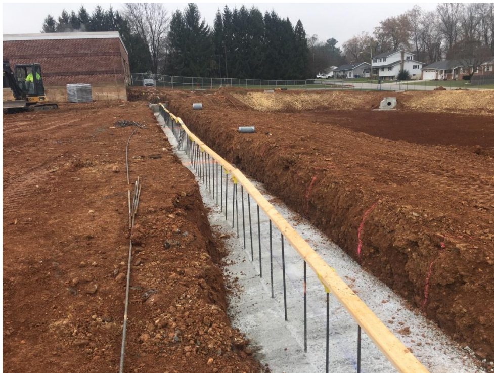
Footer for classroom addition on the Queen St side of building..
