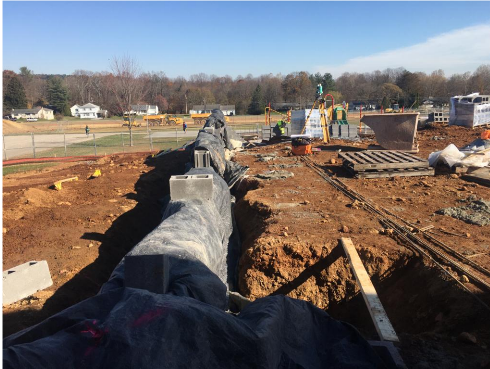
Footers and wall with cold weather protection installed.
