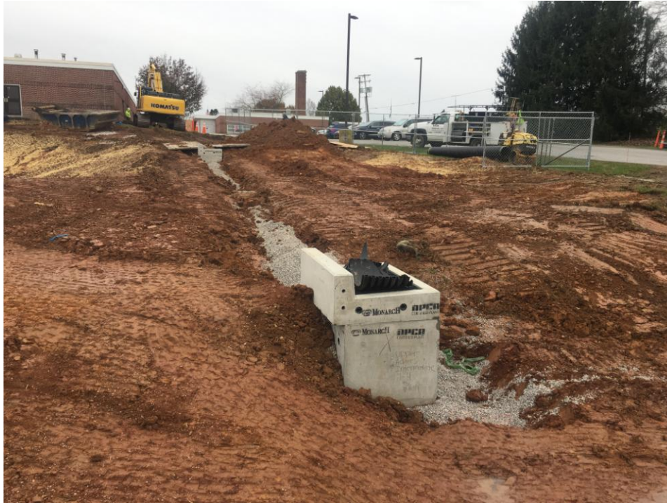
New outlet to existing retention pond for new storm basin at West side of building by rear parking lot.
