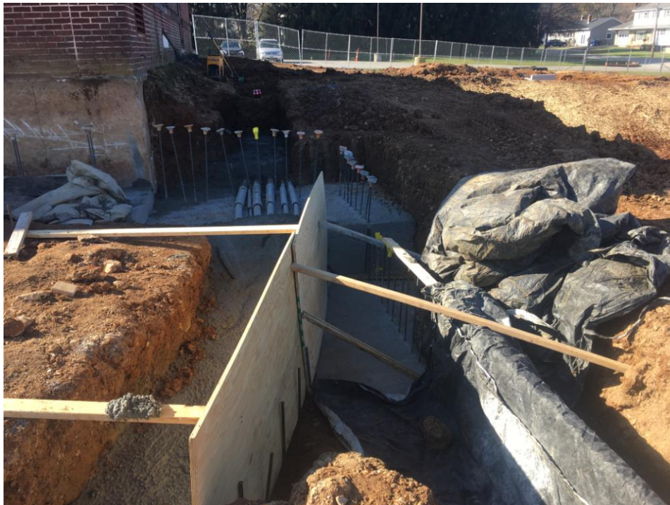
Trench for Classroom Addition duct bank where it crosses footer.
