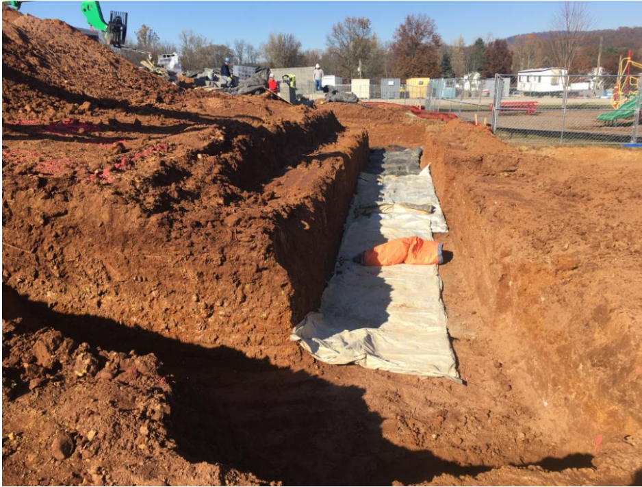
Footer trench being installed for East wall of Gym.
