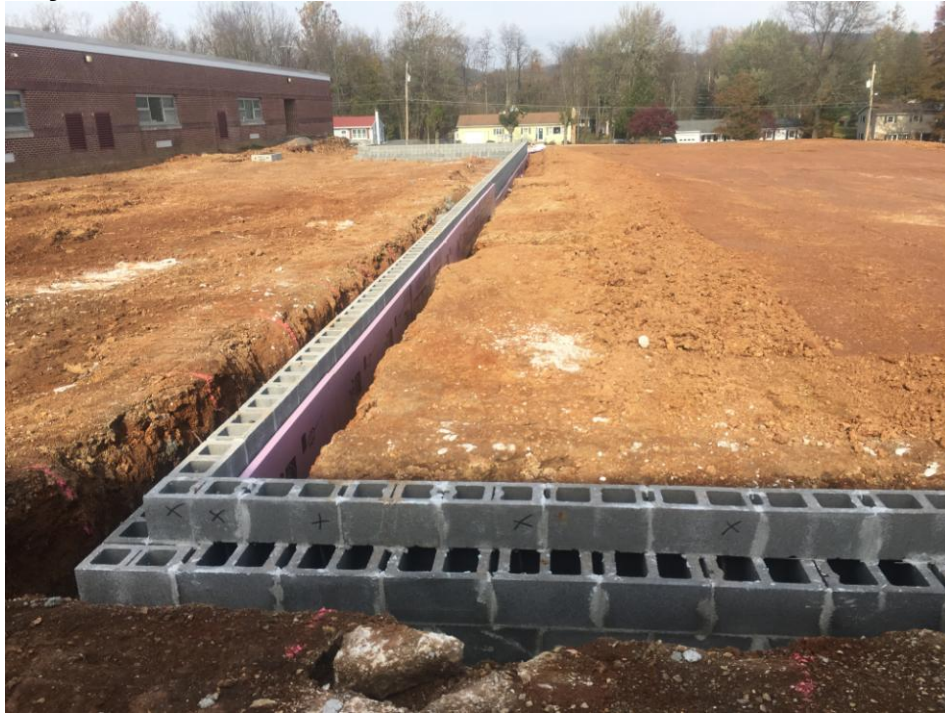
Foundation walls being installed.
