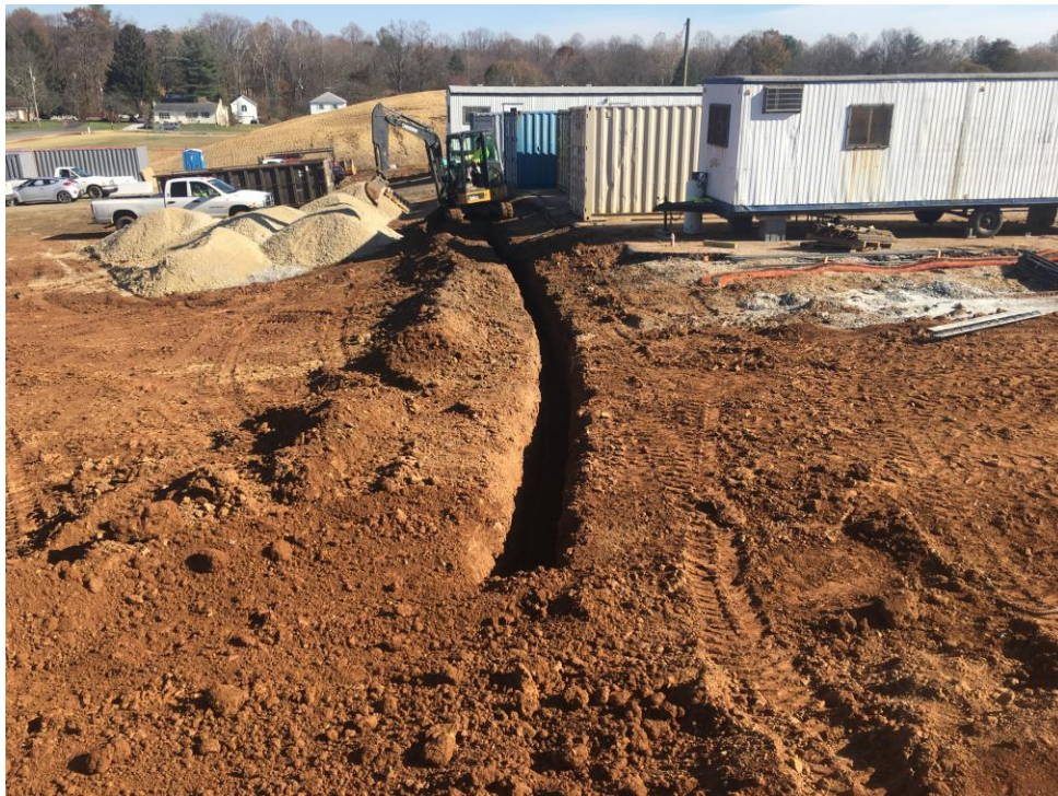
Trench for temporary electric cable for contactor trailers.
