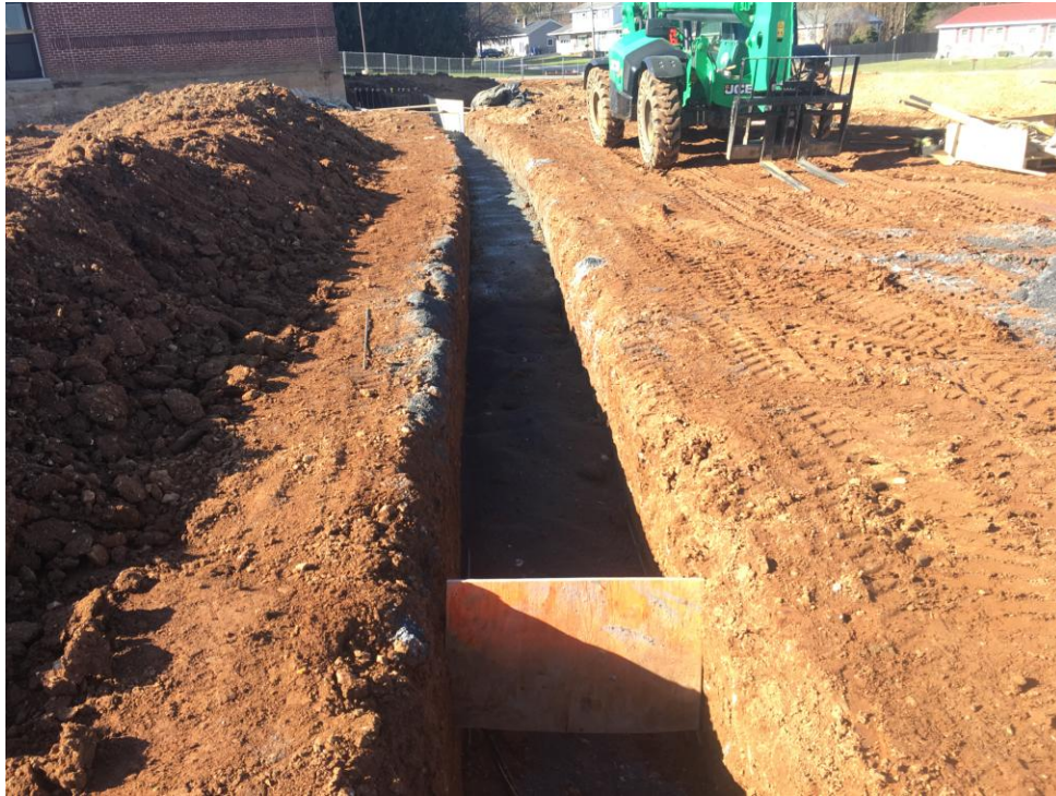
Duct bank being carried under classroom addition footer.
