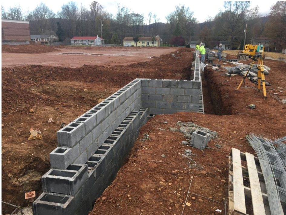
Foundation and building walls being installed.
