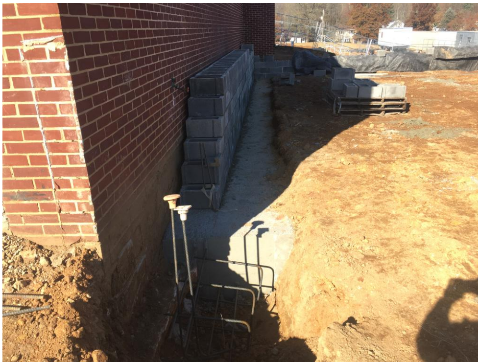
Start of foundation wall for Gym/Band Area.
