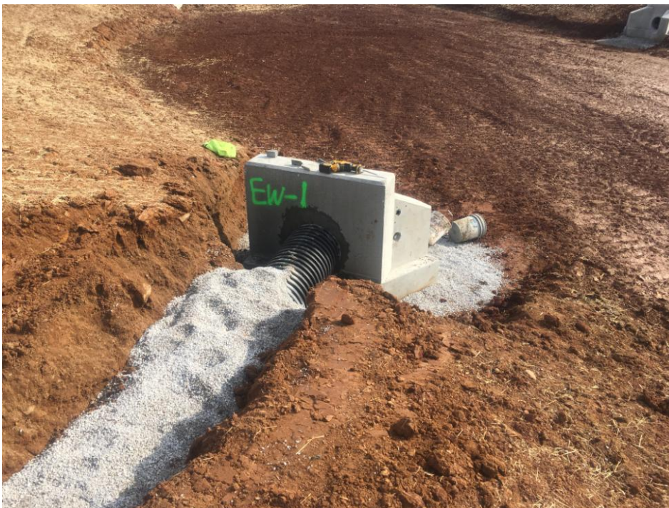
Outlet wall for new drain at East side of existing building classrooms.
