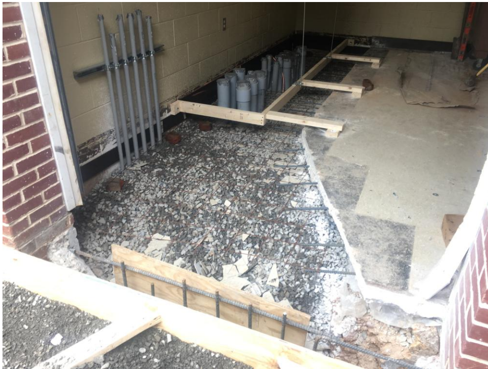
New switchgear area ready for concrete pour.
