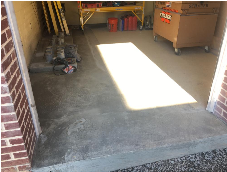
New switchgear area after floor was poured.
