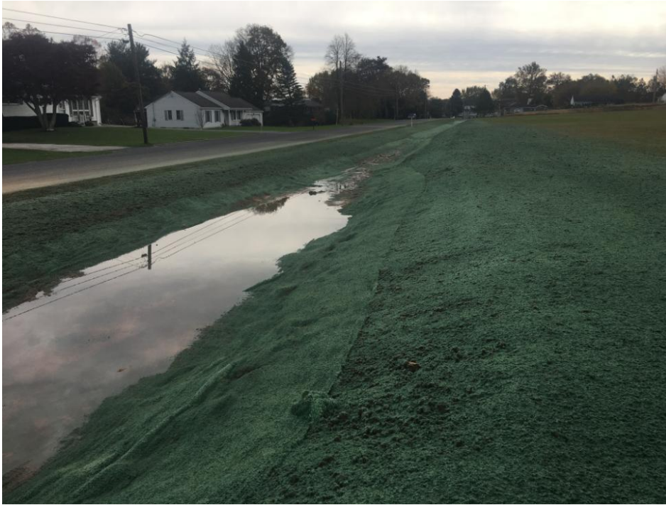
Stabilization matting and seeding along Conewago St.
