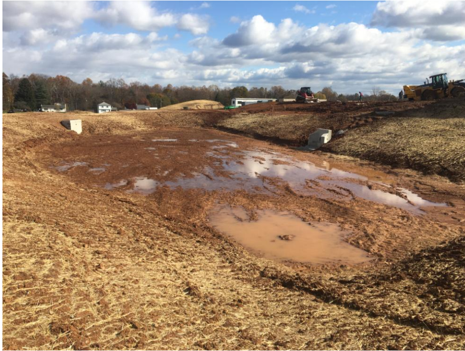
Detention Pond along Queen St showing new drain headwall on right.
