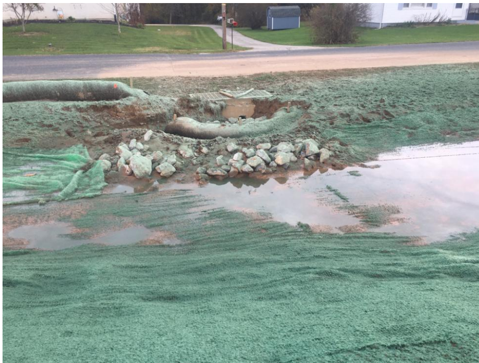
Stabilization matting and seeding at Conewago St drain.
