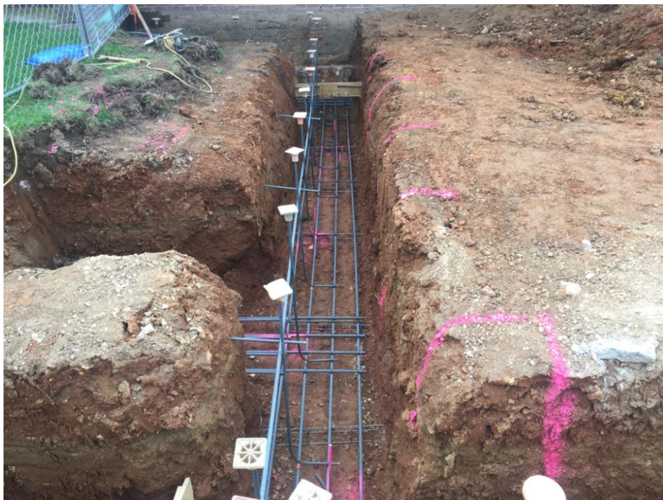
Rebar being installed in footer trench.
