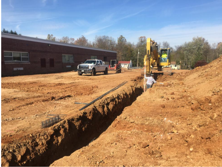
Footer trench being dug.
