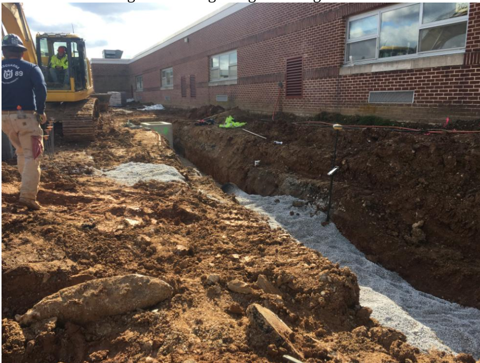
New catch basin and storm line being installed.
