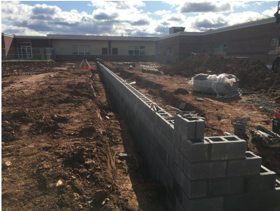
Foundation wall being laid.
