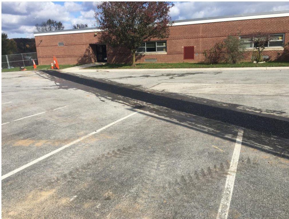
Trench for electrical duct bank has been paved across rear parking lot.
