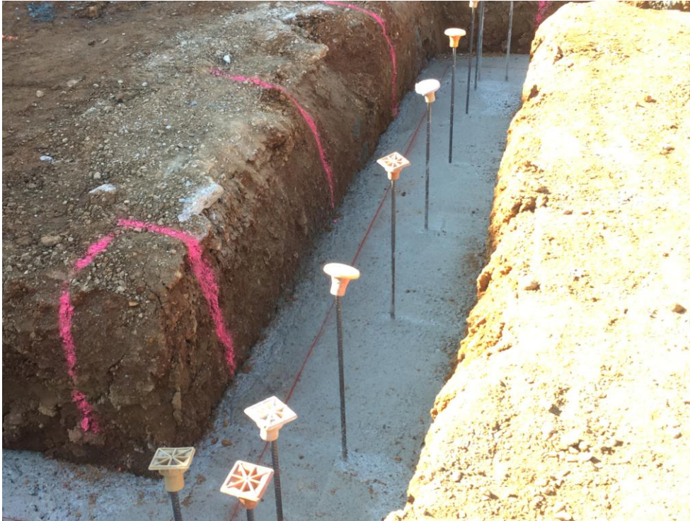
Footers after pouring.
