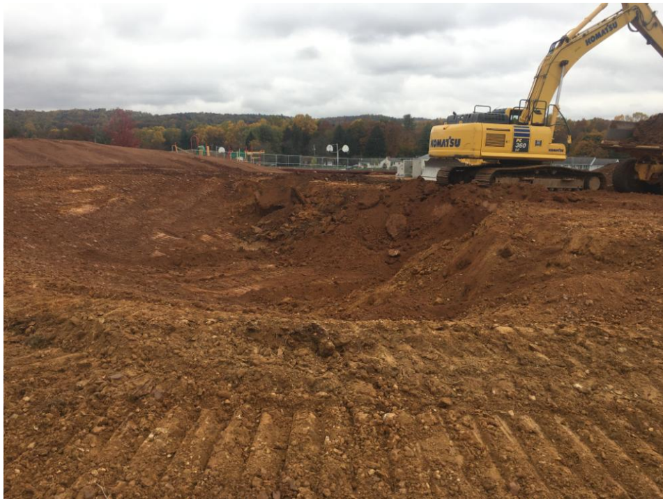
Excavation of the upper Detention Pond along Fohl St.
