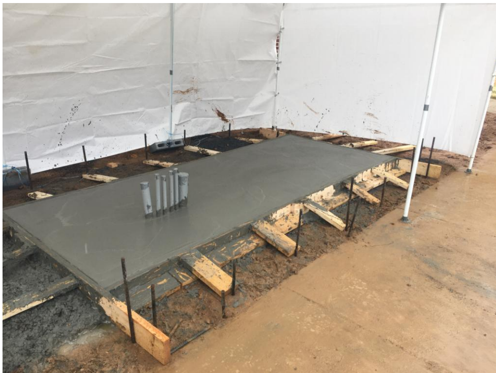
Pad for new Generator.
