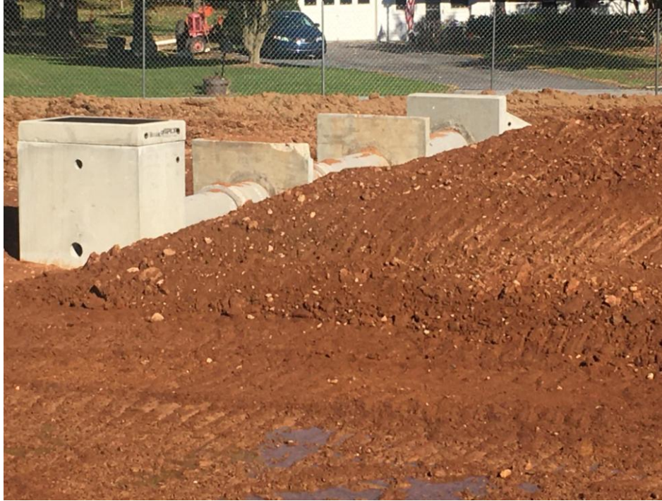
Installation of pond outlet and storm piping on Queen St side.
