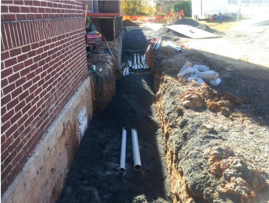
Duct Bank being installed at side of building and into switchgear.
