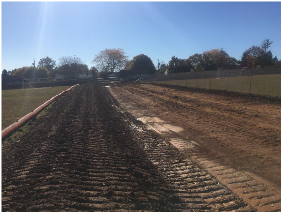
Temporary Haul Road across site with E&S sock installed.
