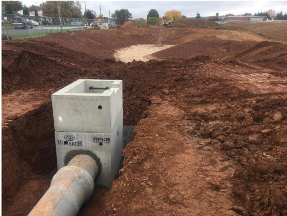
New Detention Pond and outlet structure along Fohl St.
