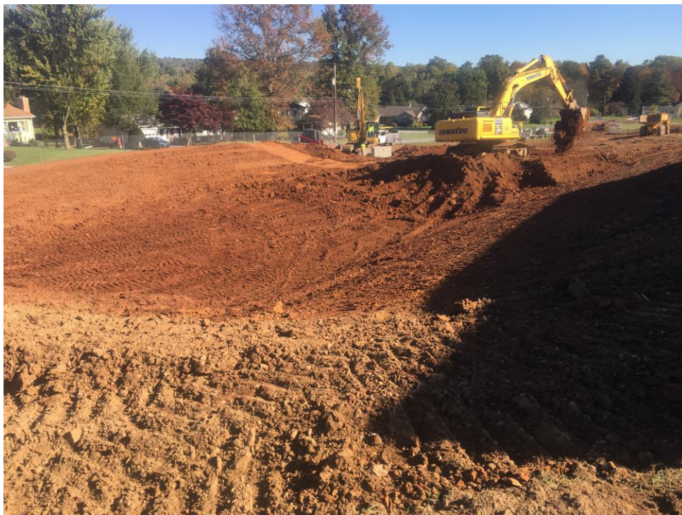
New Detention Pond.
