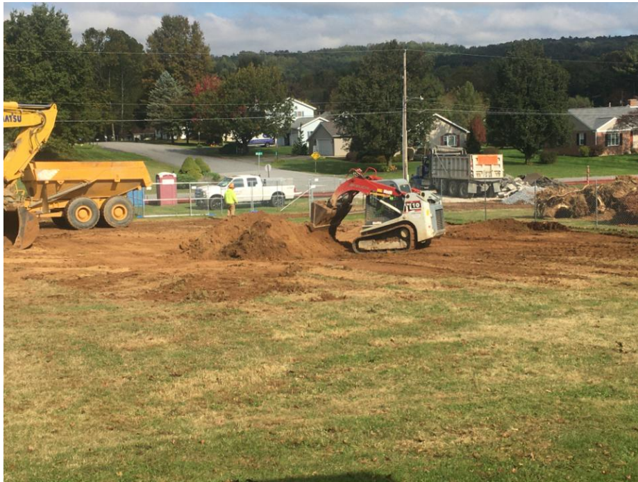
Topsoil being stripped from site..
