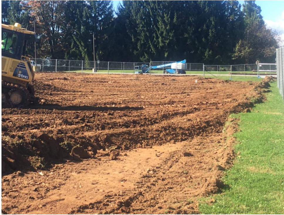
Beginning excavation for new detention pond.
