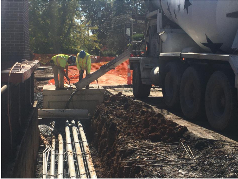
View of concrete being poured over new electric duct bank from vault.
