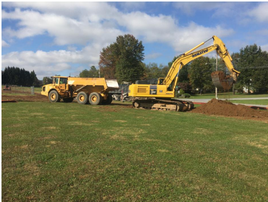
Excavation for storm drainage starting.
