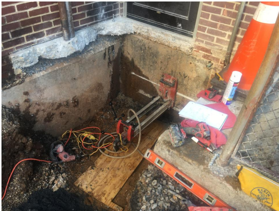
Core drilling for conduits into basement electrical room..
