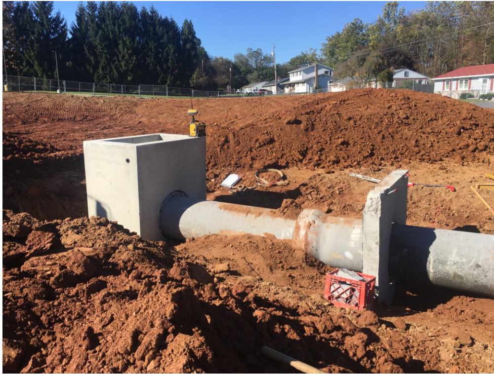
Detention pond outlet and storm water piping being installed.
