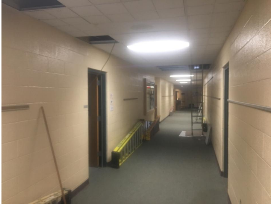
View of main hallway at BES with almost complete ceiling tile installation.
