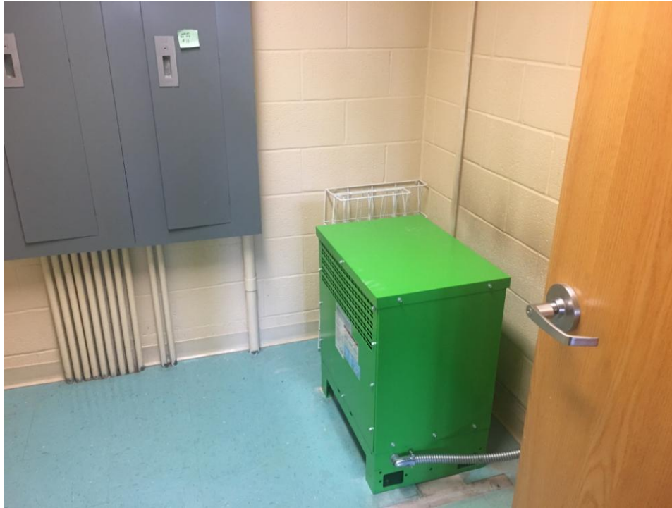
View of new transformer being installed in the corridor closet at BES.
