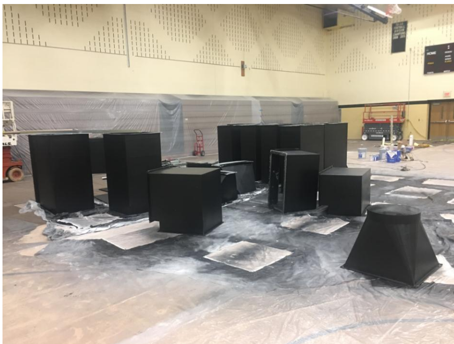
New ductwork being painted in Gym at BHS
