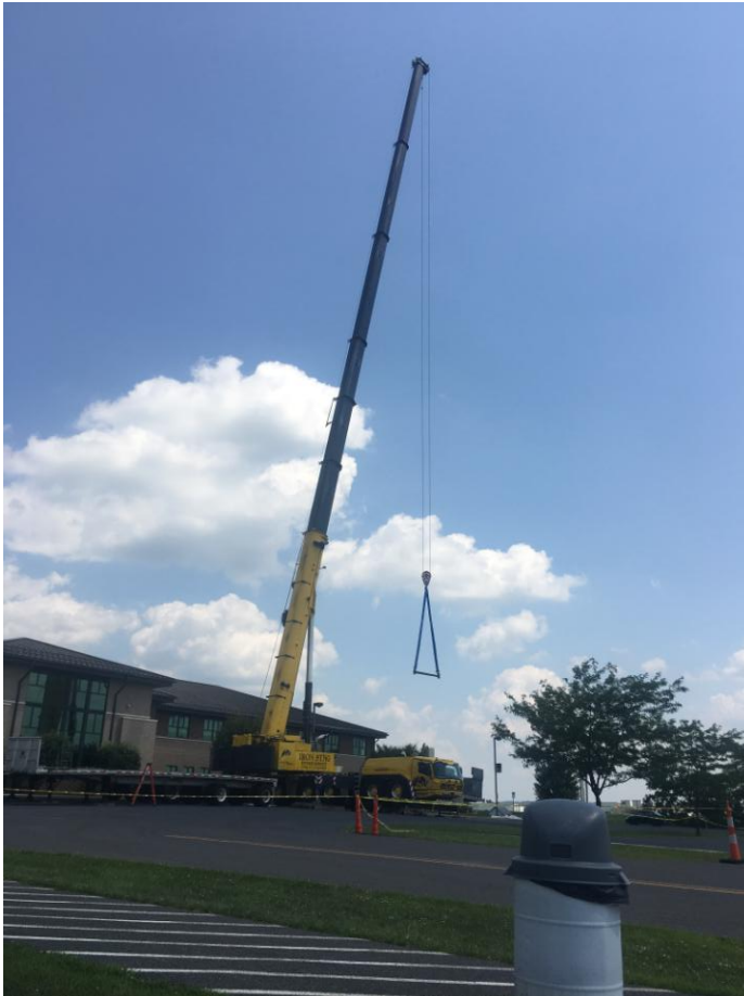
Crane getting ready to lift units at BHS.
