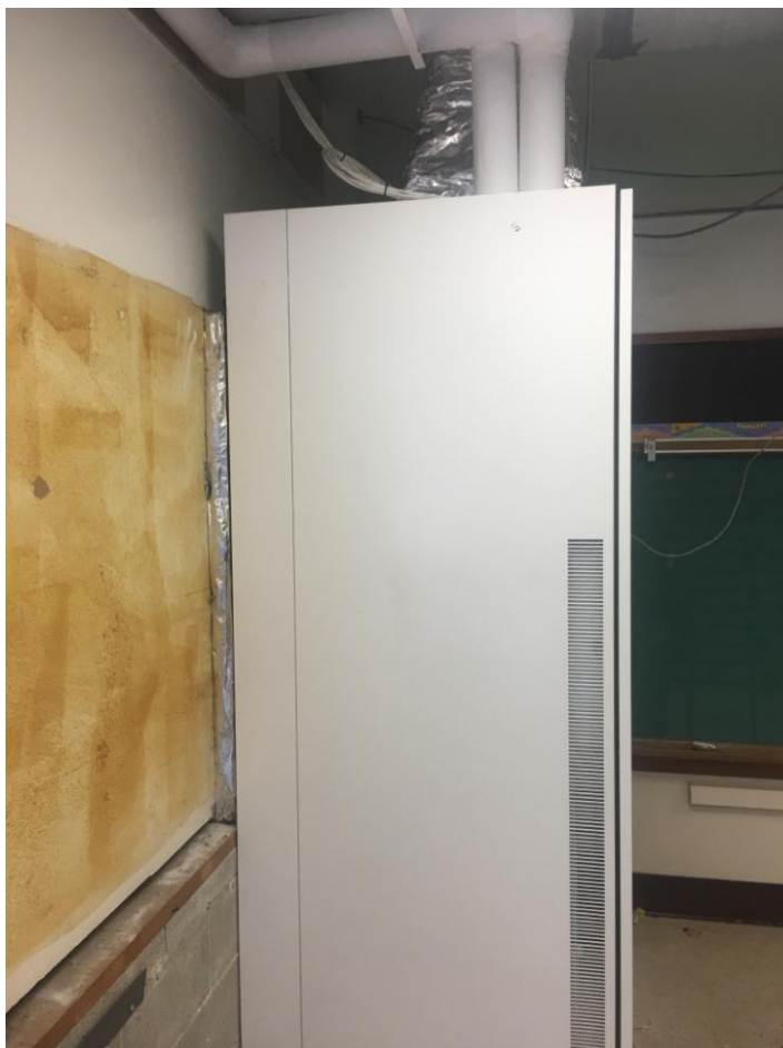
VUV unit being installed in short hall classroom at AES .
