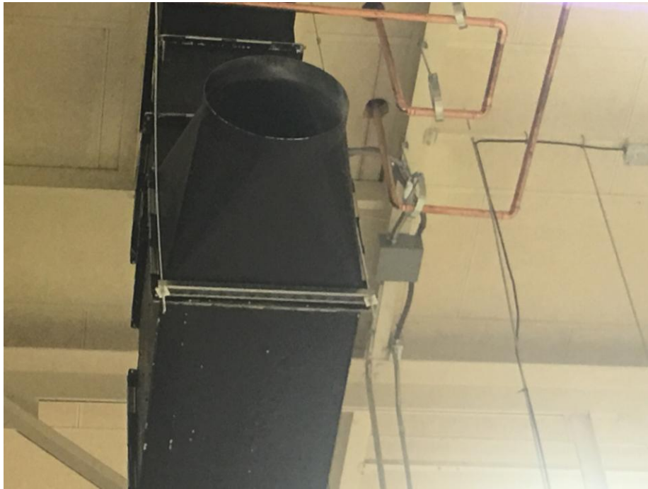
New duct takeoff in BHS Gym.
