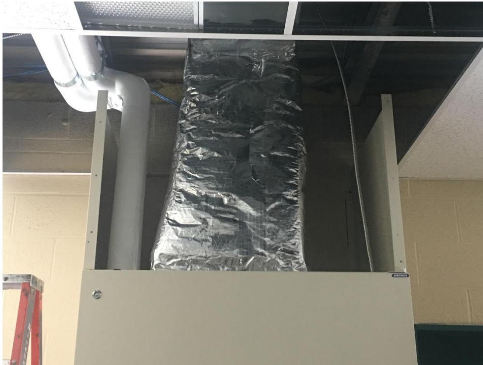
View of ductwork and cover installation on classroom VUV at BES.
