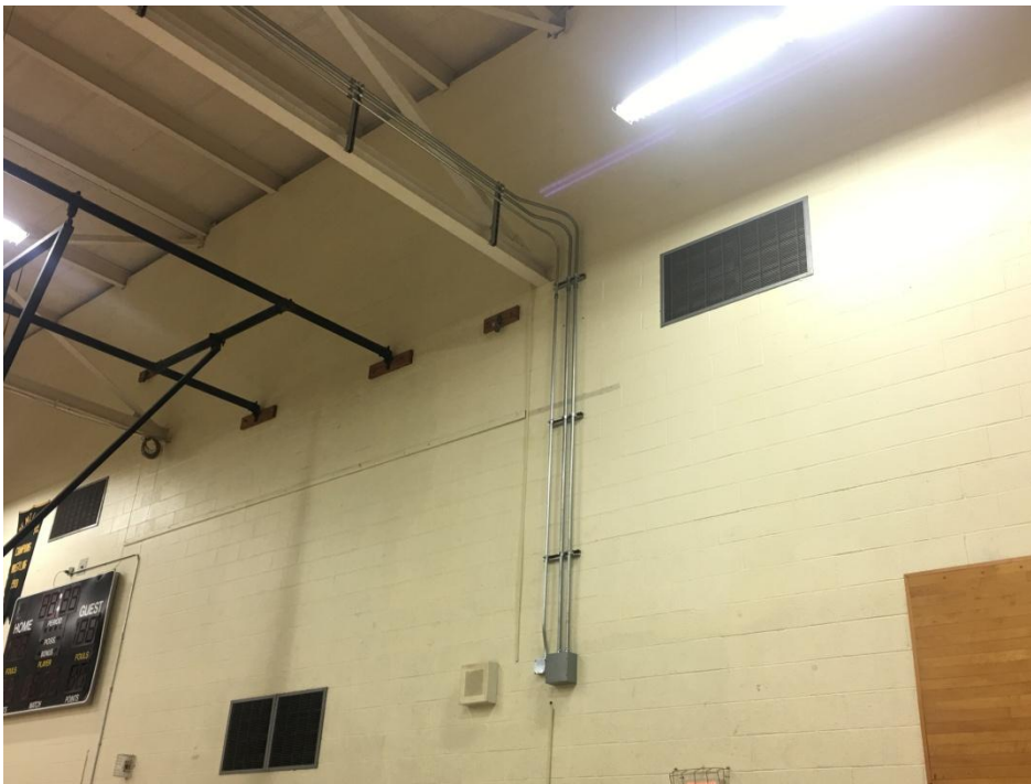
View of new electrical piping at BHS.
