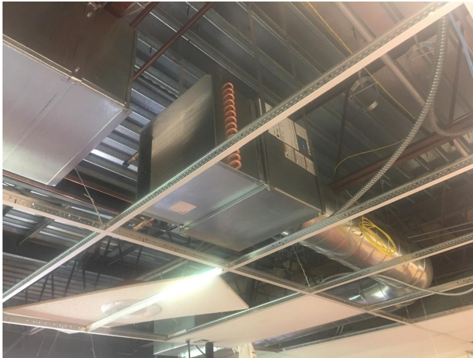
View of VAV unit coil being installed.
