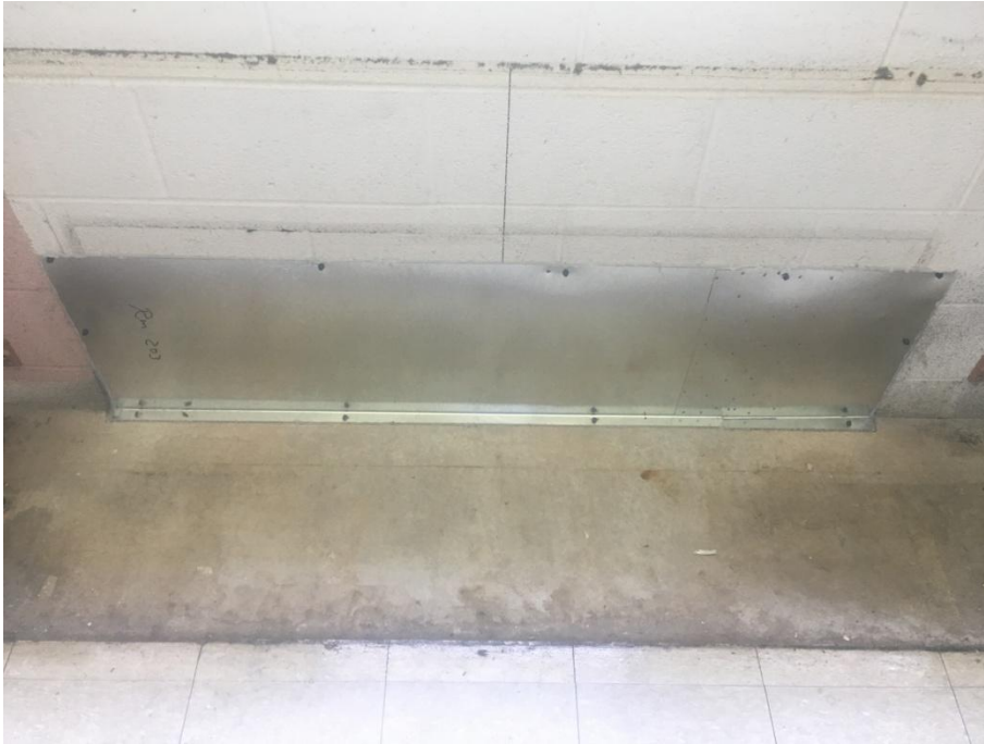
View of closure panel of old vents at AES. This will be behind the new shelving.
