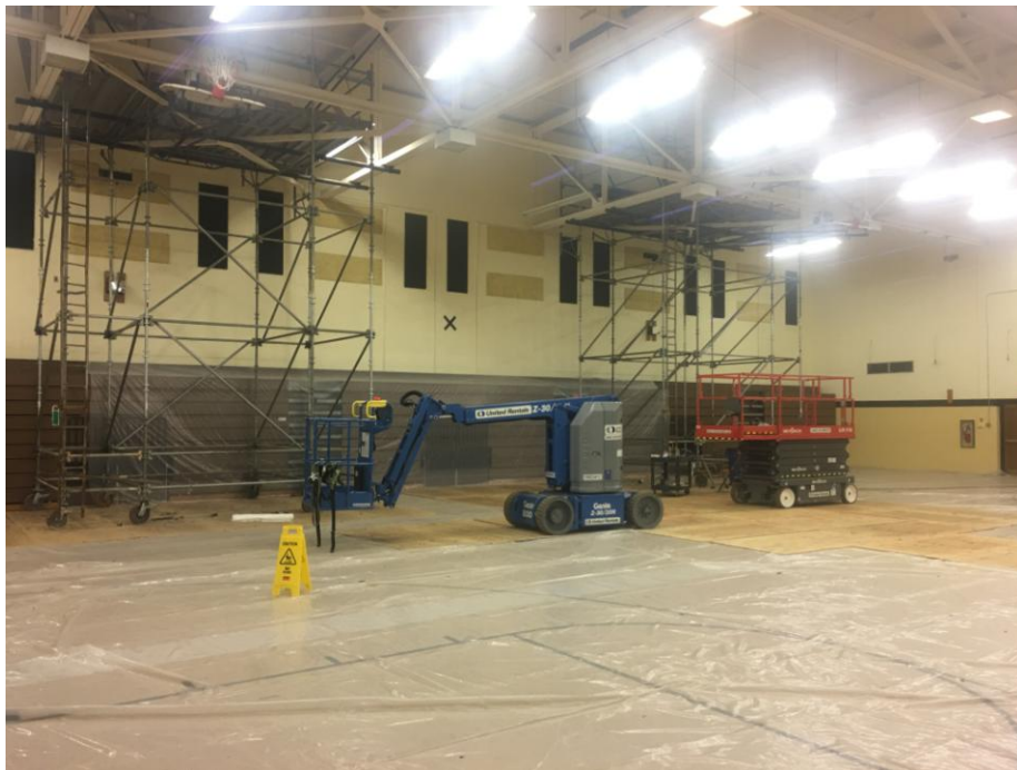
View of work being done in North Gym of BHS.
