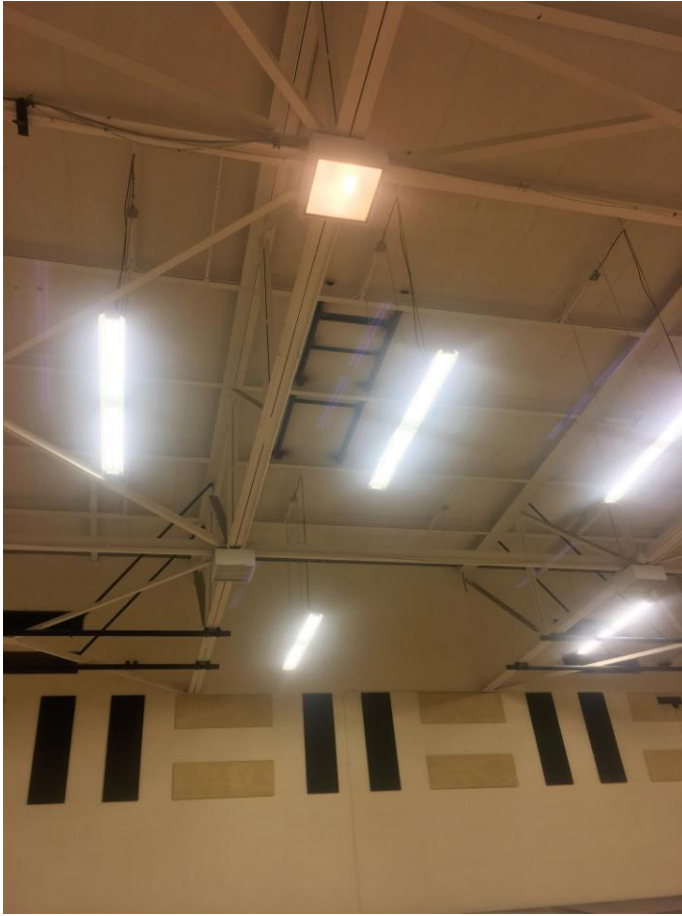
View of steel supports for new units in North Gym at BHS.
