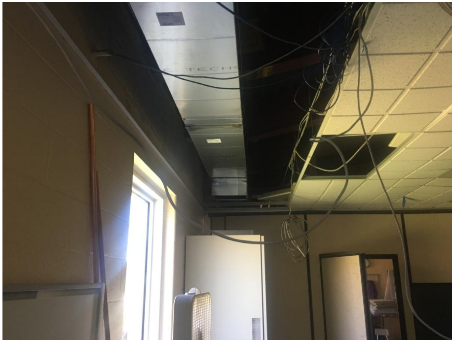
View of ductwork being run to new VUV unit.
