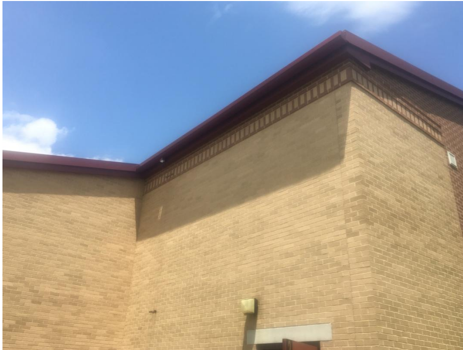
View of new gutter at BES..
