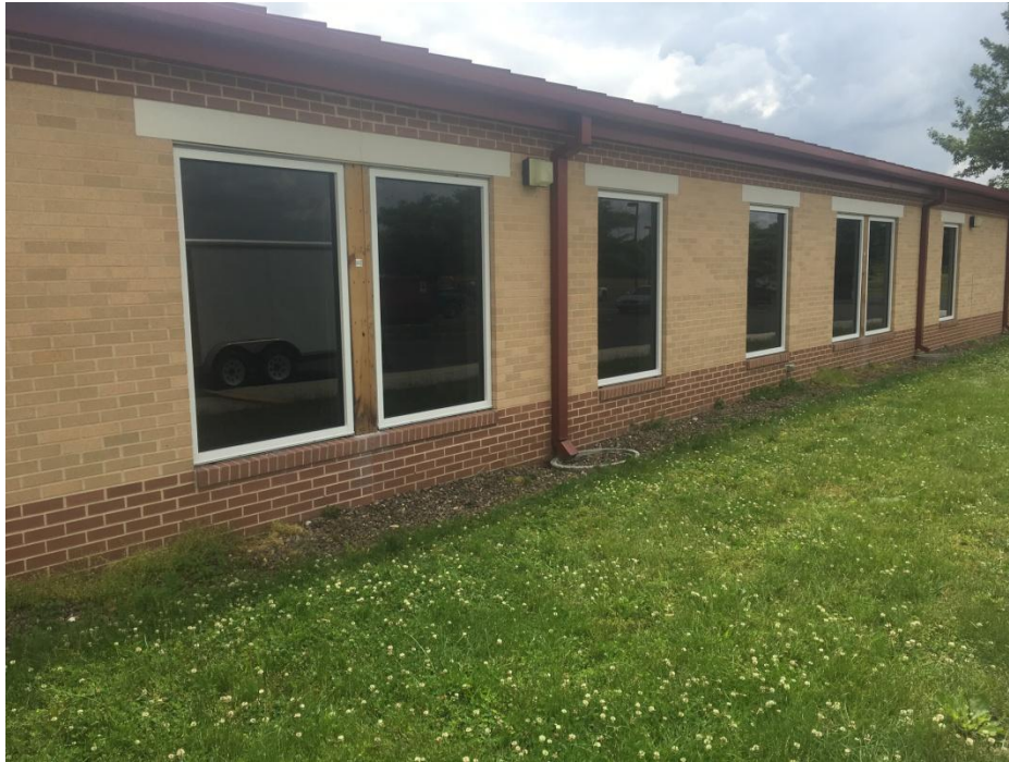
View of new windows at BES.
