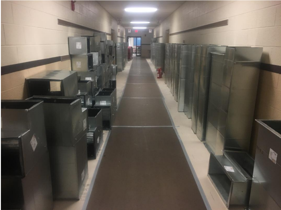
Ductwork ready to be installed at AES.
