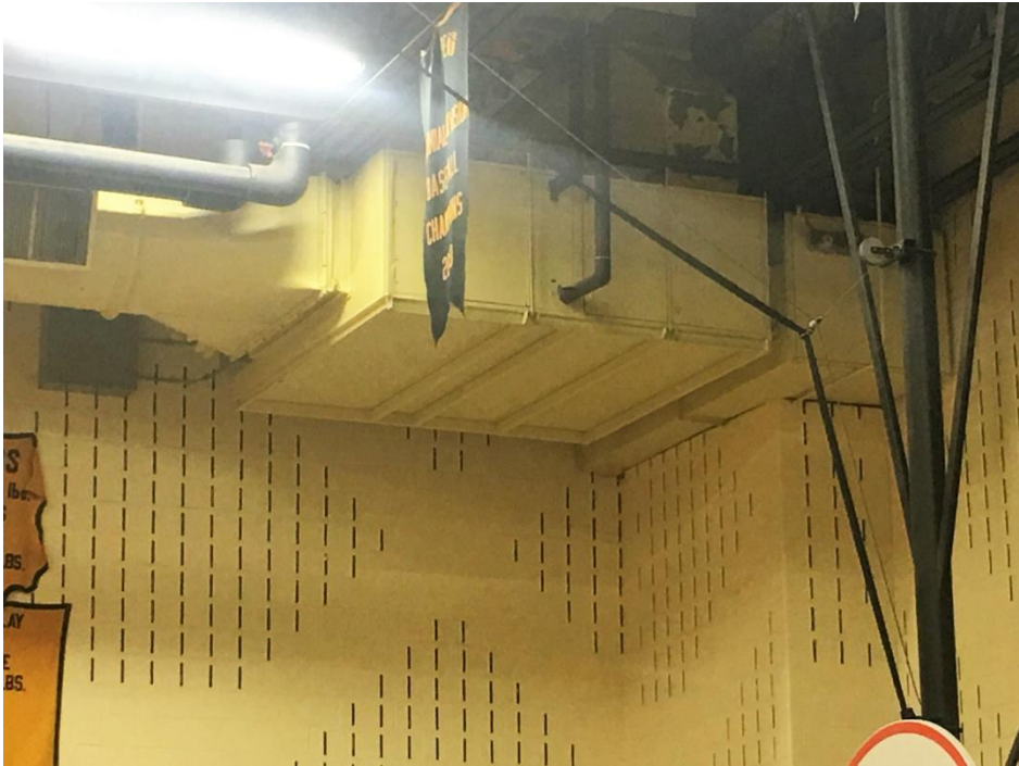
View of one of the units being removed at BHS.
