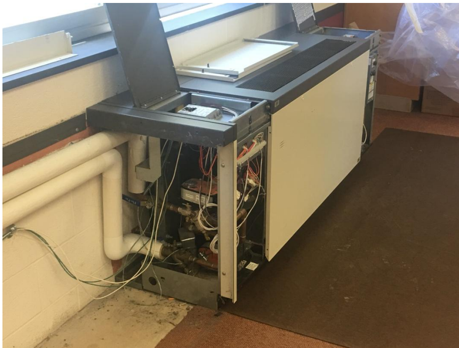
Unit Ventilator being demoted at AES.
