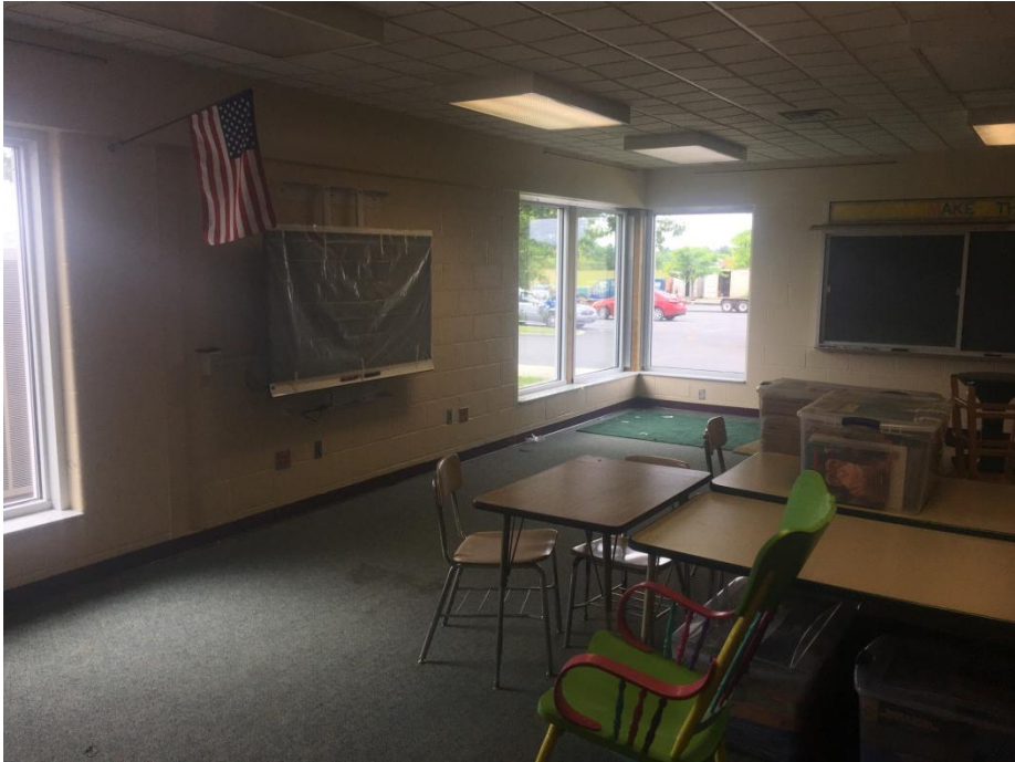
Interior view of new windows at BES.
