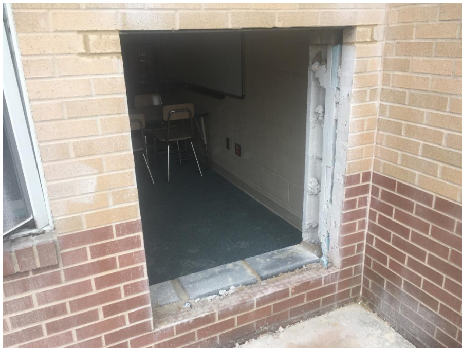
Close-up of masonry opening for new HVAC unit at BES.
