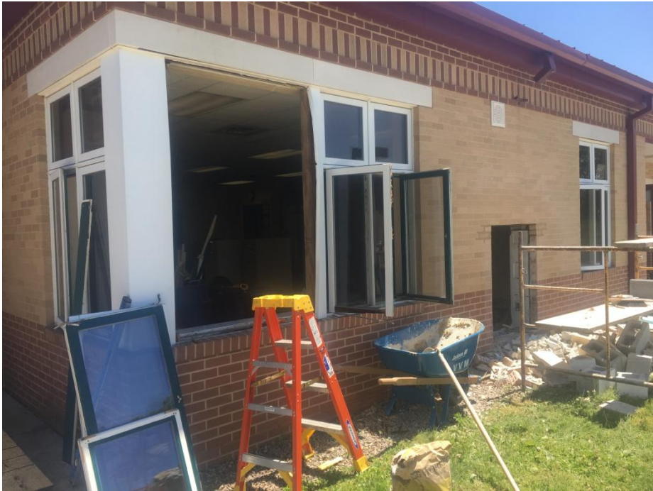
View of window demo and masonry opening installation at BES.
