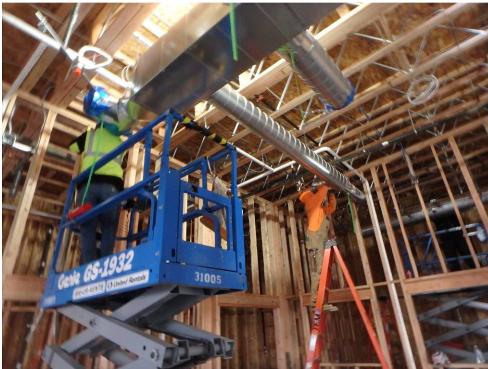
Vacuum lines above the dog wash stations
