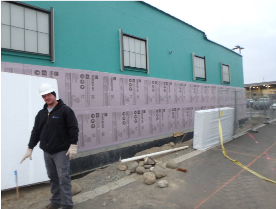
North elevation insulation and translucent windows
