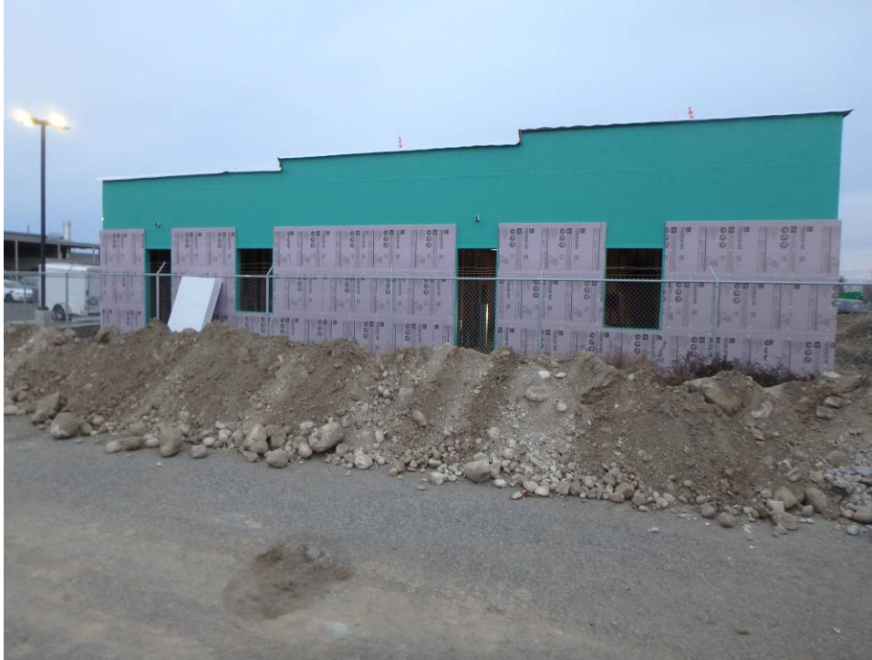
South elevation insulation board and liquid-applied
