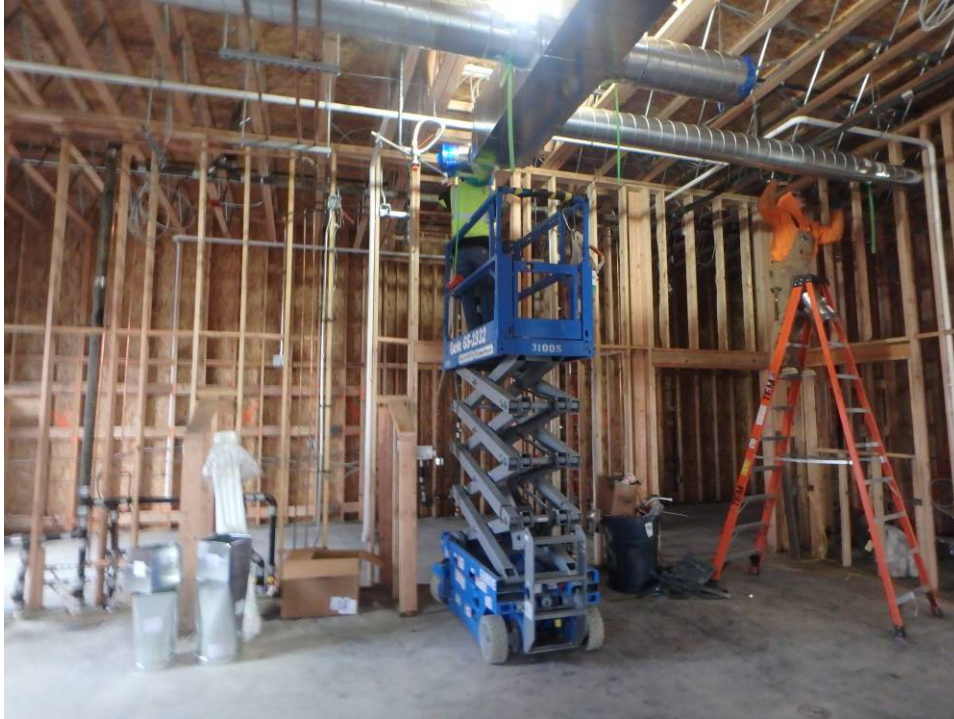
West wall of the lab, framing and ductwork
