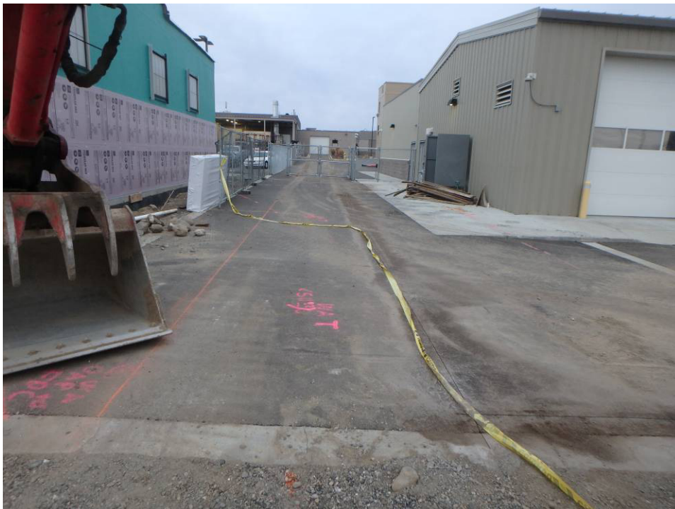
Looking west at the saw cuts to the northwest fire hydrant between the buildings.
