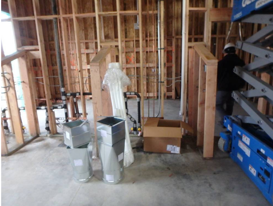
Vacuum lines (white) behind the dog wash stations
