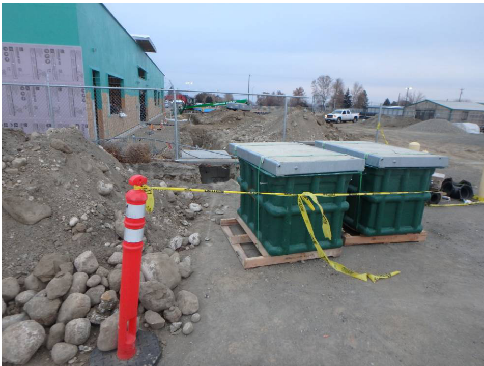
Two of the three Fiber vaults
