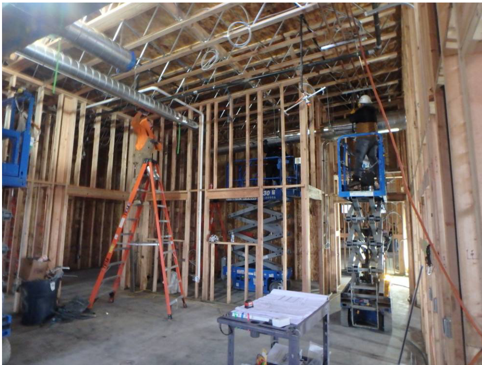
Office framing and ductwork
