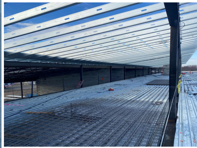
L3 Mezz Decking & housekeeping Pad
