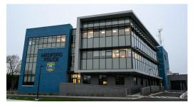
The new Medford Police Station opened in December 2020. On its roof is a 60 kW solar system, fully owned by the city, which helps power the station. The building itself is highly energy-efficient and uses half the energy that it would consume if it was built to only meet the current energy code. The station uses zero fossil fuels for its heating, cooling, and ventilation systems, and instead, relies on heat pumps and a highly efficient energy recovery ventilation system.
