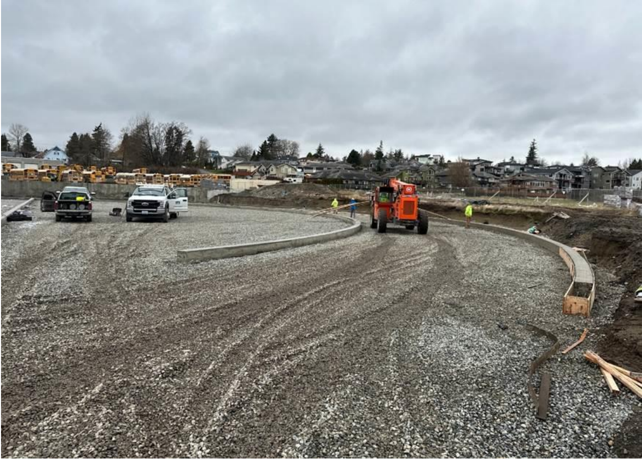
Track curb ongoing installation
