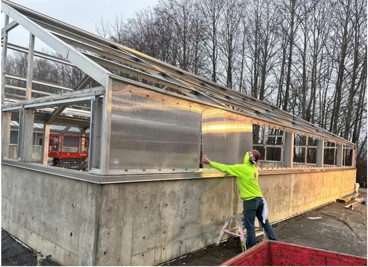
Greenhouse plexiglass panel installation is now underway
