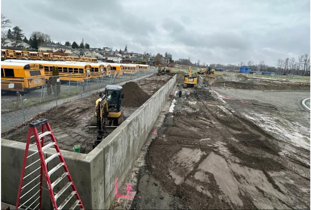
Backfill at the retaining wall next to the long jump area
