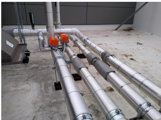
Figure 6. Chilled Water Hydronic Piping
