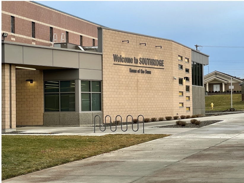
Figure 13. Weight Room Addition
