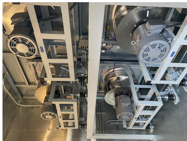
Figure 9. RTU Factory Start-Up
