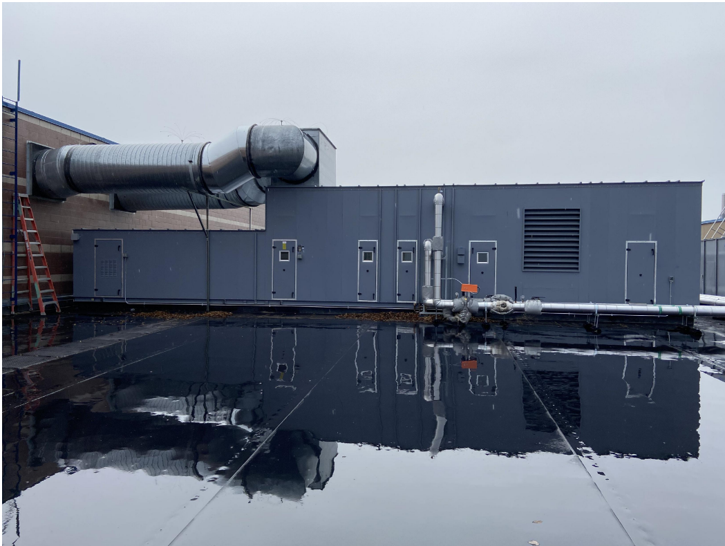
Figure 8. Energy Recovery RTU
