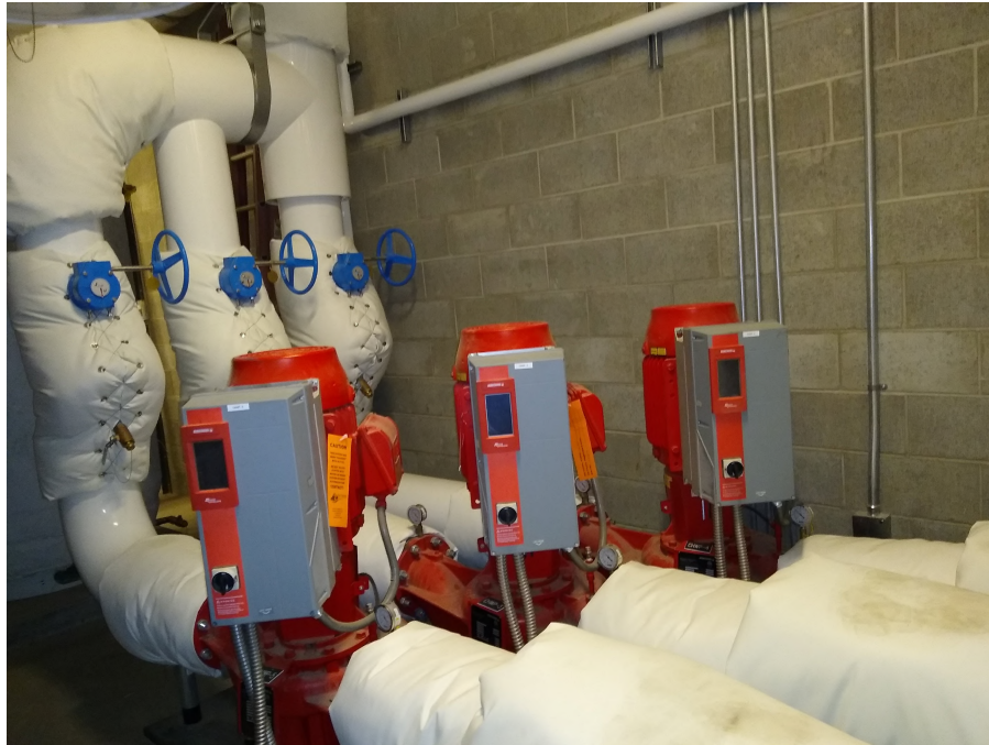
Figure 12. Chilled Water Pumps
