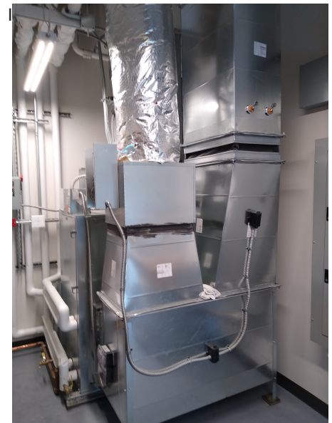
Figure 11. Fan Coil Units
