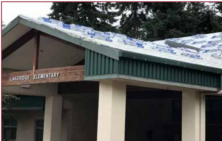
Infrastructure projects such as the new roof at Lakeridge Elementary are funded by the capital/tech levy.
