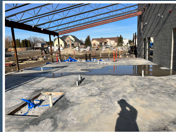
Kitchen Rough-in & Steel Framing
