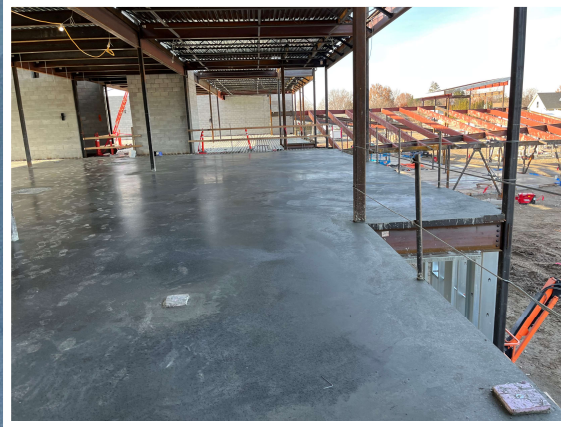
Area B Slab on Deck
