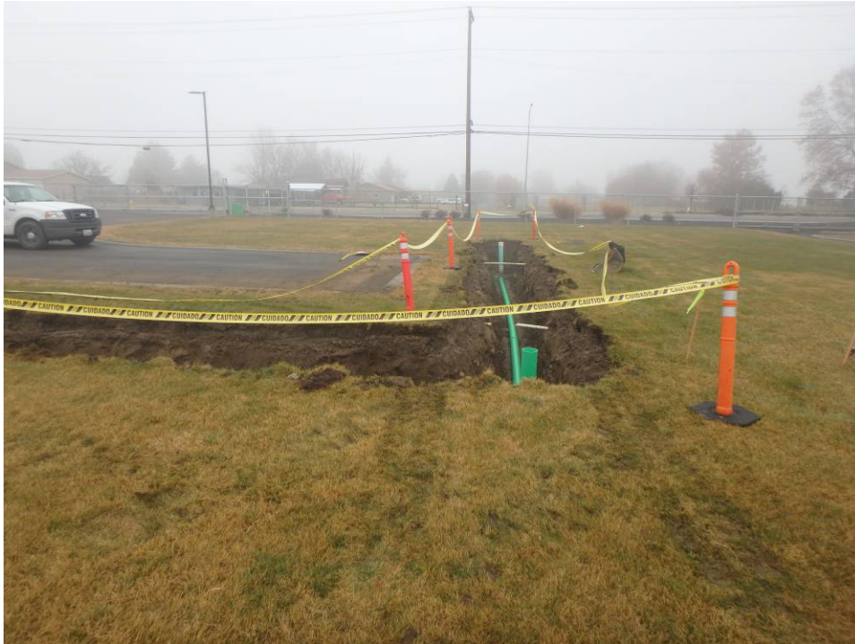
Sewer line set looking north
