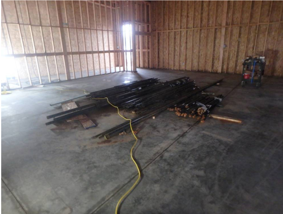
North classroom and staged sprinkler piping
