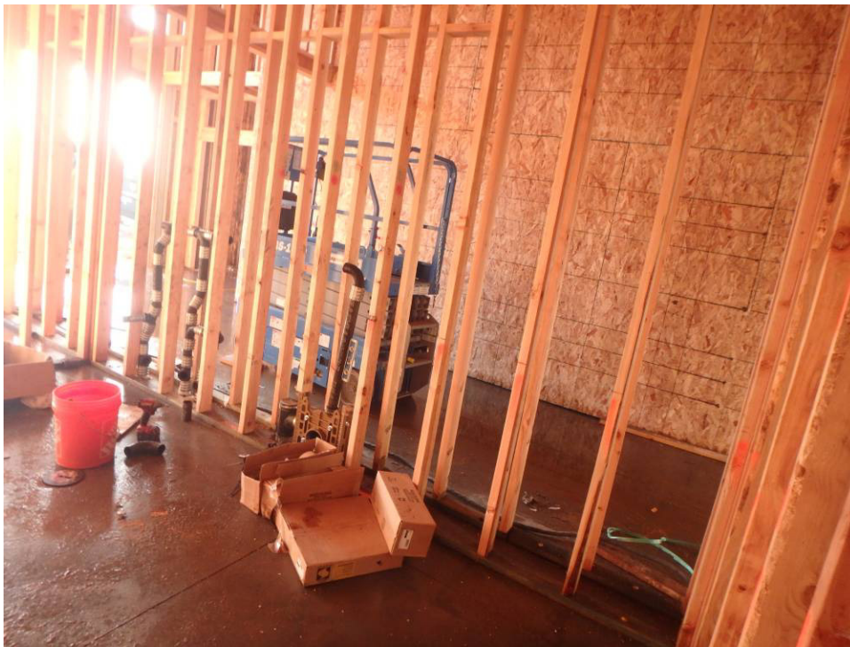
South Restroom rough-in and framing
