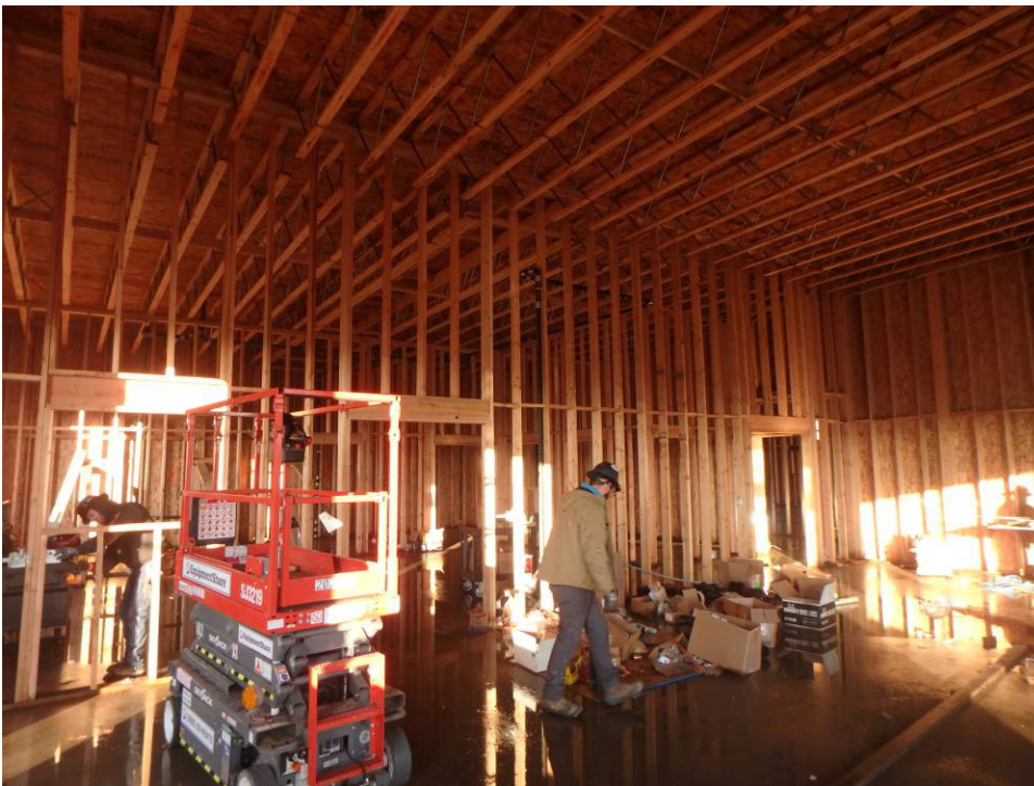
Looking north at the classroom (southeast room) framing, sheathing and roof framing
