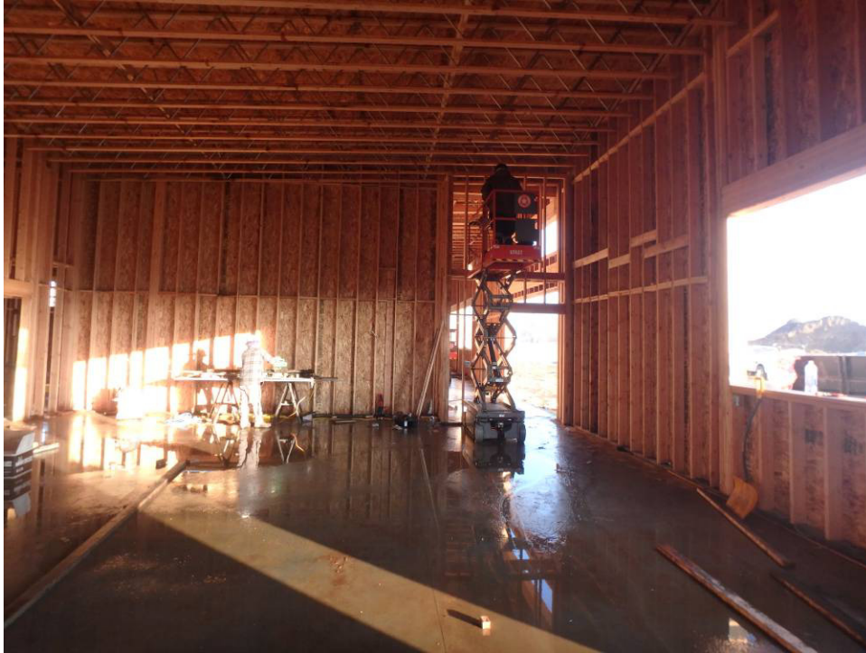
Looking north at the classroom entrance framing, sheathing and roof trusses
