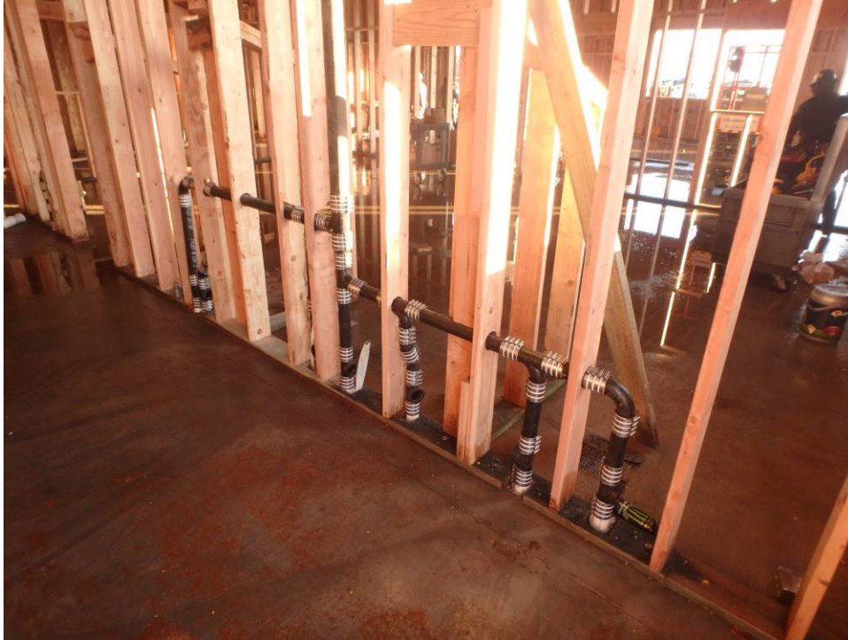
Plumbing stub-ups for the dog washes from the kennel side
