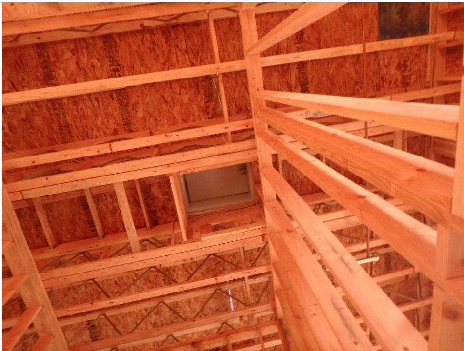
Roof hatch and roof trusses
