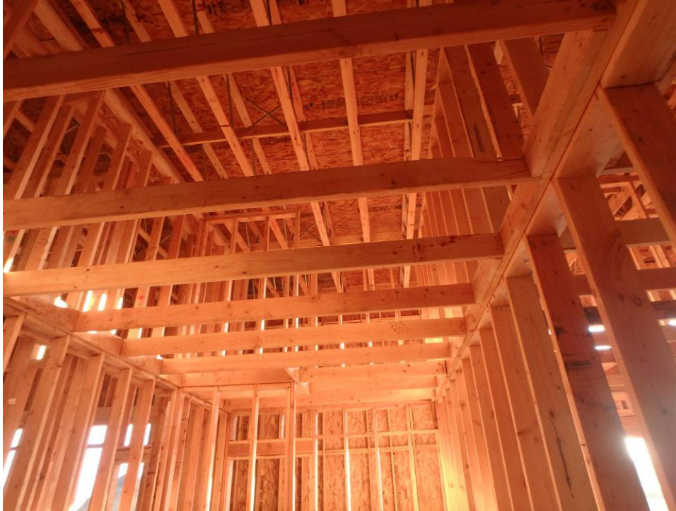
Restroom dropped ceiling framing
