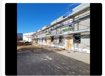
Stucco on the southern classroom
